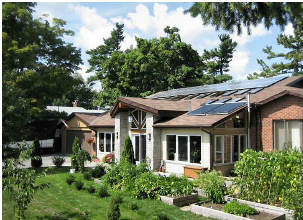
Figure 4. The “testbed” system. The store is buried under the lawn (six boreholes, 20 m deep). The air-heat collector is behind the bushes on the right. The heat pump is in the basement. A pair of solar collectors is mounted on the roof (lower right).
