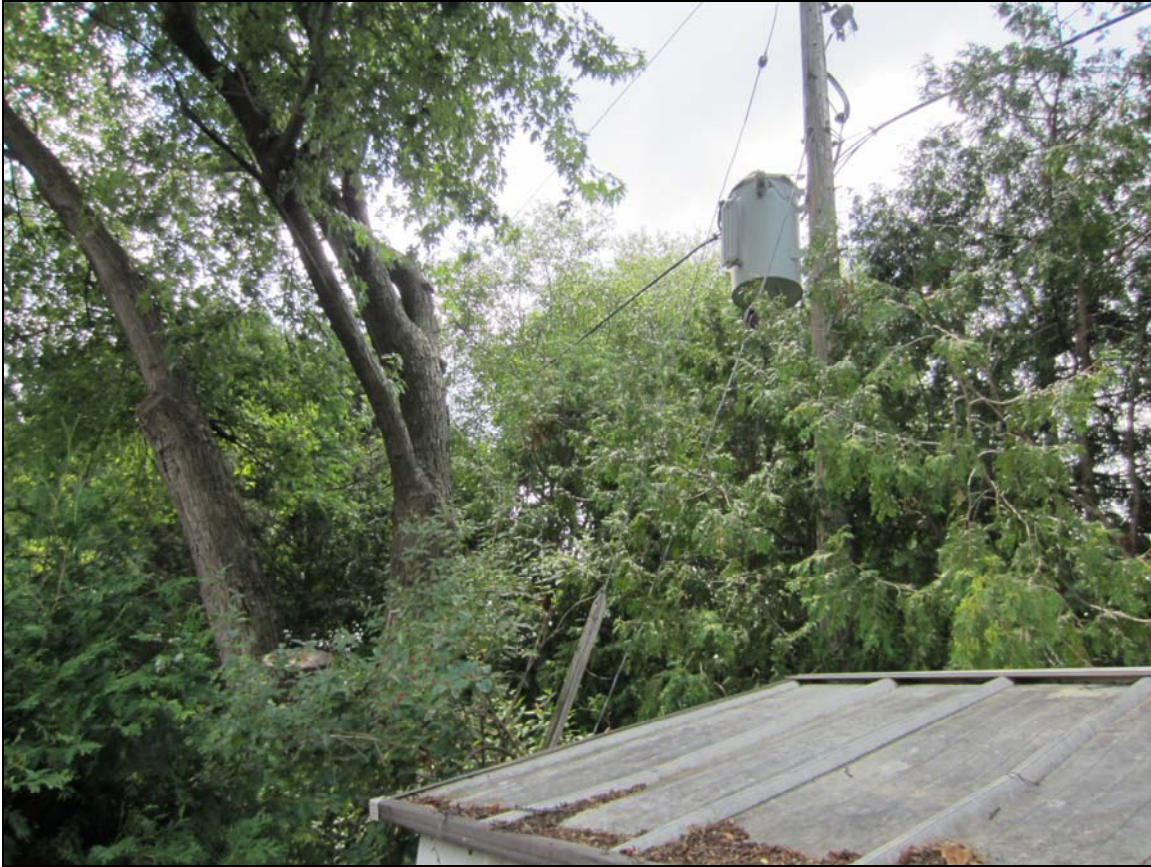
Figure 12. Pole and transformer surrounded by vegetation
