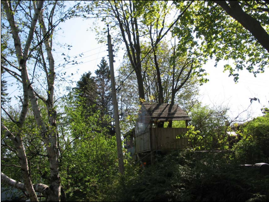
Figure 11. Pole obstruction caused by customer construction
