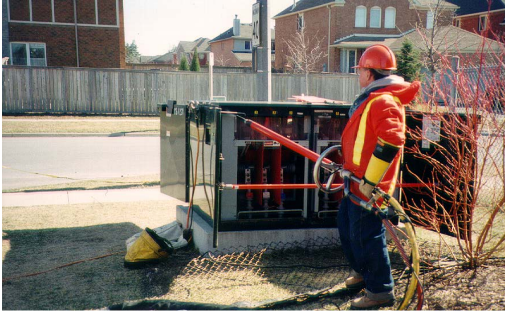
Figure 56. 27.6 kV Switchgear Dry Ice Cleaning
