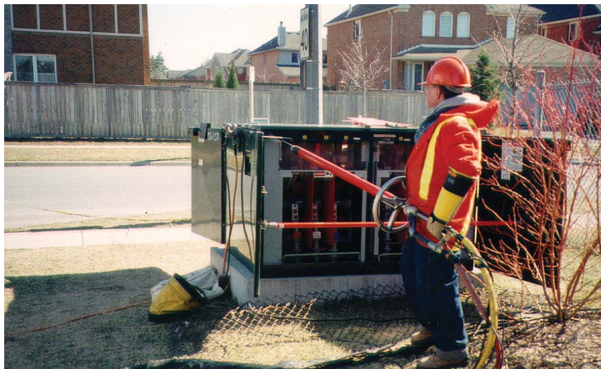
Figure 10.4.1.1: 27.6 kV Switchgear Dry Ice Cleaning
