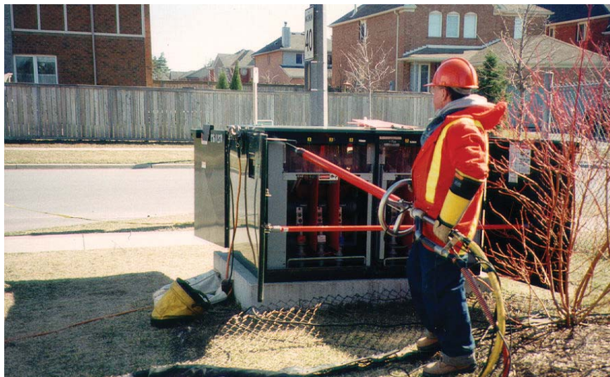
Figure 10.4.1.1: 27.6 kV Switchgear Dry Ice Cleaning
