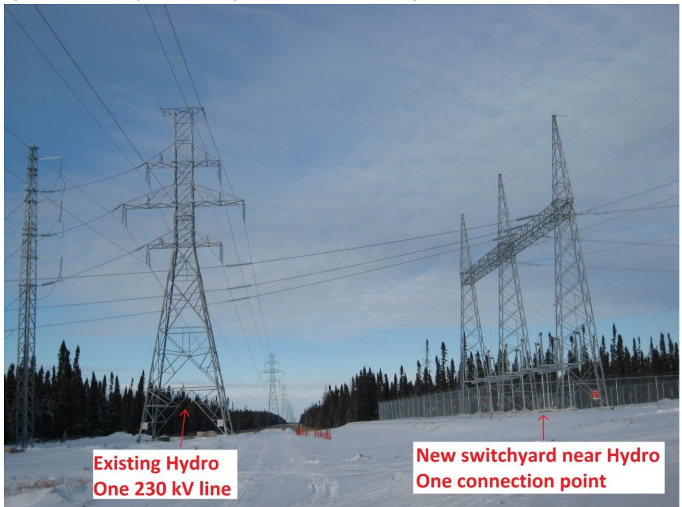
Figure 3: New switch yard near the Hydro One 230 kV connection point.
