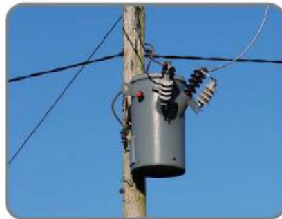
Pole Mounted Transformer
