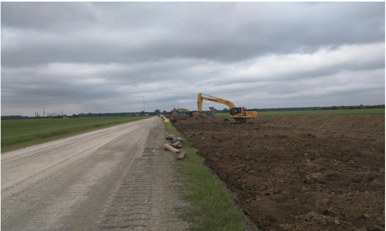
Following the preparation of the subsoil, the topsoil is replaced, disced and returned to, in this case an agricultural field.
