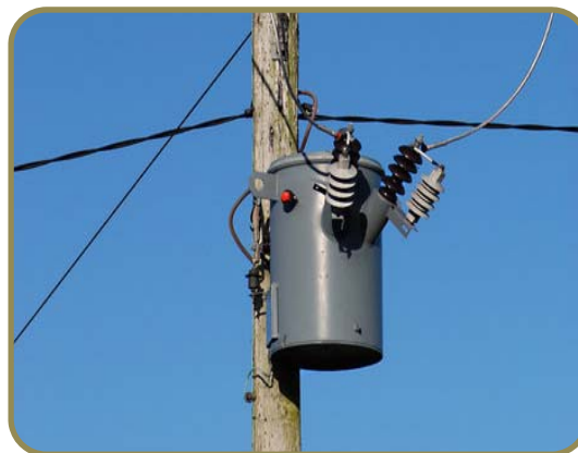
Pole Mounted Transformer
