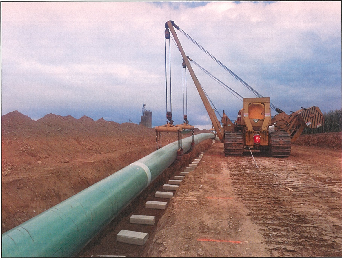
Foam pillows were installed at the bottom of the trench the entire length of the pipeline to protect the pipe from possible damage from stones.
