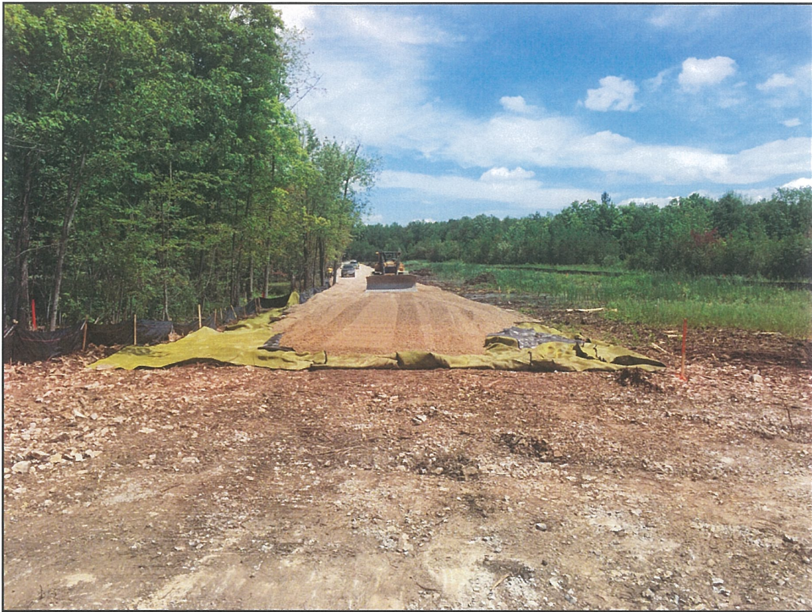
A temporary access road was installed through the wetland west of Valens Road (Beverly Swamp) to minimize impacts to the area from construction equipment. Wildlife exclusion fencing was also installed on either side of the right-of-way to ensure the protection of potential Eastern Milksnakes and other vulnerable species.
