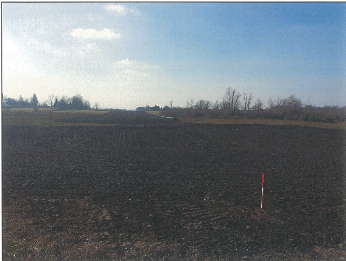
Topsoil soil was spread and returned back to original grade at the end of 2015. Union will perform additional cleanup along the right-of-way as required in spring 2016.
