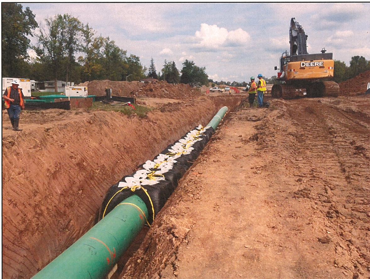
In sections of the right-of-way where the water table is higher, geotextile pipeline weights (PipeSaks) are installed to prevent the pipe from floating to the surface.
