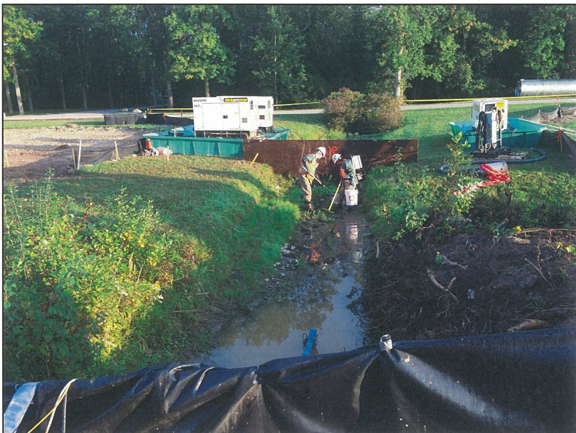
A fish/wildlife rescue is conducted by qualified biologists once the area is isolated. Digging cannot begin until all fish/wildlife are relocated downstream of the crossing location.
