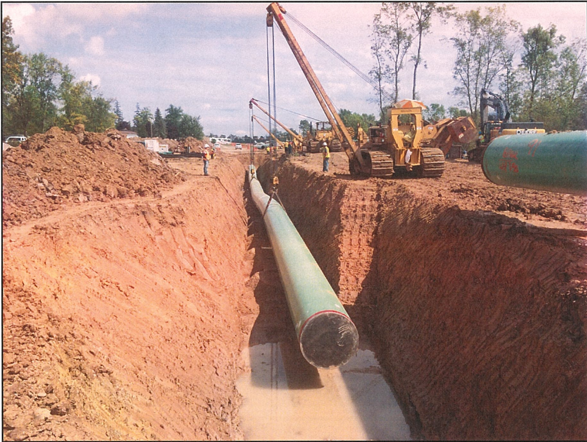
A shorter “creek section” of pipe is lowered in during watercourse crossings to help ensure watercourse crossings are completed within 24 hours.
