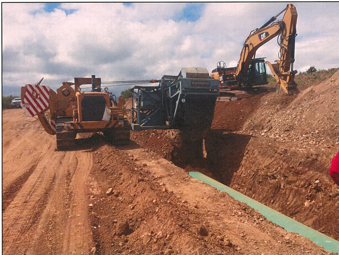
Subsoil is screened during initial backfilling operations using a padding machine to ensure stones do not damage the pipe.
