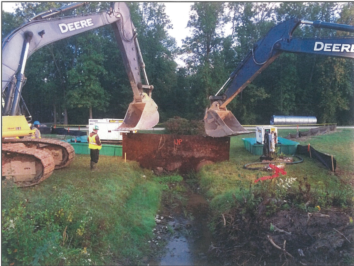
Steel plate dams are installed in watercourses to isolate the pipeline crossing area. Water is pumped from the upstream portion of the watercourse around the work to maintain flow downstream. Extra pumps and generators are kept onsite in the event of primary pump and/or generator failure.
