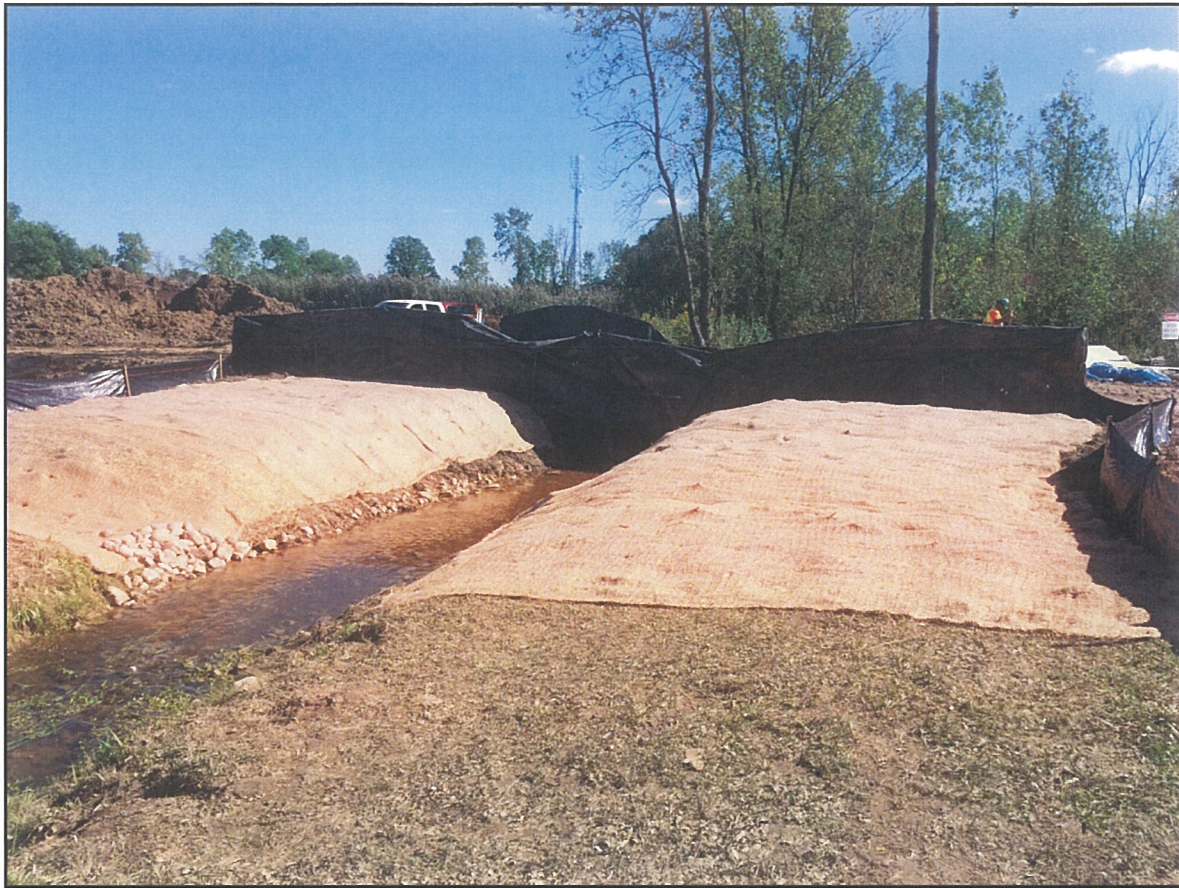
After the watercourse crossing is completed, the watercourse is restored back to pre-construction conditions or better and all disturbed areas are seeded with a creek restoration mix and protected by erosion control blanket and silt fence.
