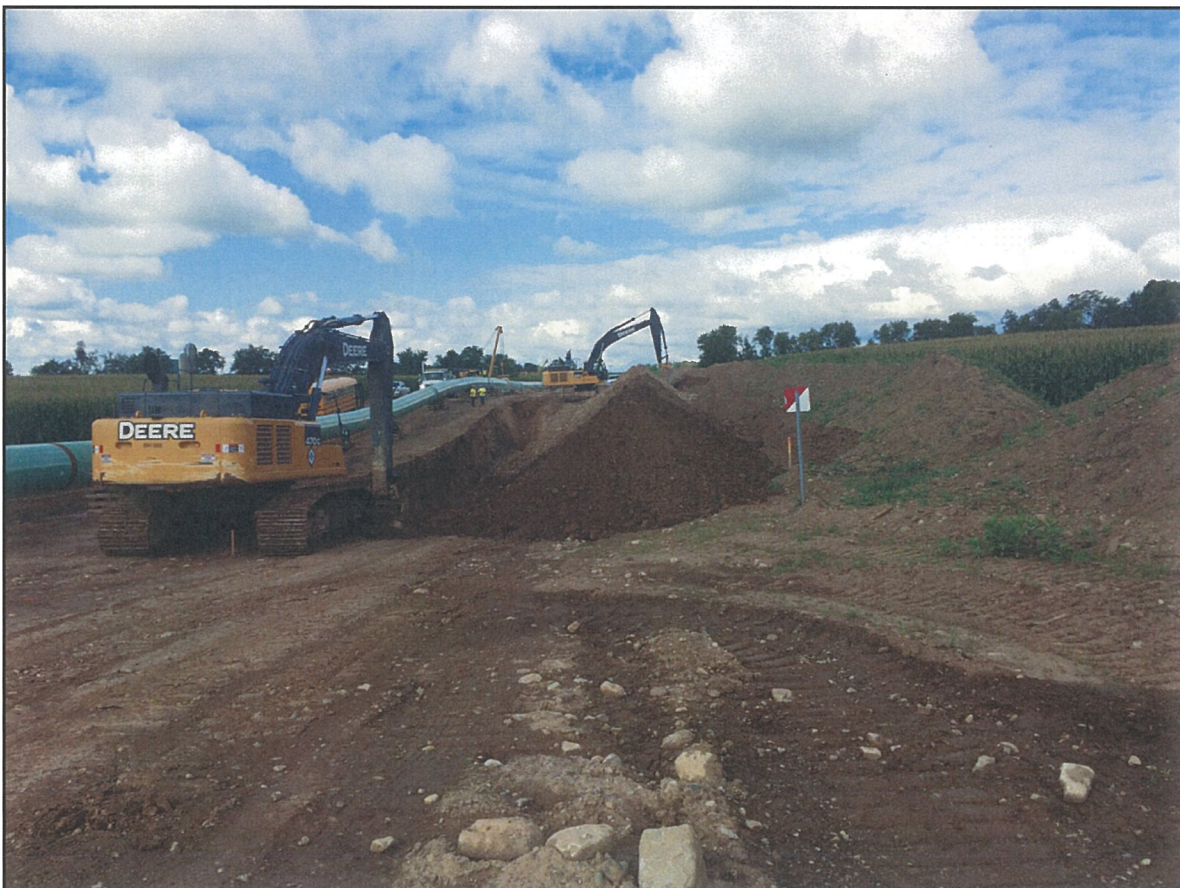
Separation between topsoil and subsoil was maintained during construction to ensure topsoil fertility is maintained.
