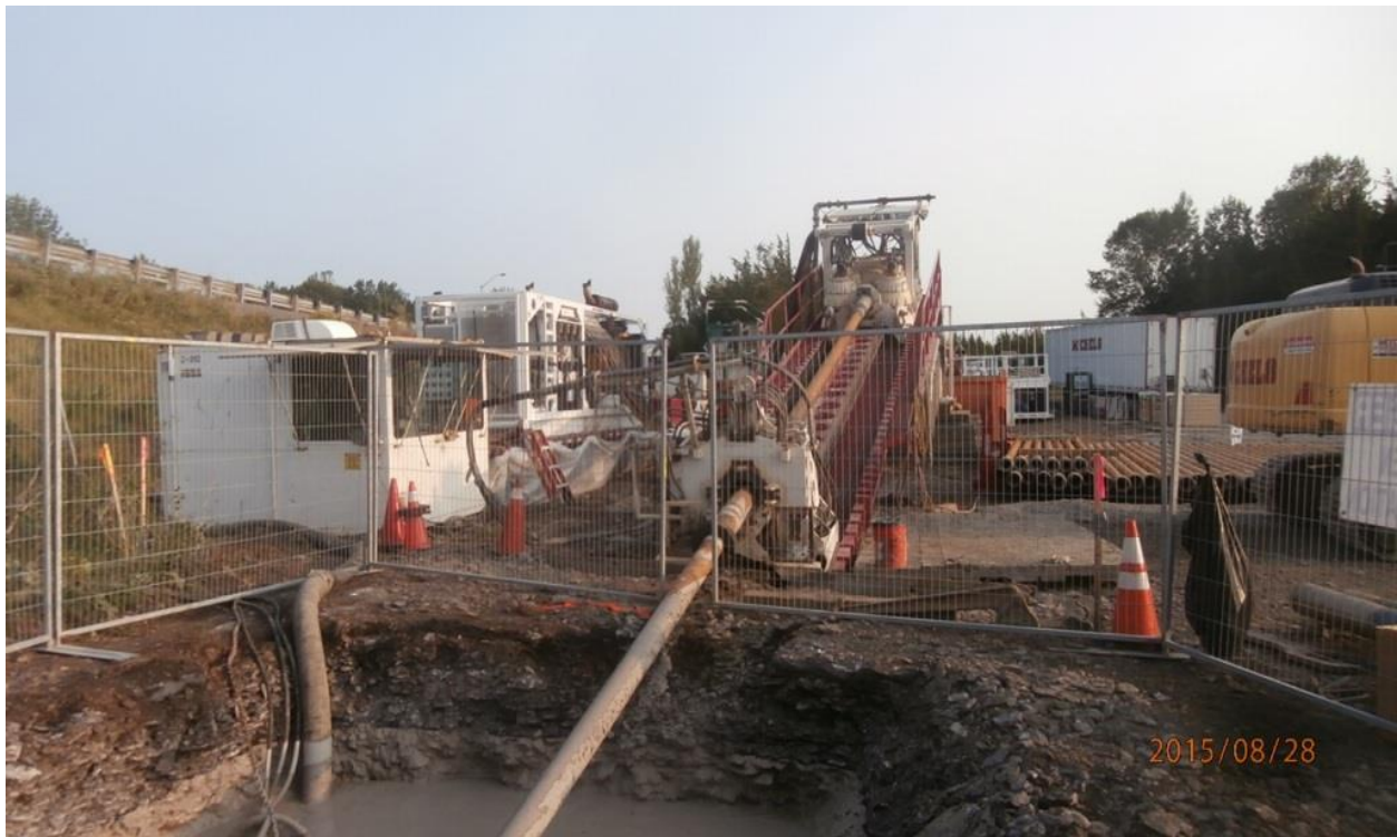
A front view of the drilling rig. A bore pit is excavated where the drill enters the ground to contain the drill fluids which will be recycled.
