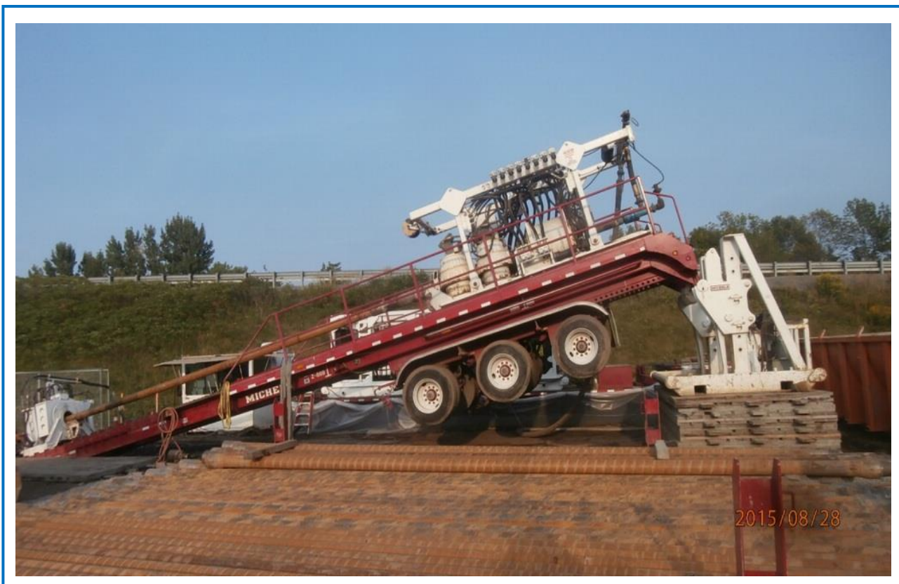
The directional drill machine was set at a precise angle to follow the design of the drill.
