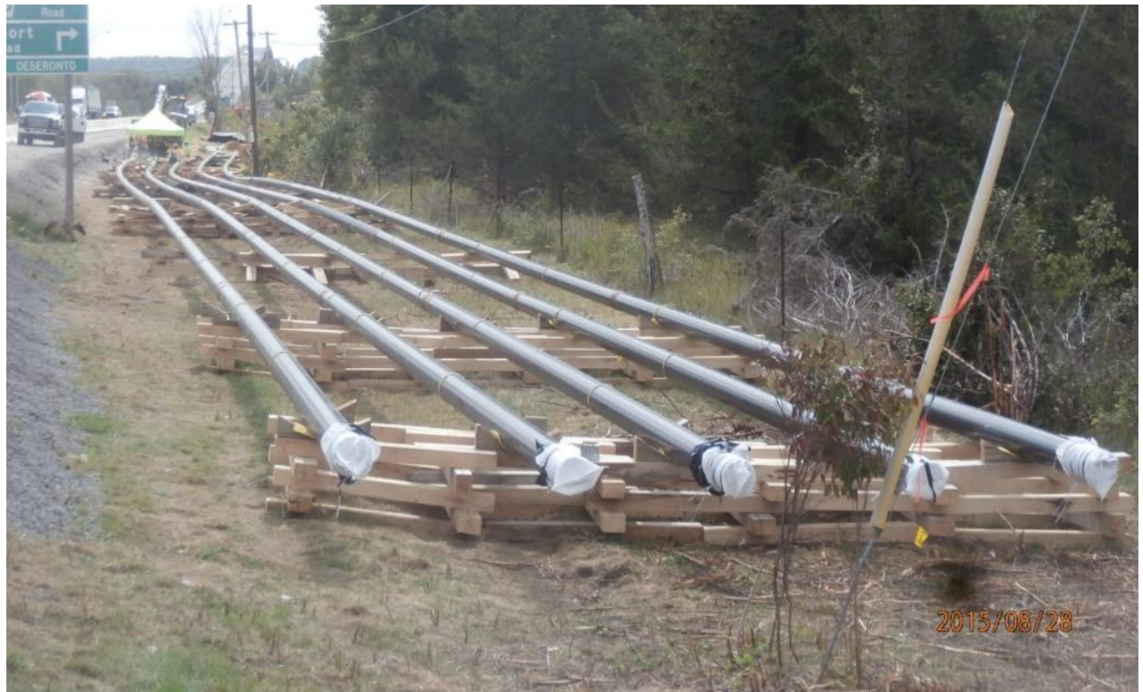
To avoid blocking access to businesses along the west side of Highway 49, the pipe was not welded into a contiguous line. Each pipeline section was pulled into place and another section welded on before continuing the pull.
