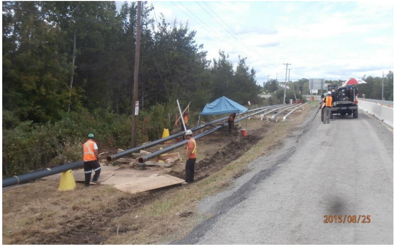
The pipe was strung out along the temporary work zone and welded together.
