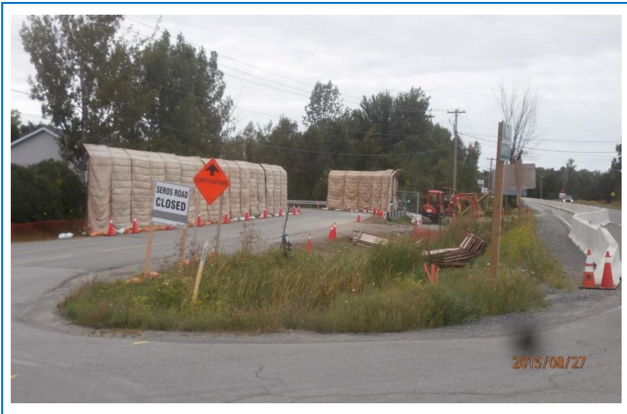
Due to the proximity of construction to residences on Seros Road, a sound mitigation wall was erected
