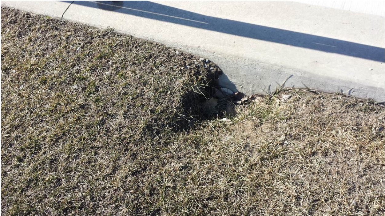
Photos 7: Trench subsidence on the North side of Costco.
