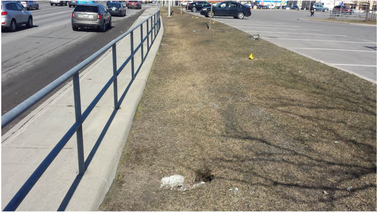
Photos 6: Trench subsidence on the North side of Costco.
