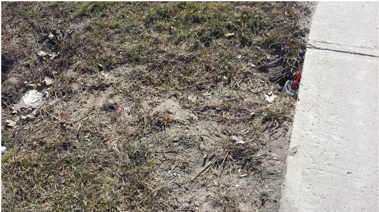
Photo 5: Trench subsidence North West of the Esso Gas Station.
