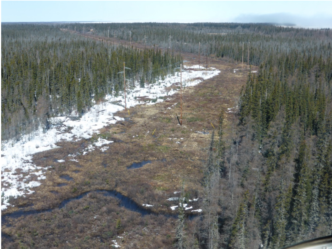
Aerial view of FNEI transmission line
