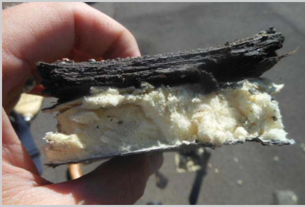
View of core cut reveals 2" polyisocyanurate, 1/8" separation sheet and 2 plies of modified membrane
