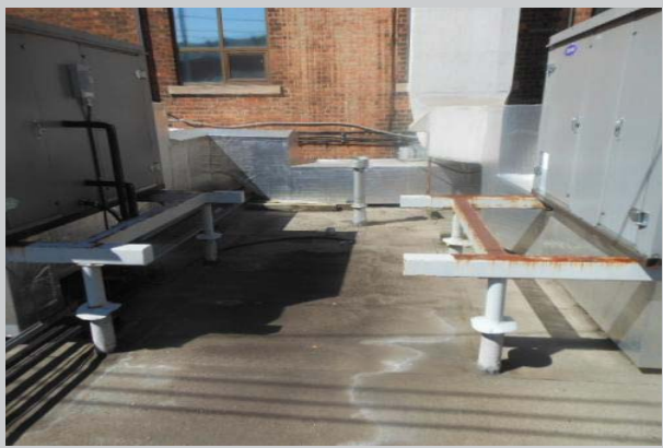
View of ponding water between the large units on section 11
