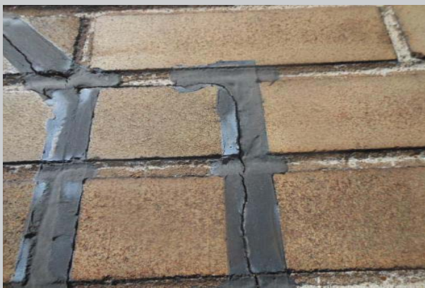
Closer view of current cracks in the brick found in a variety of areas below roof sections 1, 2 and 3.
