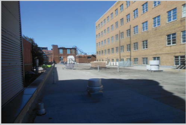
View of small area which was recently replaced. A wall from the firehall fell and collapsed the deck.
