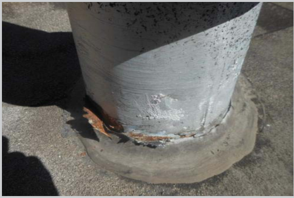
This cone will need to be replaced as the corrosion here has badly deteriorated the base.
