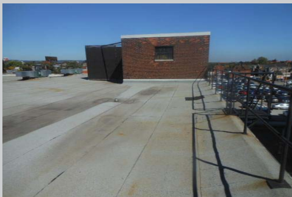
View of section 8 and the poorly installed railing that do not have proper pitch pans (seen on the right). Note the deteriorated membrane in the middle of the roof.
