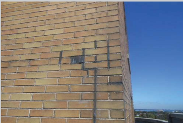
These walls are in very poor shape and should be protected better with new cladding, stucco or a coating.
