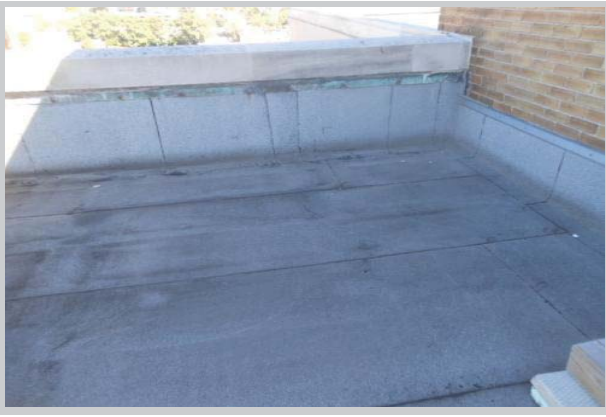
View of badly deteriorated membrane located on the north side of section 3
