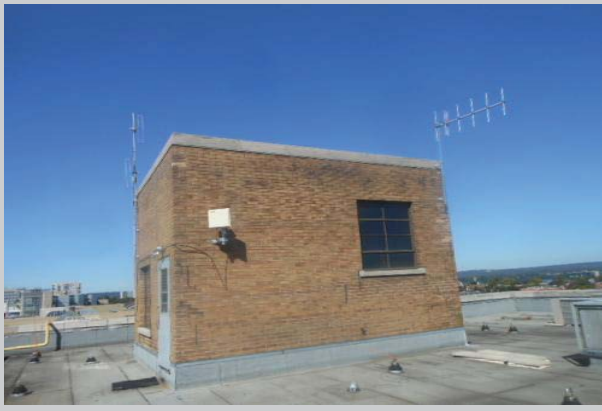
View of penthouse brick work that needs to be better protected as leaks are coming through these walls.
