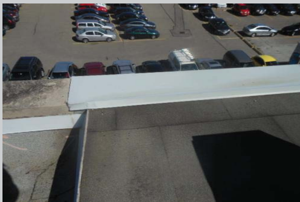
The membrane is in poor shape as seen here on section 8 where it ties into section 9 on the north side.
