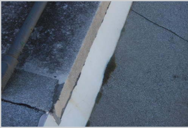
Moss growth from water that is getting from in behind the metal counter flashing.
