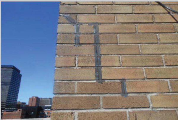
signs of previous attempts to repair the deteriorated mortar in the brick work.
