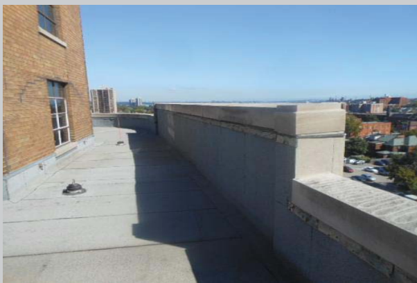
View of the east side of section 4 where an exaggerated cricket/saddle was installed to help with the drainage.
