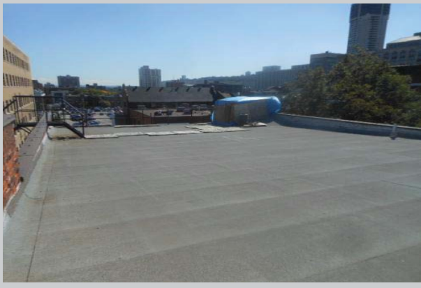
View of section 6 which is sloped 2:12
