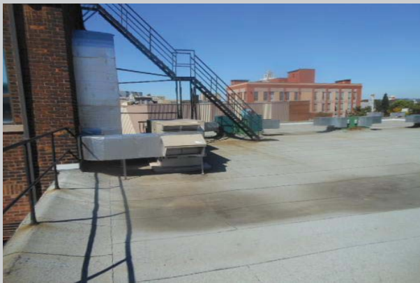
View of deteriorated membrane as seen on the right dark spots
