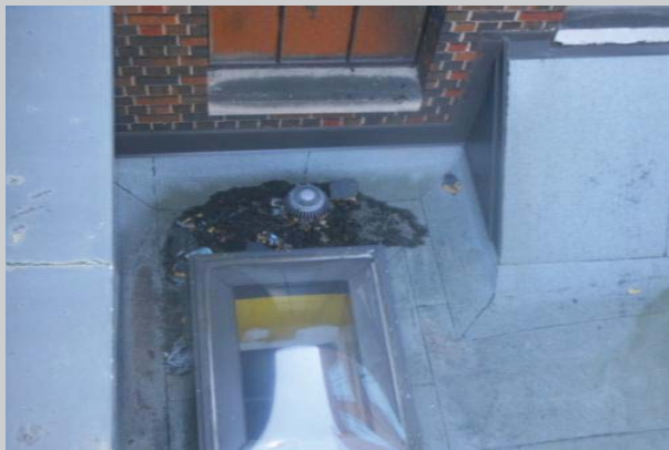
All the debris should be removed from the drain strainer over section 10
