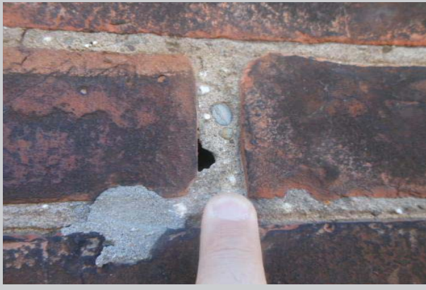
There are some mortar issues along the wall at the lower brick work of section 9
