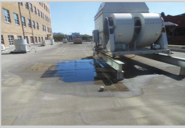
Example of ponding water around one of the larger HVAC units in the middle of the roof.
