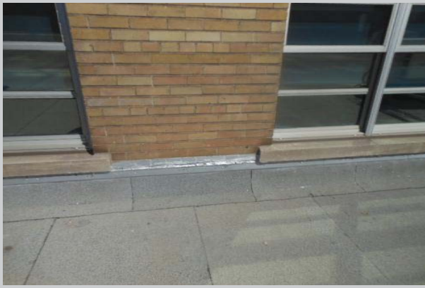
View of perimeter flashing along the base of the windows
