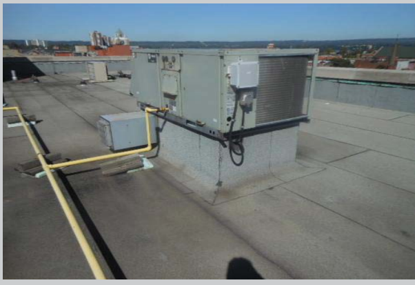
Signs of ponding water to the left of the HVAC unit, towards the middle of the roof section.
