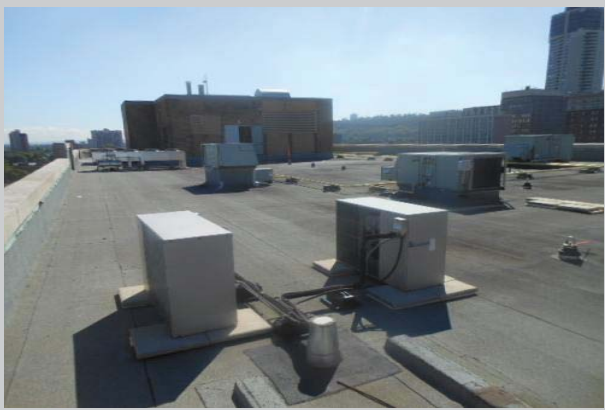
The redundant sleepers should be removed. This is the view from the west side of section 4 facing the east.
