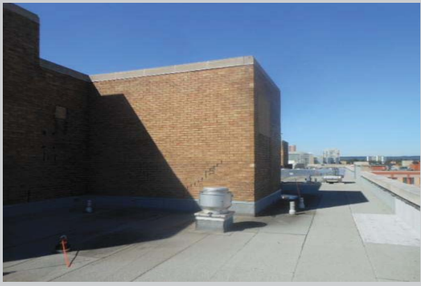
View of the northside of section 4 where a small area was already replaced recently (note lighter grey patch along the perimeter)
