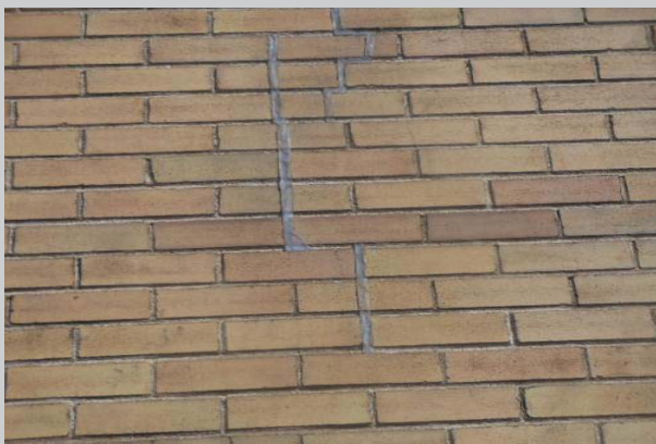
More brick work attempted repairs.
