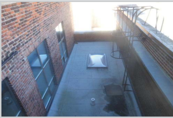
View of section 10, ponding water is excessive on the right
