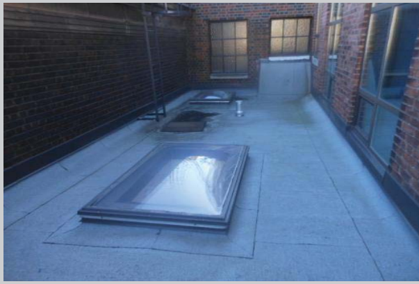
The lower roof #10, This roof has already been replaced because of sloppy workmanship and poor quality material. The insulation was soaked. The roof was replaced in approximately 2007
