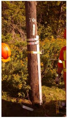
Figure 2: Pole Reinforcement Installation
