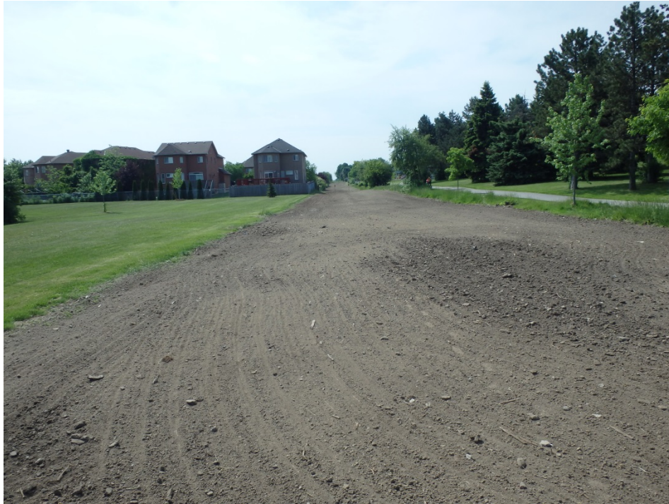
Photo 23 - Condition of ROW adjacent to residential properties directly after seeding (June 2016)
