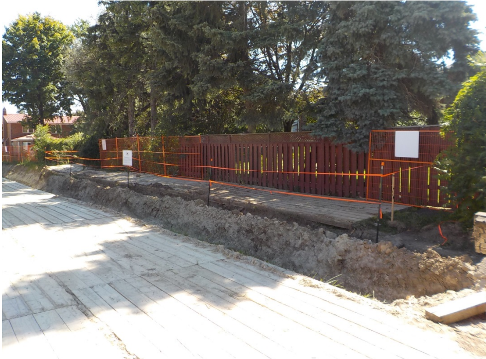
Photo 1 – Typical tree protection zone set up in Segment B (July 2015)
