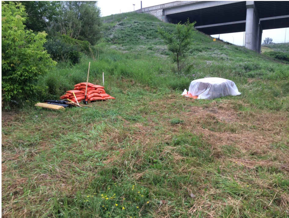
Photo 3 – Preparing HDD contingency equipment near the East Don River Channel (June 2015)
