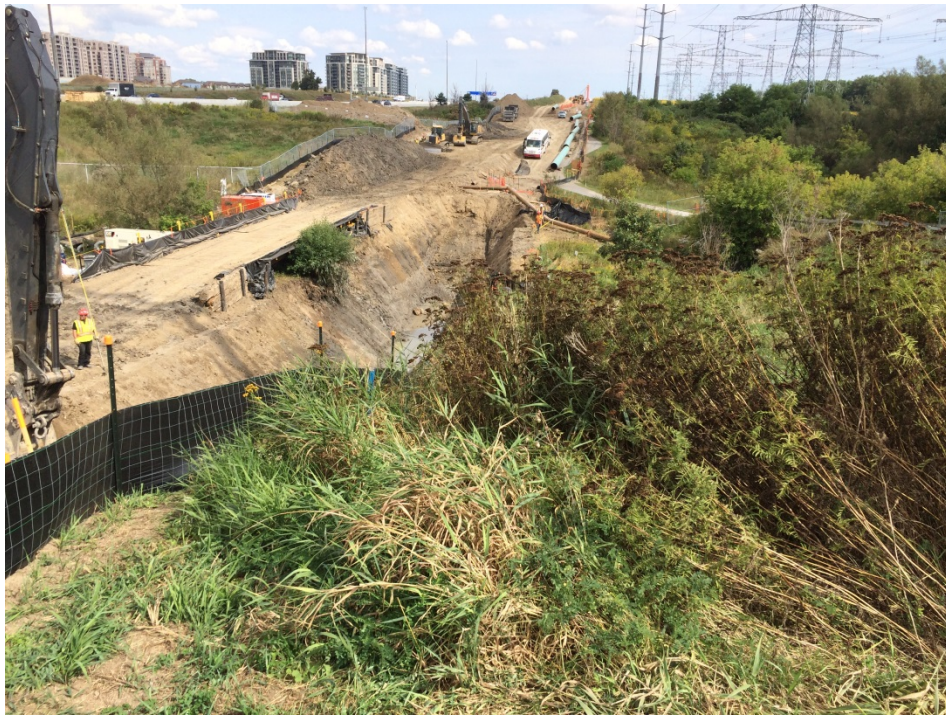
Photo 8 – Completing the isolated open cut on German Mills Creek (September 2015)
