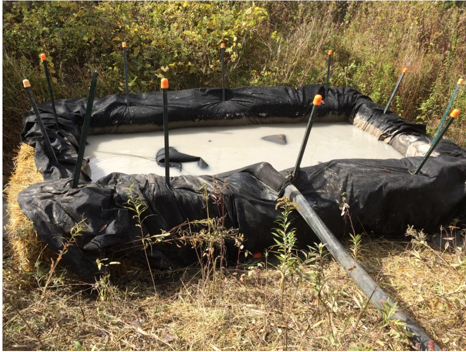
Photo 35 – Churchville-Norval PSW - establishing initial sediment basin (October 2015)
