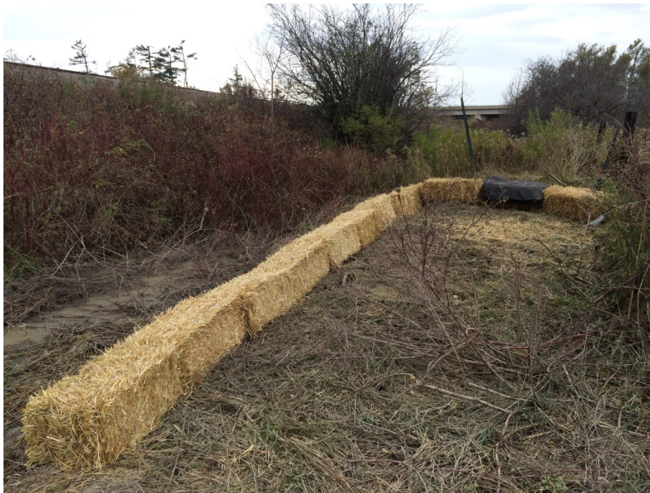
Photo 37 – Churchville-Norval PSW – establishing secondary straw bale check dam for filtering which was later transitioned into a basin (October 2015)
