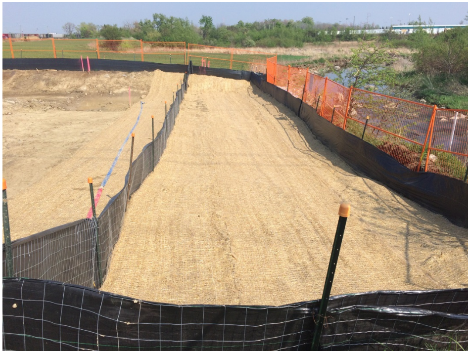
Photo 28 – Etobicoke Creek restoration along the banks of the creek as per TRCA recommendations to resolved non-compliance (April 2015)
