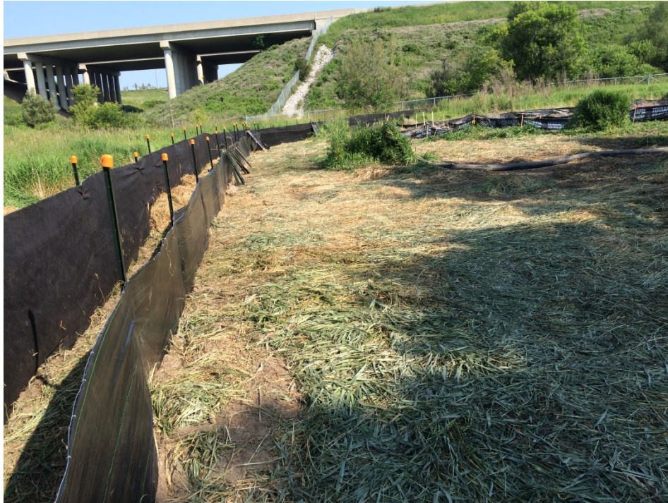
Photo 5 – Establishing secondary containment of the IFR from watercourse using double rowed sediment fence and straw bales at the East Don River (July 2015)
