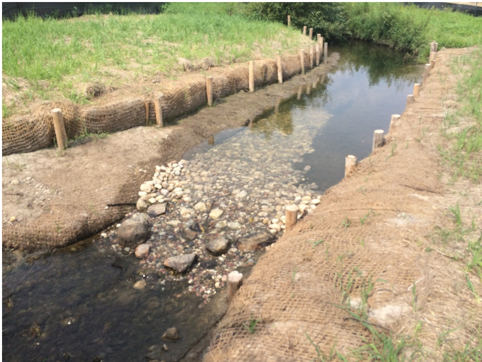
Photo 12 – Bed and bank restoration at Little German Mills Creek (July 2015)
