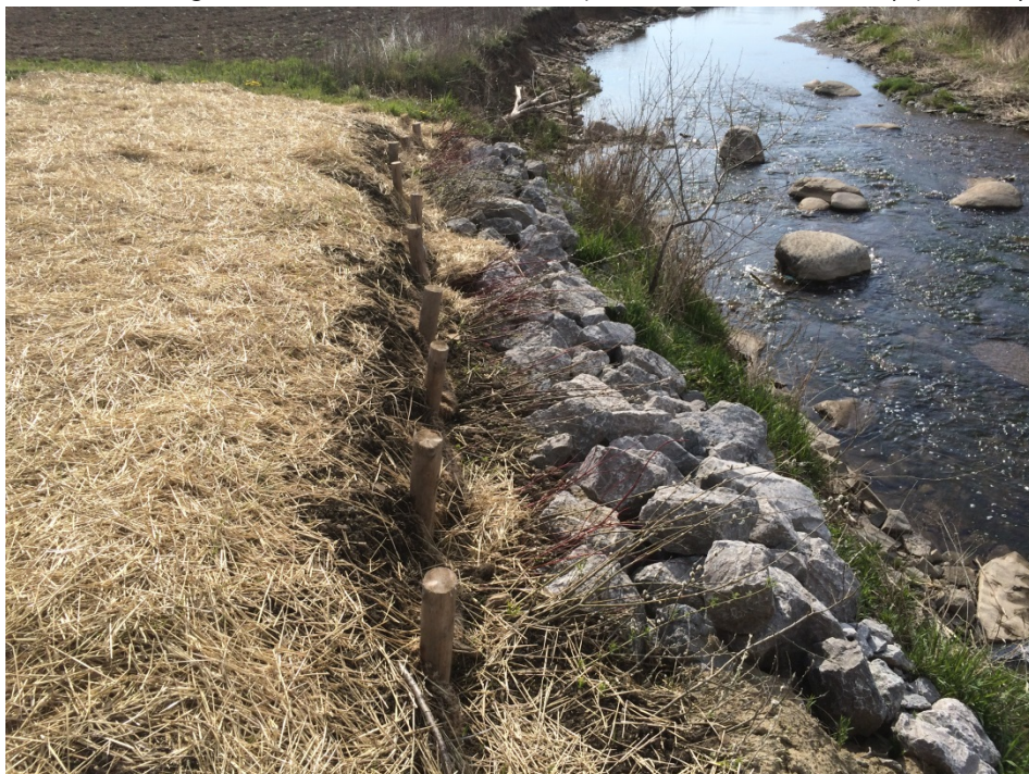
Photo 30 - Etobicoke Creek after final bank restoration (May 2016)
