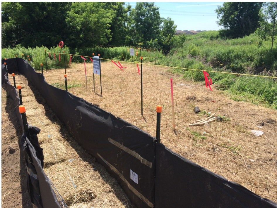
Photo 32 – Establishing sediment fence barrier and signage at Fletchers Creek (July 2015)
