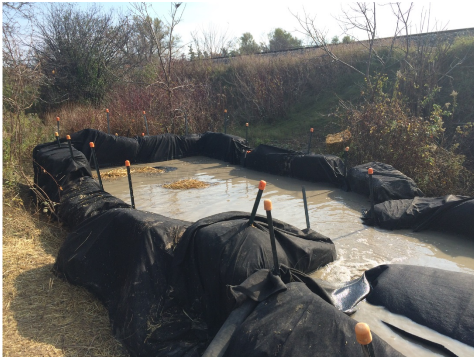
Photo 36 - Churchville-Norval PSW – establishing secondary chambered sediment basin (October 2015)
