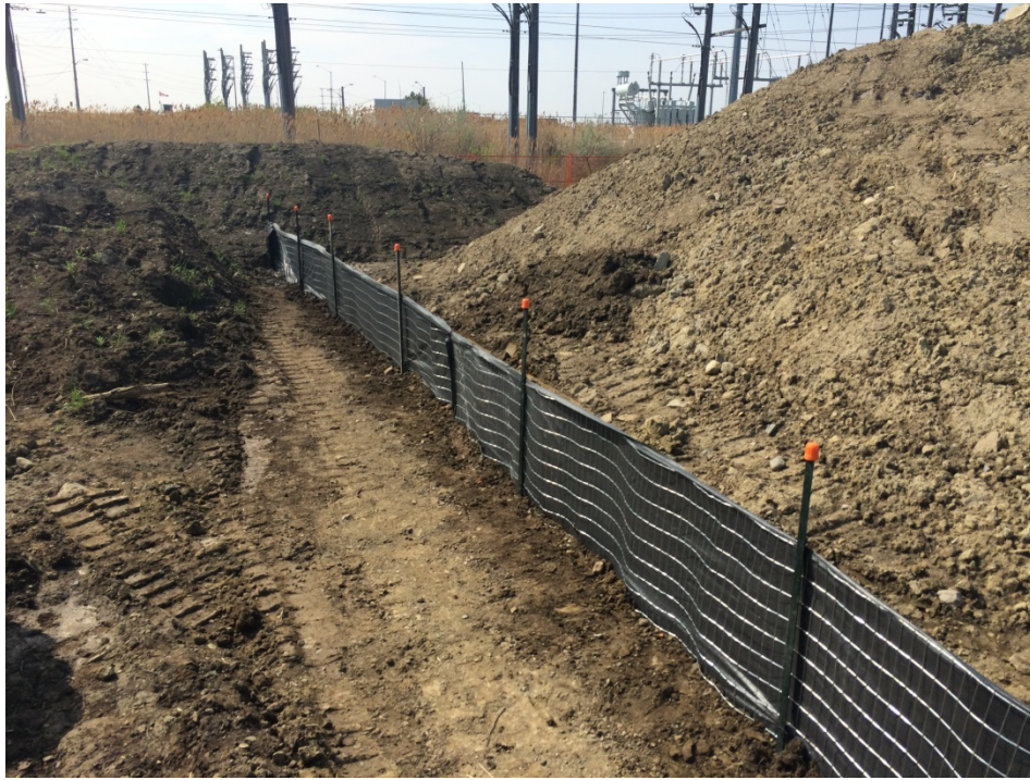
Photo 29 – Placing sediment fence around stockpile at Etobicoke Creek (April 2015)
