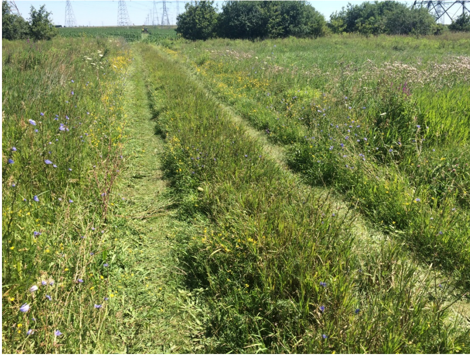
Photo 33 – Condition of HONI access road near Eighth Line prior to improvements (April 2015)
