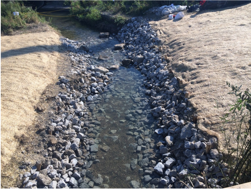
Photo 9 – German Mills Creek immediately after restoration and temporary stabilization (September 2015)
