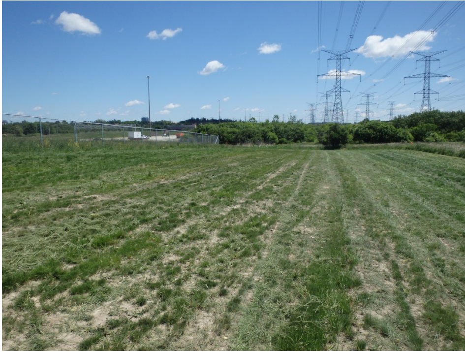
Photo 25 – Condition of ROW in area seeded in 2015 (June 2016)
