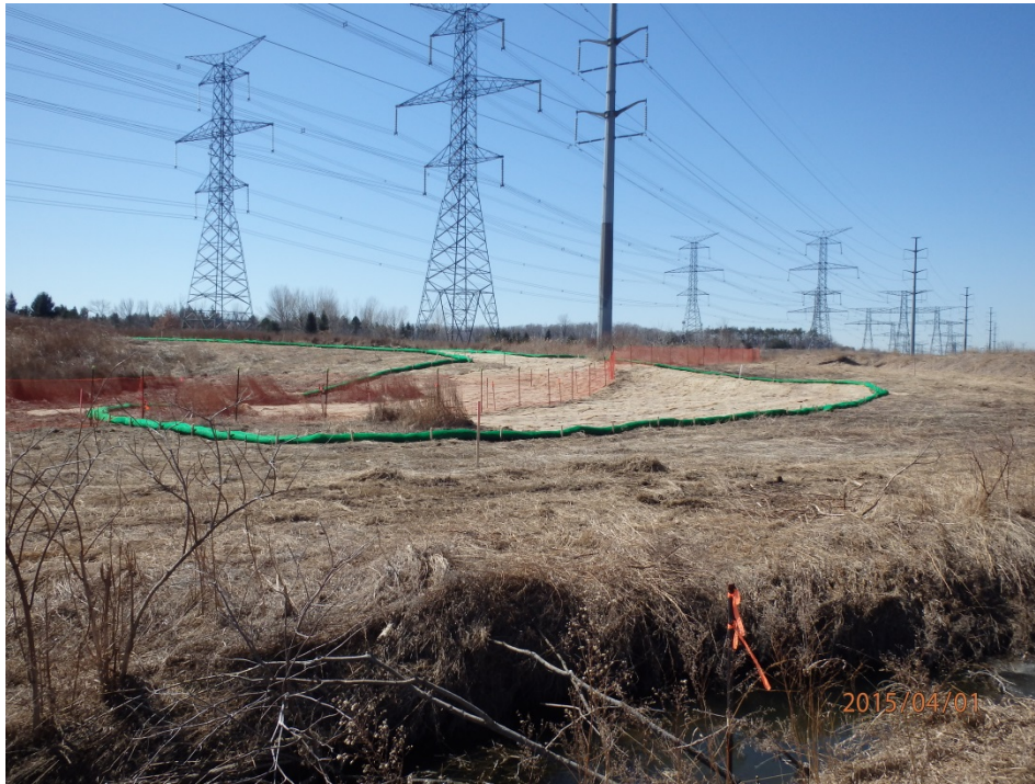
Photo 19 – Erecting snow fence and ESC mitigation measures to delineate the Goin Archaeological Site prior to construction (April 2015)
