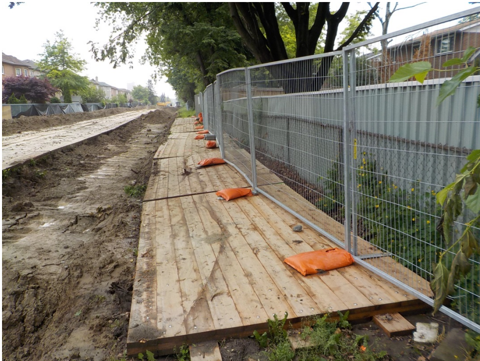
Photo 2 - Typical tree protection zone set up in Segment B (July 2015)
