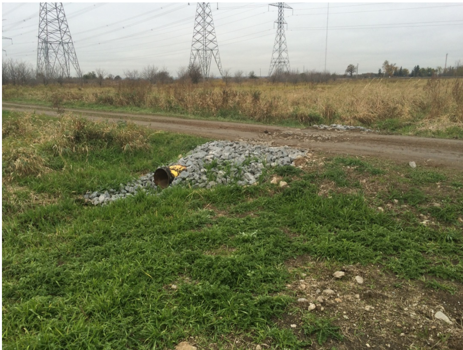
Photo 34 – Culvert replacement on HONI Access road near Eighth Line (October 2015)
