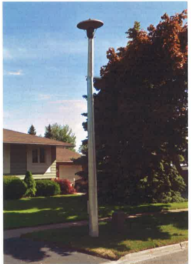
New Streetlight Pole & Secondary Pedestal
