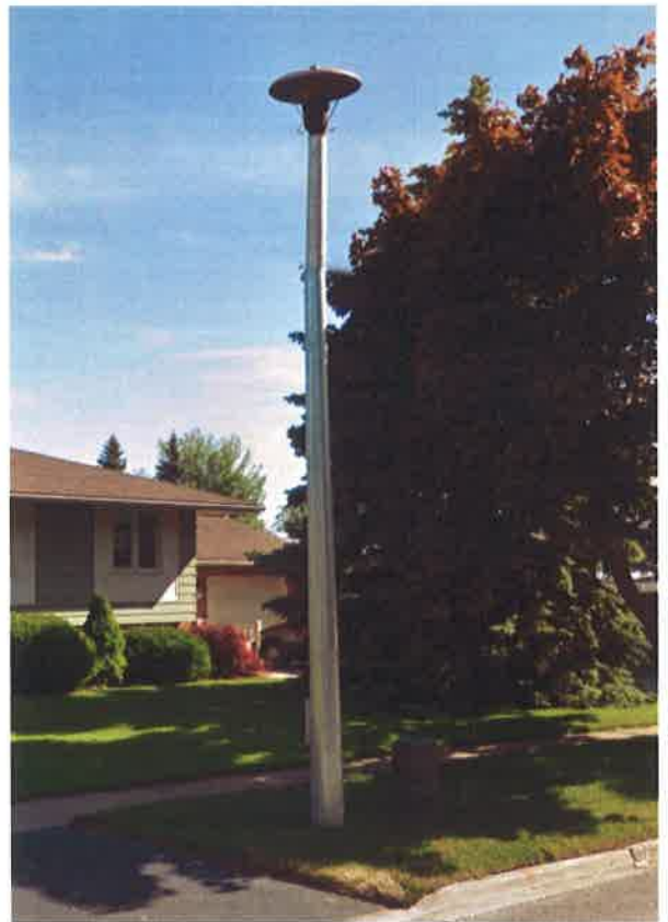
New Streetlight Pole & Secondary Pedestal
