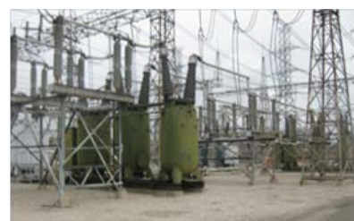
Oil Circuit Breaker in poor condition
