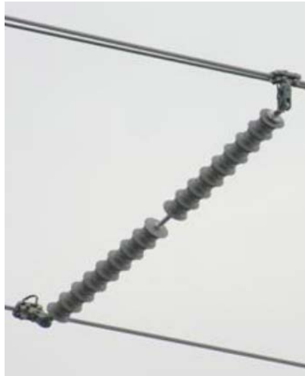
Figure 7-6 – Inter-Phase Spacer
