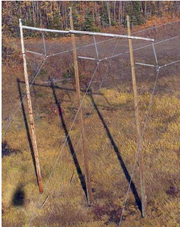
Figure 7-5 – Semi-Strain (L21S, structure 4, 230 kV, polymer)
