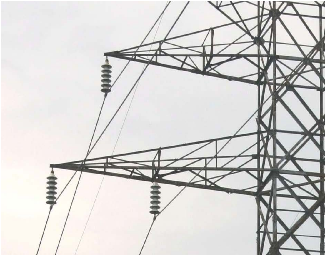
Figure 12-1 - Semi-conductive-Glaze Bell-Shaped Insulators (C14L/C17L, str 7, 230 kV, porcelain)
