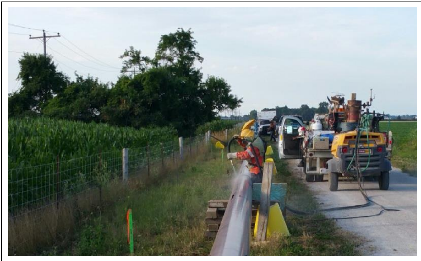
After two sections of pipe have been welded together, the joints are sand blasted to remove any impurities and rust and then an epoxy coating applied. For safety, the worker must wear protective clothing and a helmet with a
