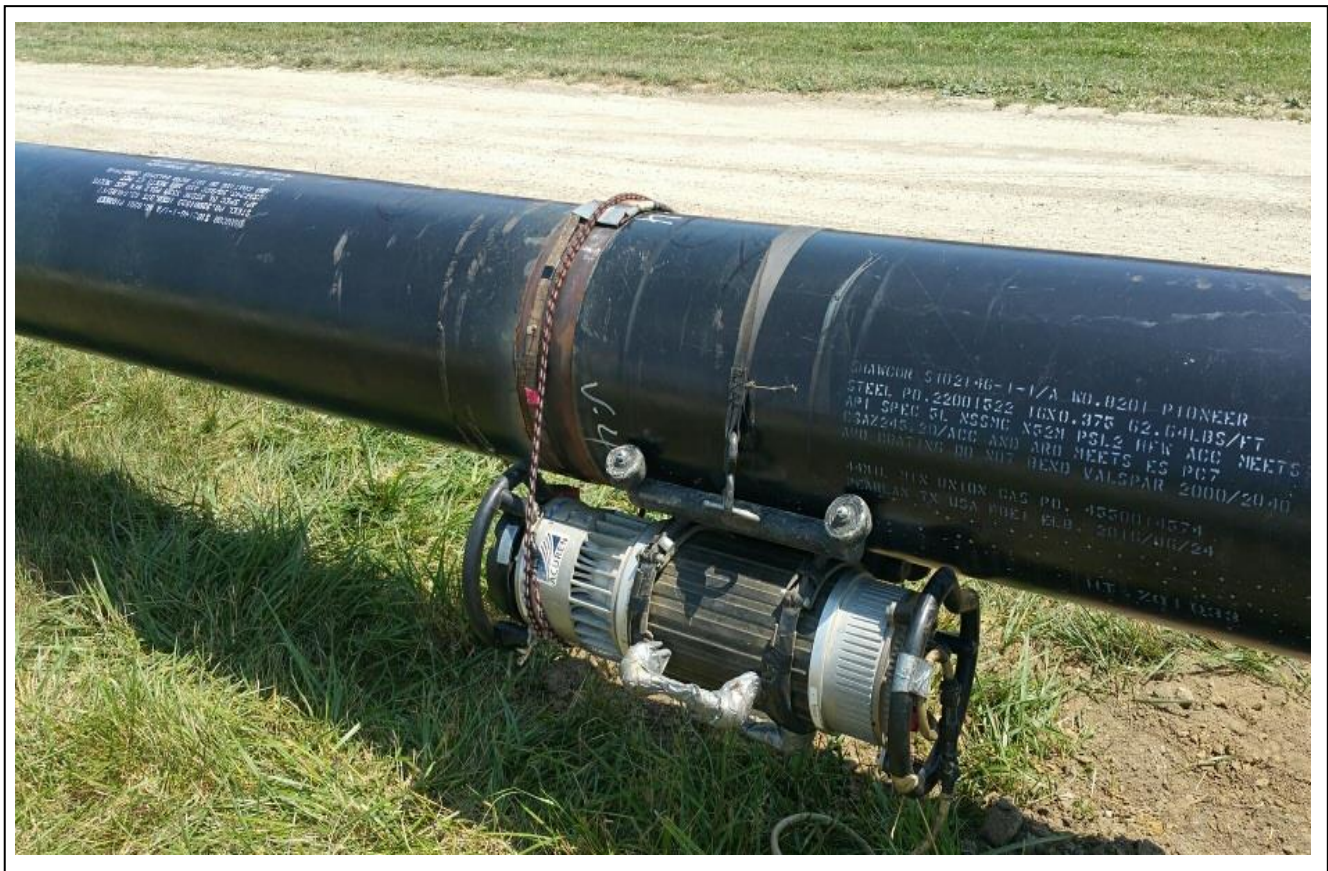
All welds are x-rayed to ensure the safety and integrity of the pipeline.
