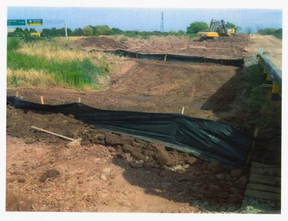
When a crossing is "open cut" it must be restored to original state the day of. The above picture shows SC14 being restored with top soiled and seeded with silt fence back in place to prevent any siltation from entering the channel.
