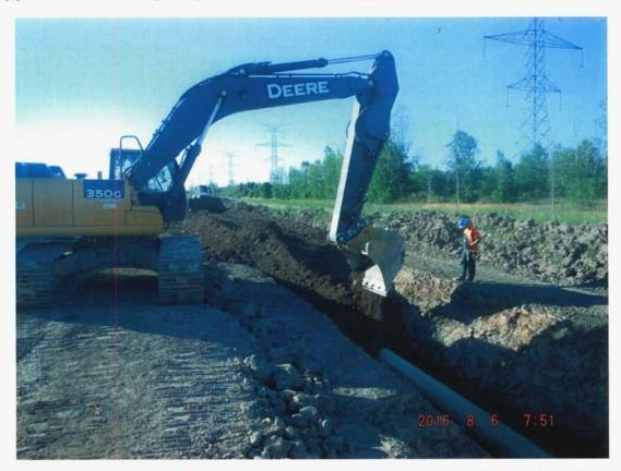
After the pipe has been laid in the ditch the survey crew walks along and shoots every weld before backfill begins. Backfill starts with "shading" which is the excavator covering the pipe gently with approx. 2ft of material for protection before the full backfill is completed. A spotter is present at all times watching for rocks that could potentially damage the pipe.
