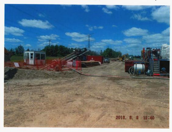
Some areas such as creek crossing and road ways cannot be excavated so a Horizontal Direction Drill (HDD) is used to bore a hole in the ground and pull the pipe through with no surface disturbance.
