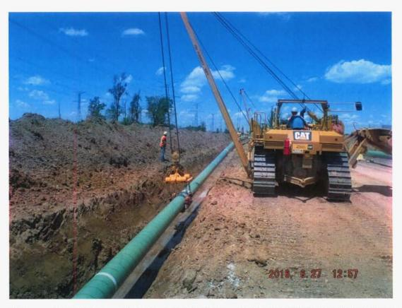
Once the ditch is completed side booms using cradles pick the pipe up and slowly roll it into the ground. During this process the entire pipe is checked for coating damage one last time with the Jeeper before it is buried.
