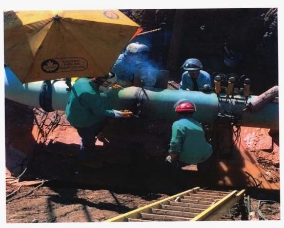
Pipe is then fitted up and welded together by a team of welders using one on each side. Four passes are made to complete the weld and upon completion each weld is given a visual inspection and x-ray by a third party company.
