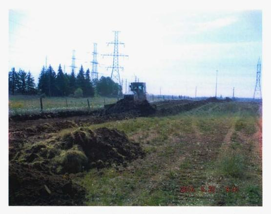
Measurements are taken to distinguish between topsoil and subsoil. A dozer is then used to perform the operation of separating the two layers.
