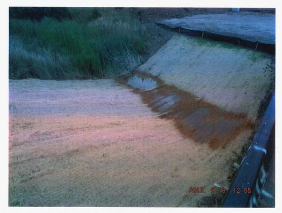
After the topsoil and seed have been replaced an erosion matting is laid down and secured over top to prevent bank/channel erosion and promote seed germination.
