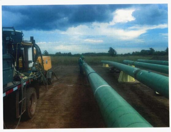
After the pipe is welded together the coating process begins. First step of the coating process is to sand blast the area of the weld down to bare metal so coating can be applied.
