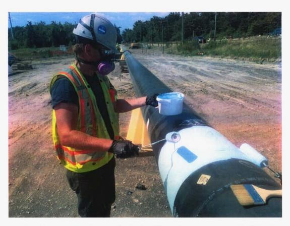
After the pipe is blasted down to bare metal two qualified and certified workers mix an epoxy coating "kit" and spread the product evenly over the bare metal using paint brushes and rollers.
