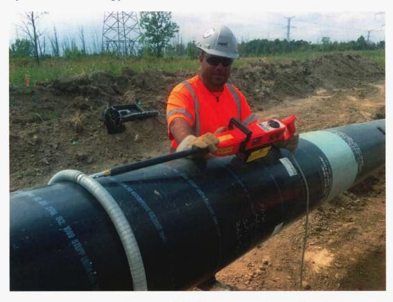
Upon the coating curing, QC tests are carried out to verify the thickness and consistency of the paint Once QC is completed the tool shown above known as a "jeeper" checks for any other spots that may have been missed.
