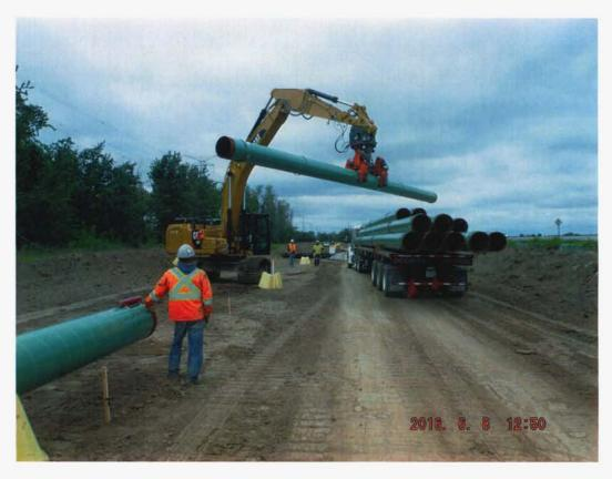
Upon completion of the topsoil stripping, the pipe is strung out along the easement to be welded together. Pipe is placed off the ground on cones and wooden skids to protect the coating from damage.
