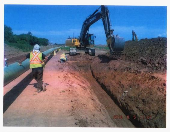
After the pipe has been welded and coated excavators are used to dig the ditch or trench where it will be installed. The running line and depth of this trench is laid out using GPS survey equipment to ensure maximum accuracy.
