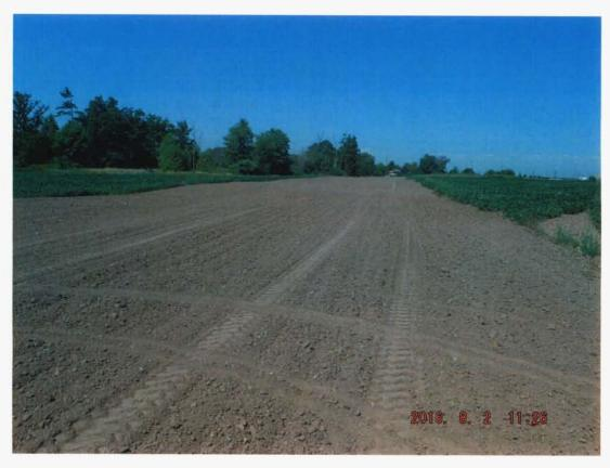
When the pipe has been backfilled the R.O.W is the sub graded and top soiled back to its original state. Shown above is a section of farm land completed and ready to be turned back to the land owner.
