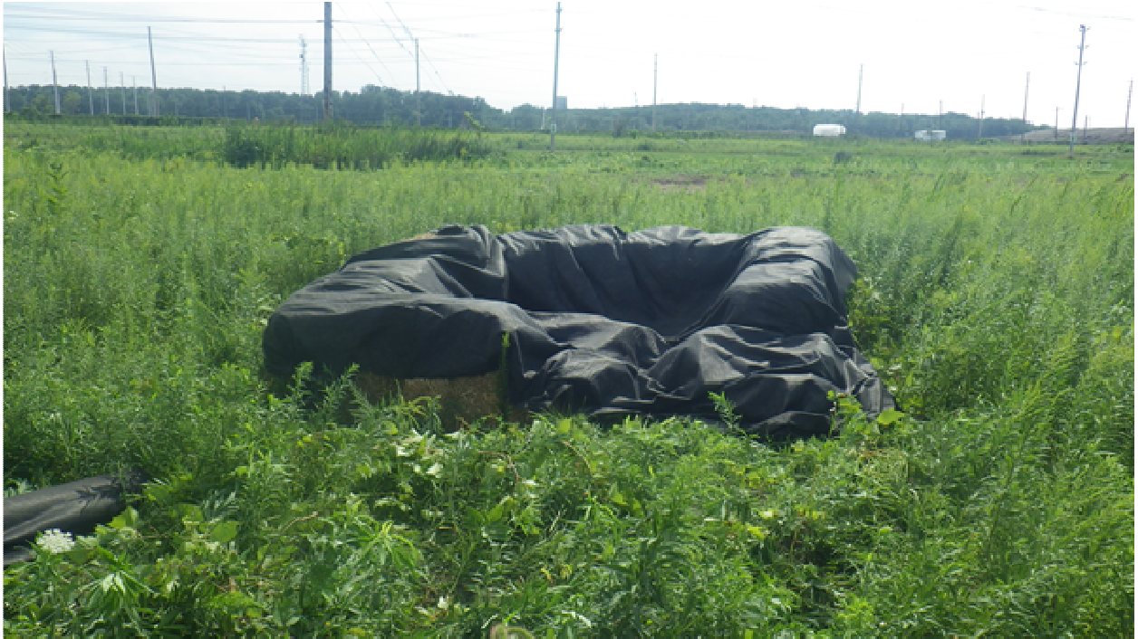
Filtration tub used to dewater Frac tanks following the hydrostatic test.
