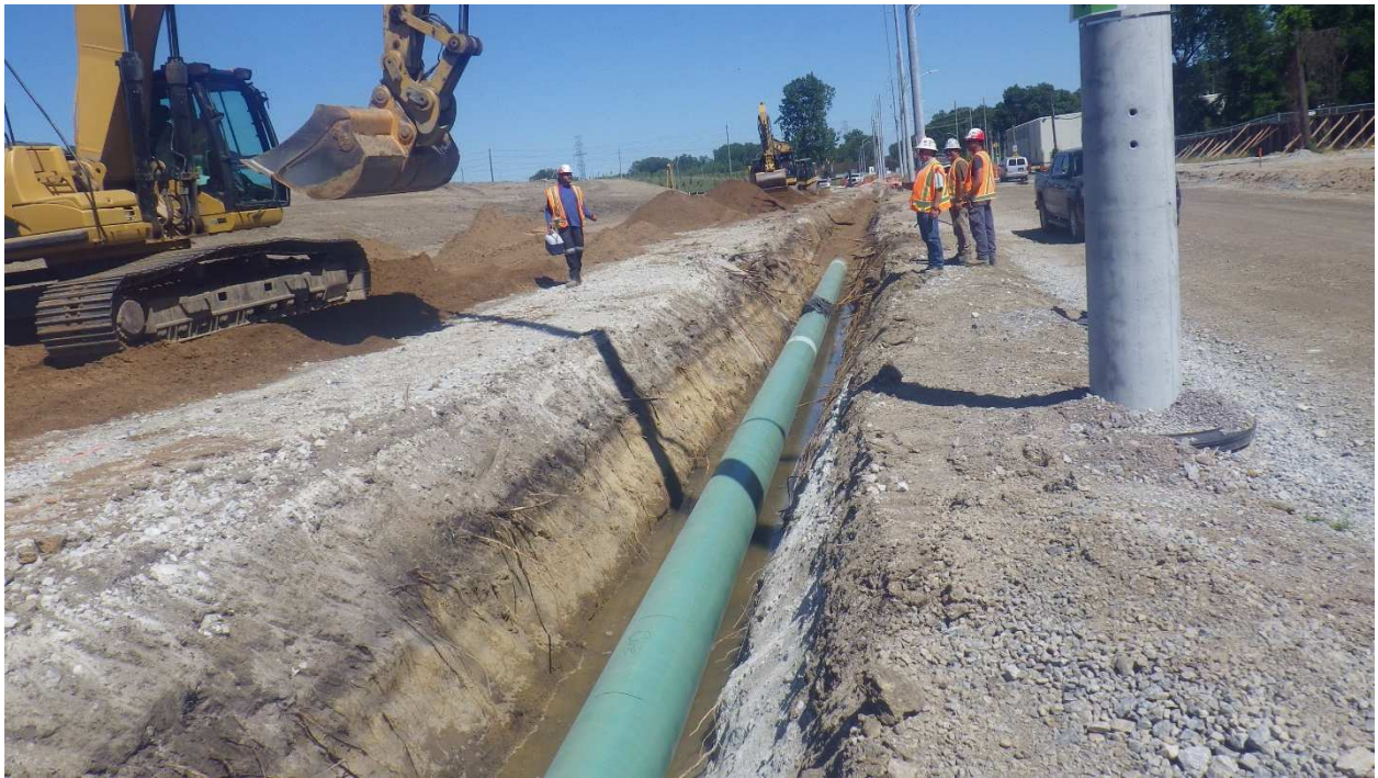
20" pipe lowered into trench along Broadway and sand backfilling.
