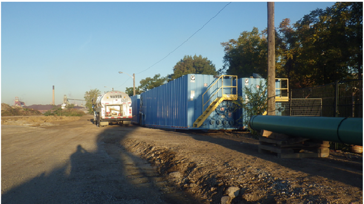
Amico water truck filling up frac tanks with water from local municipal source for hydrostatic testing.
