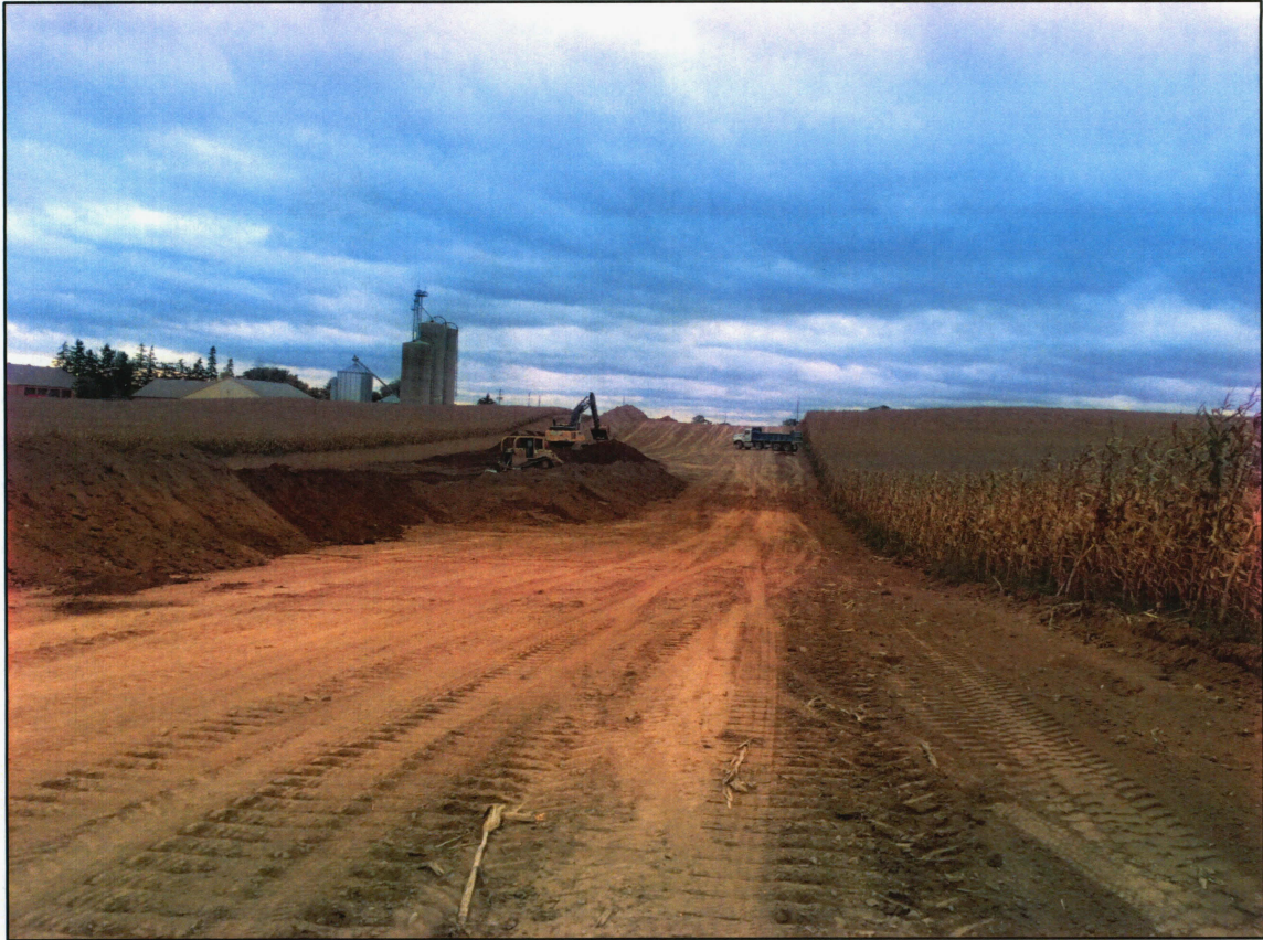
A chisel plough is used to relieve subsoil compaction and then stones are picked manually and with skid steers. Once the subsoil is ready, the topsoil is spread across the right-of-way, as pictured.
