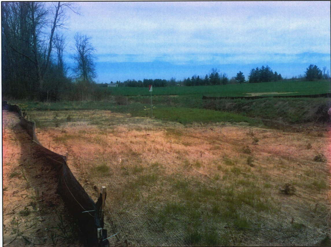
All watercourses were monitored in spring 2016 to determine if there was adequate vegetative growth/stabilization on the banks. As vegetation had not fully established itself, all sediment and erosion controls were left in place.
