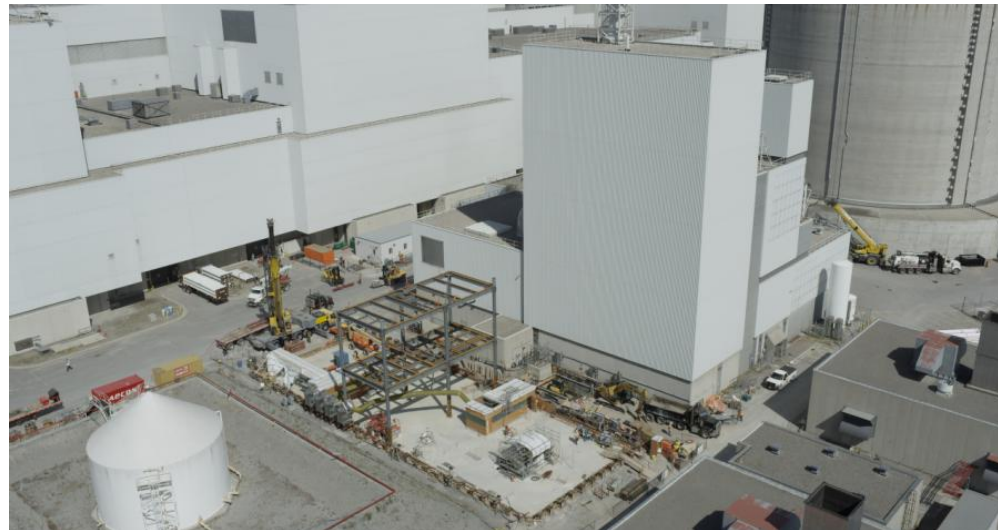
Erection of Structural Steel
