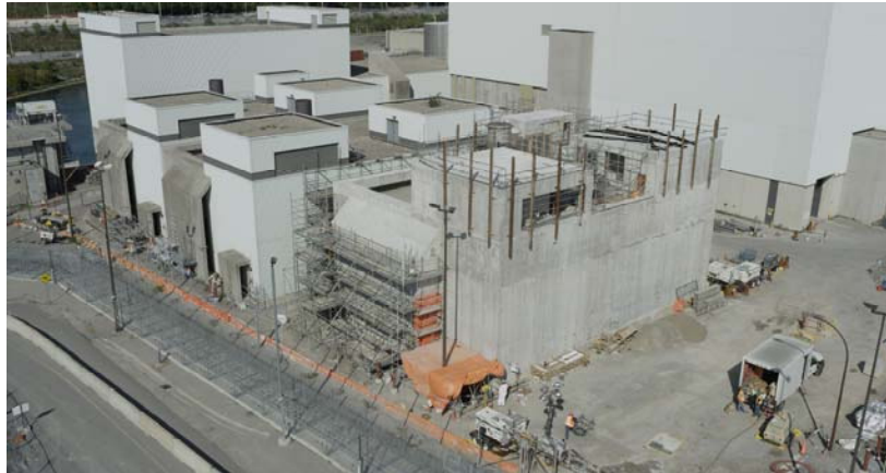
Completion of Civil Work
