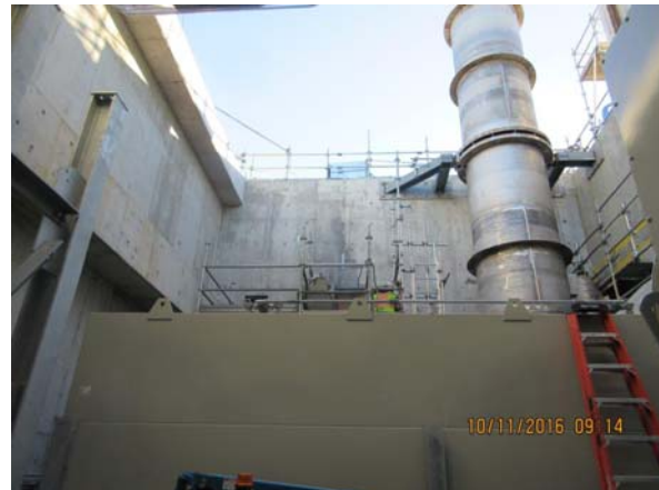
Stack Installed
