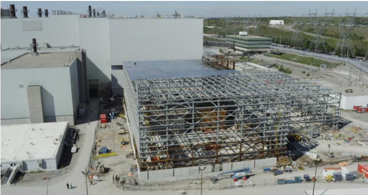
Erection of Structural Steel
