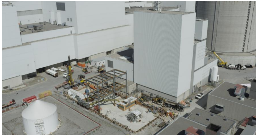
Erection of Structural Steel
