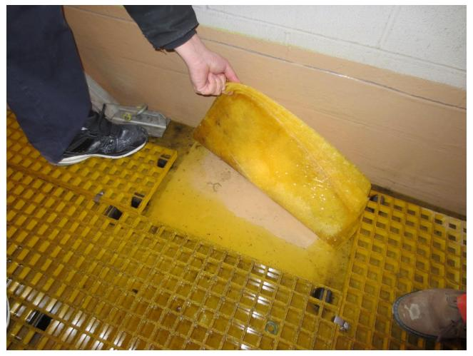
Picture of T1's bay showing puddles of oil accumulated on the ground (Picture taken 2015 Q1)
