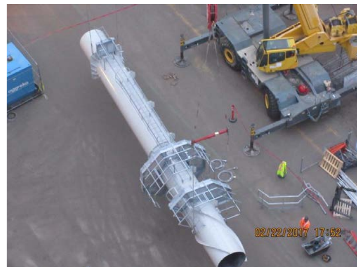
Installation of Landing Scrubber Stack
