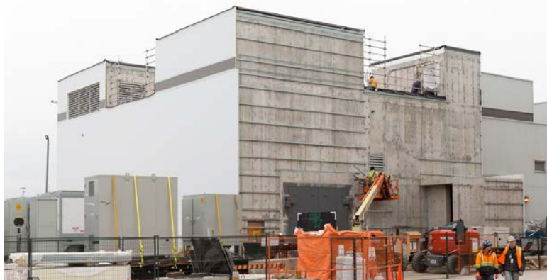
Installation of External Cladding
