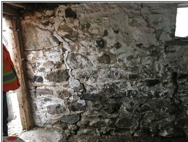
Photo 1: E1 – View of a crack on south foundation wall in the basement
