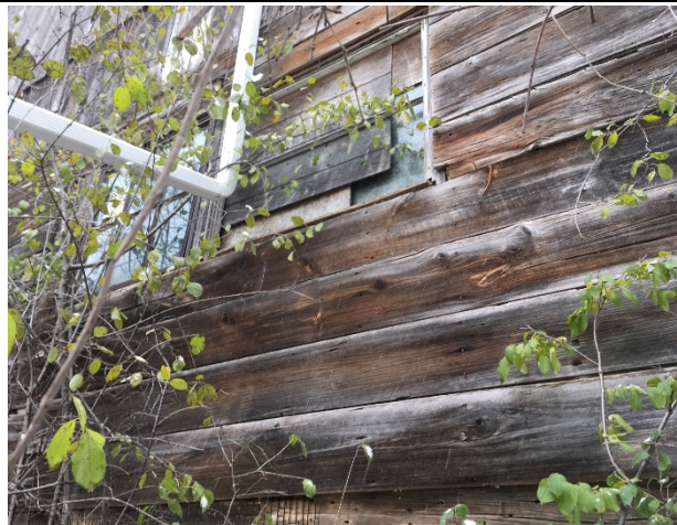
Photo 41: E21 – View of the boarded damaged window and damaged wood boards on the south elevation
