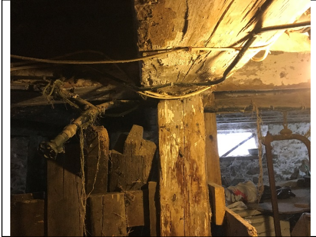
Photo 31: E16 – View of the wood post and floor joist in the basement
