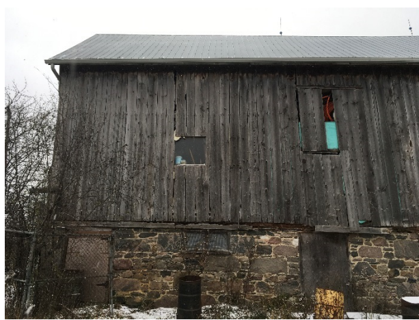
Photo 51: E26 – View of the damaged wood boards on the east elevation
