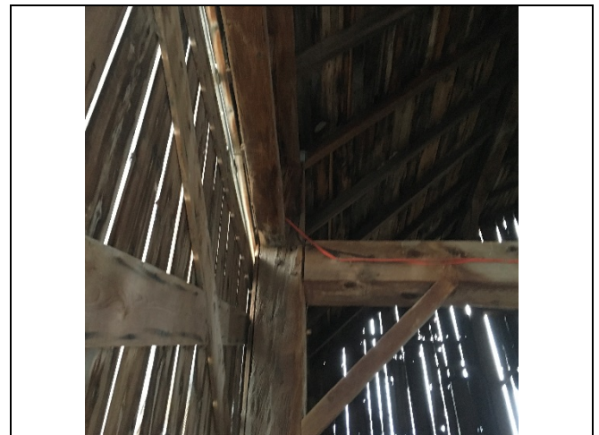
Photo 36: The condition of the wood roof frame structure appears to be consistent with the pre-construction assessment.
