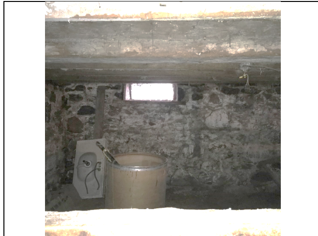
Photo 8: No significant change to the condition of the west foundation wall was observed following the construction.
