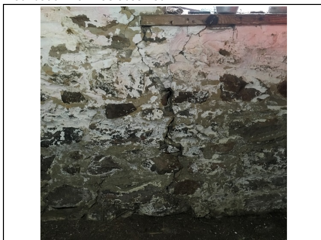
Photo 4: No significant change to the crack on the south foundation wall was observed.
