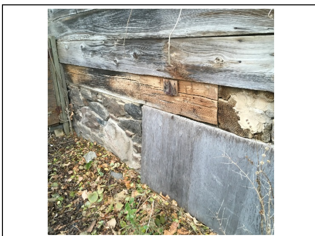
Photo 46: No significant change to the south elevation damaged wood boards was observed.
