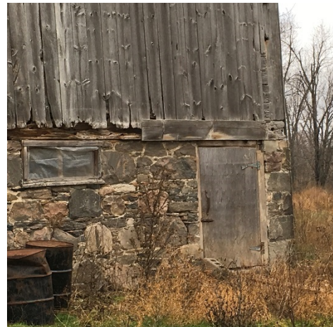
Photo 54: No significant change to the damaged wood boards was observed on the east elevation.
