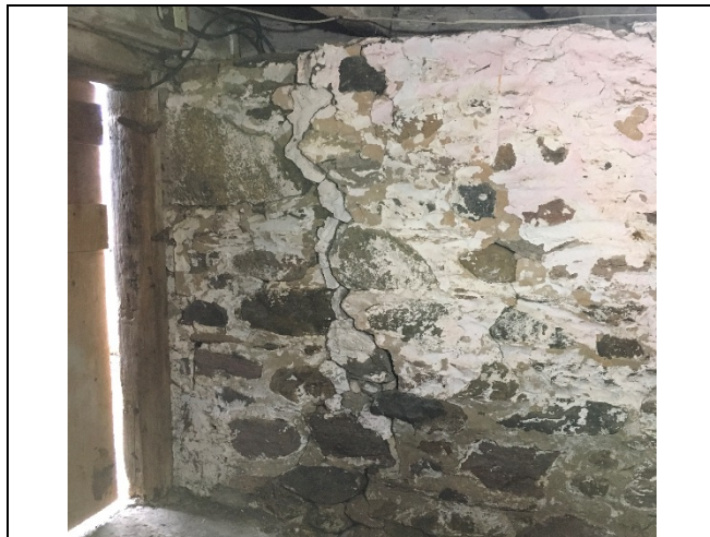
Photo 2: No significant change to the crack on the south foundation wall was observed.
