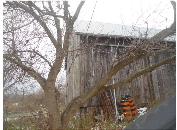
Photo 57: E29 – View of the west elevation
