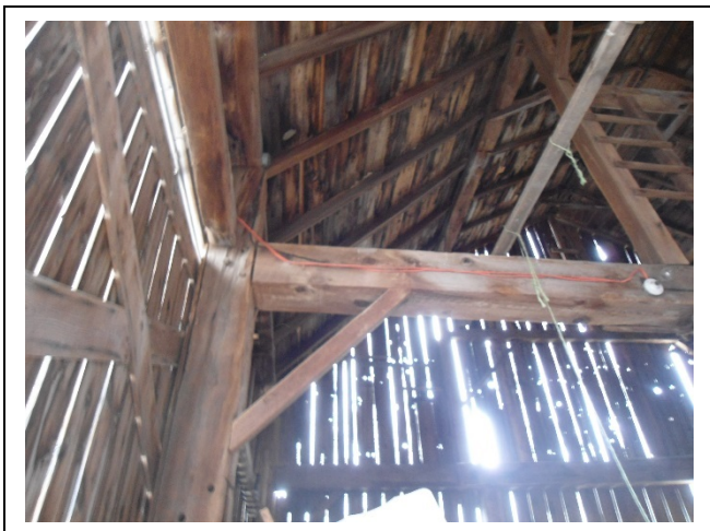
Photo 35: E18 – View of the wood frame structure
