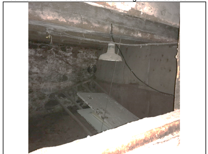
Photo 10: No significant change to the west foundation wall.
