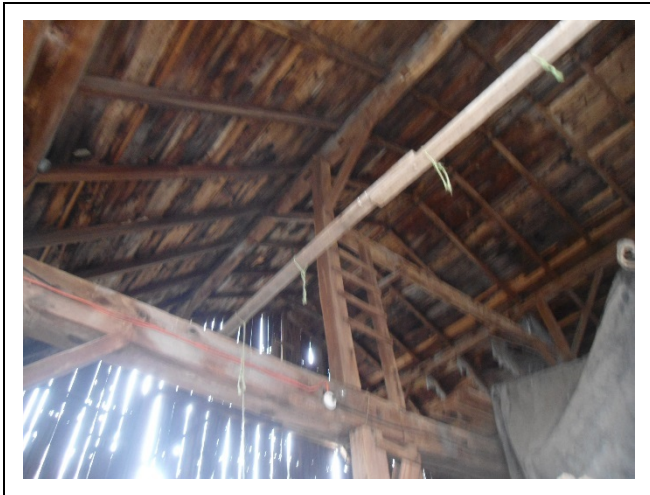
Photo 33: E17 - View of the first floor wood roof frame structure
