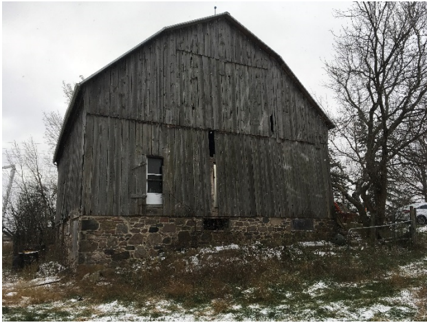
Photo 55: E28 – General view of the north elevation
