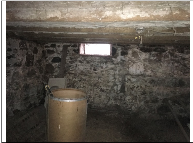
Photo 7: E4 –View of the west foundation wall
