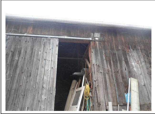
Photo 61: E31 – View of the wood boards above the sliding door
