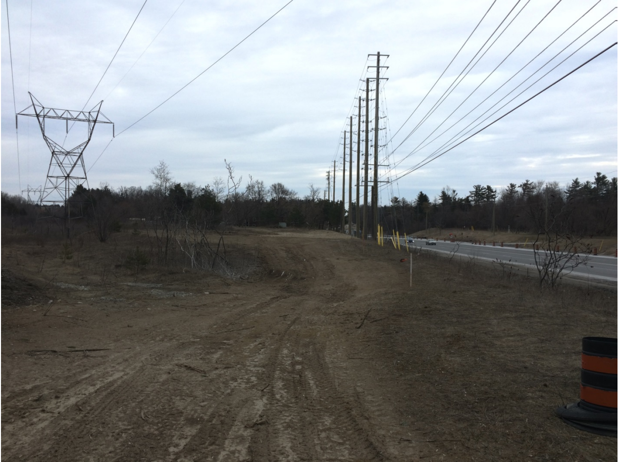
Photo 11: West of Ganatsekiagon Creek looking east. Hydro corridor crossing.
