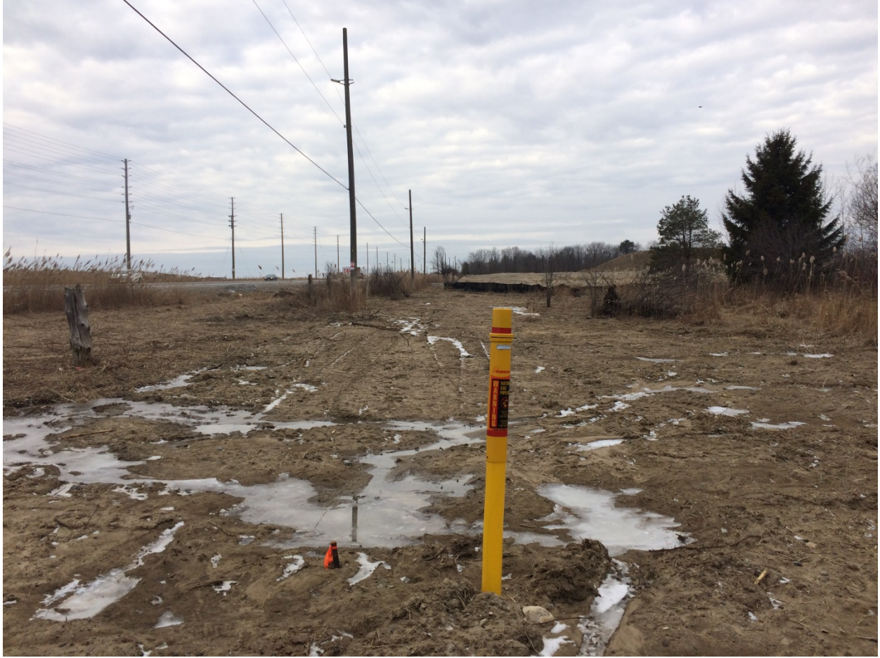
Photo 18: West of 1290 Taunton Rd (looking west)
