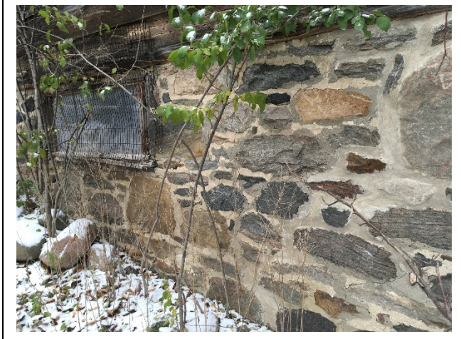
Photo 25: E13 – Exterior view of the south foundation wall
