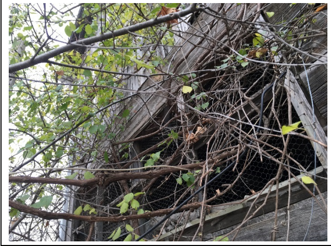
Photo 43: E22 – View of the south elevation storage opening
