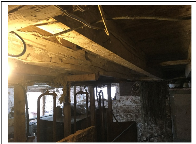
Photo 29: E15 – View of the floor joists in the basement
