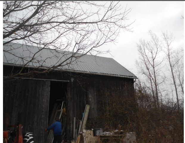
Photo 59: E30 – View of the north portion of the west elevation
