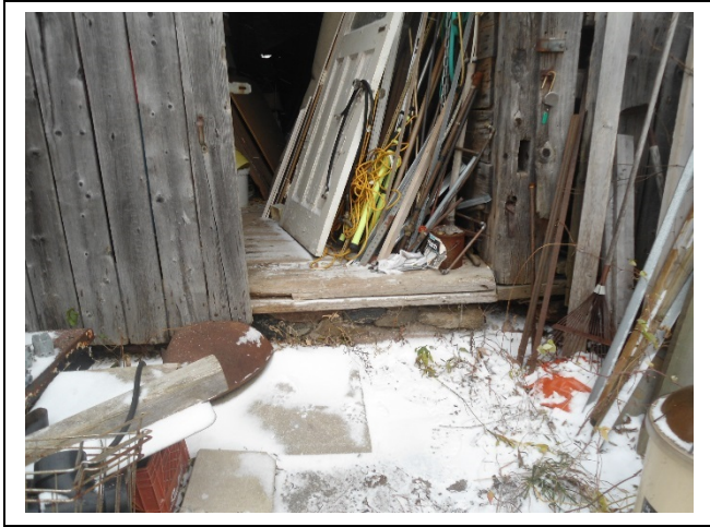
Photo 63: E32 –View of the lower portion of the sliding door
