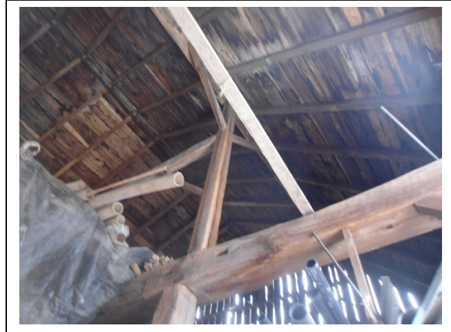
Photo 37: E19 – View of the roof wood frame structure
