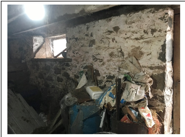
Photo 23: E12 –View of the east foundation wall towards the entrance door
