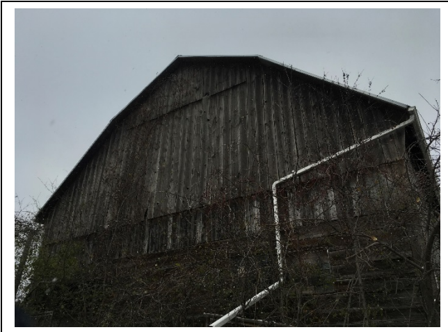
Photo 47: E24 – General view of the south elevation
