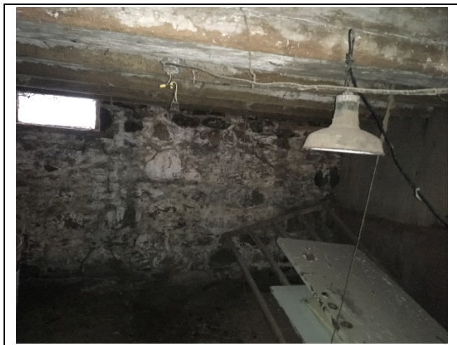
Photo 9: E5 – View of the west foundation wall.
