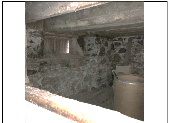
Photo 6: No significant change to the south foundation wall.
