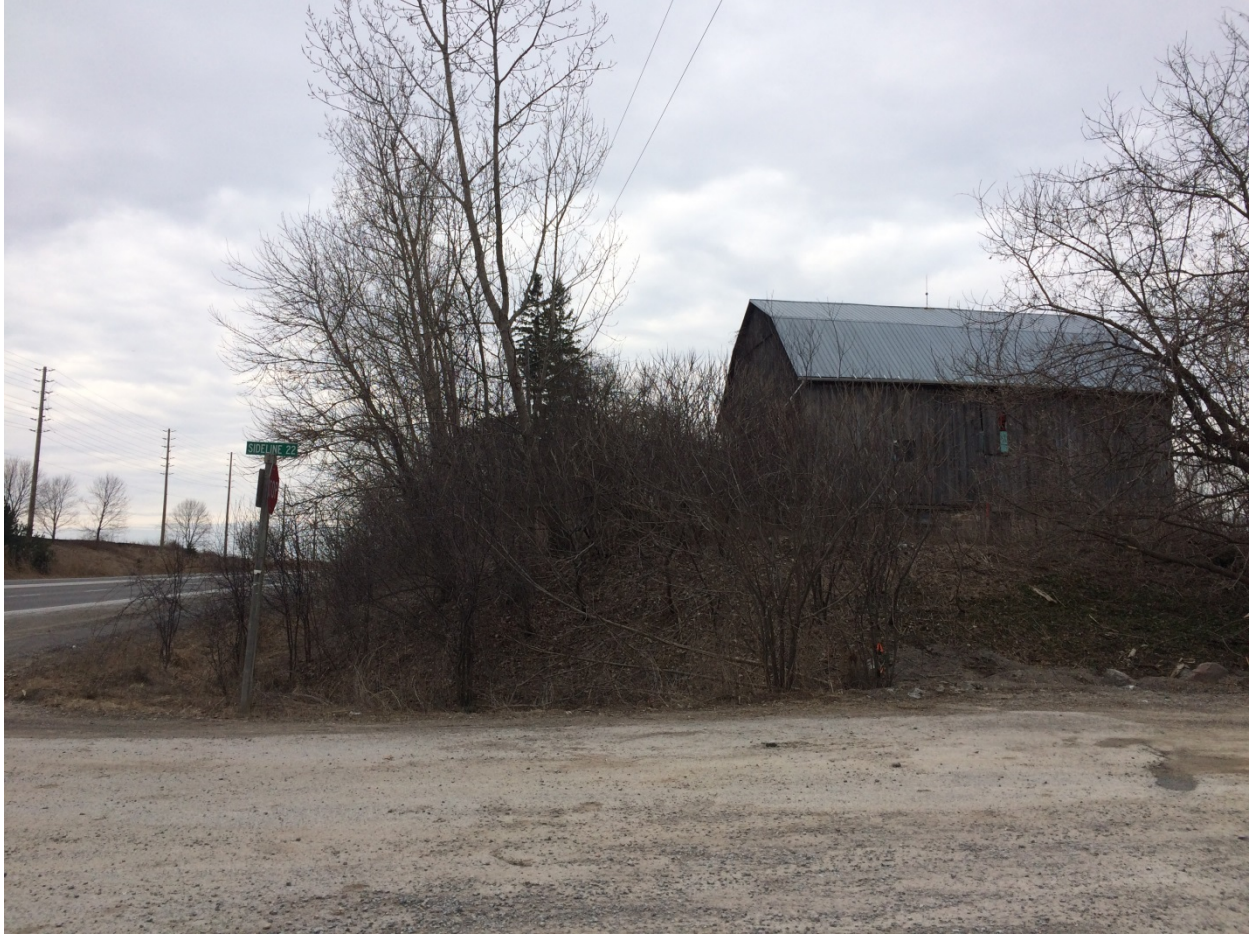
Photo 15: Heritage building at 1290 Taunton Rd (looking west)
