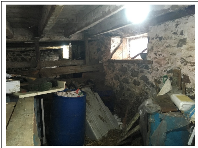
Photo 21: E11 – Another view of the east foundation wall
