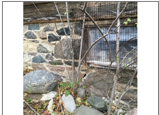
Photo 28: The observed condition is consistent with the pre-construction assessment.
