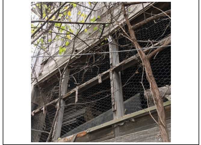
Photo 44: At the south elevation storage opening, no significant change was observed.
