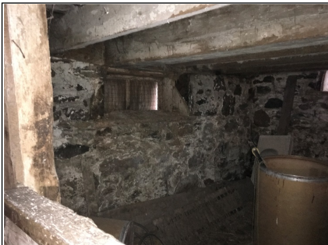
Photo 5: E3 – View of the southwest foundation wall
