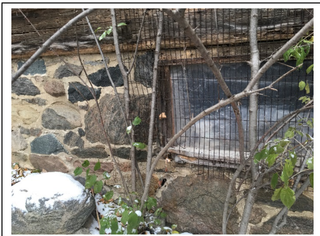
Photo 27: E14 – View of the south foundation wall around the window
