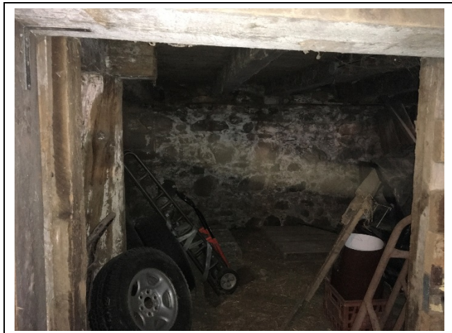
Photo 11: E6 – View of the west foundation wall
