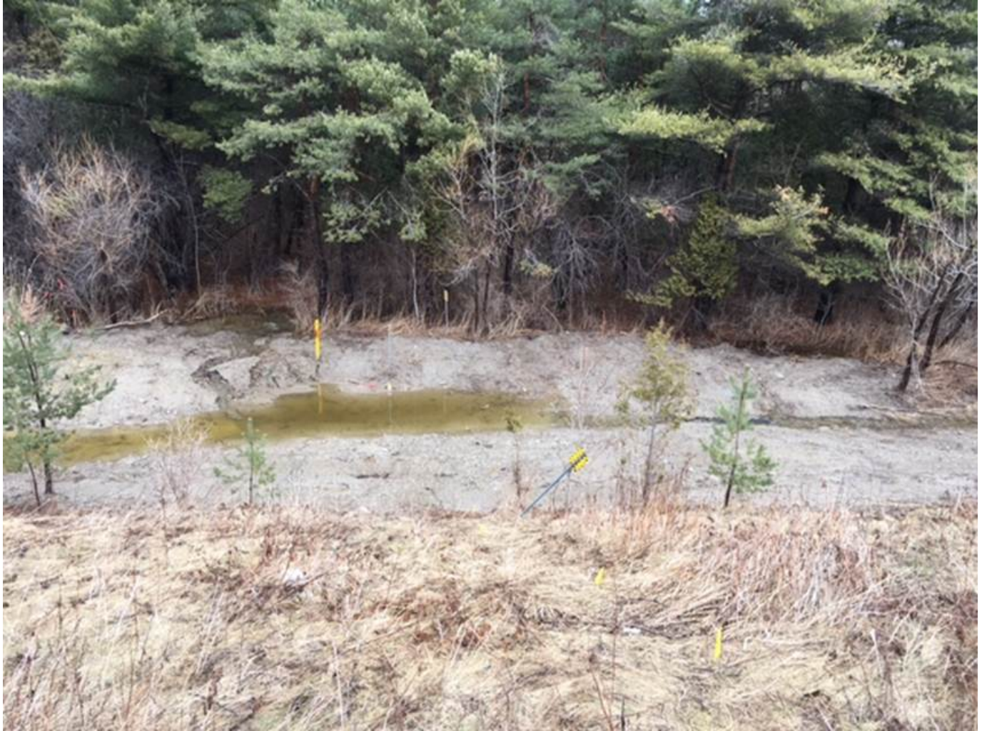
Photo 1: Taunton Rd and Sideline 16 tie-in pit (looking north)
