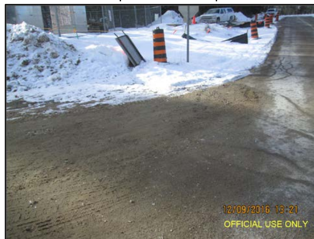
Photo 12: Looking southwest at Header Station - Downslope of silt fences shown in Photo 11 – Note that silt fences appear to need repair in Spring 2017
