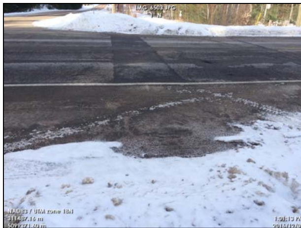
Photo 1: Paving Material replaced at Plant Rd./Baggs Rd. intersection – new material matches road grade
