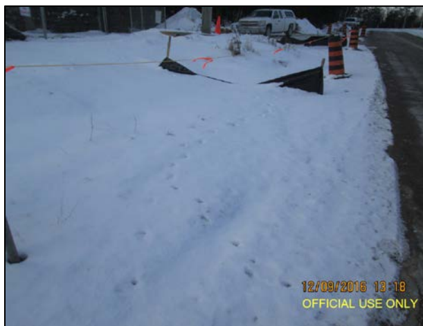
Photo 11: Looking southwest at Header Station - Silt fences in place downslope of excavation piles – Note that silt fences appear to need repair in Spring 2017
