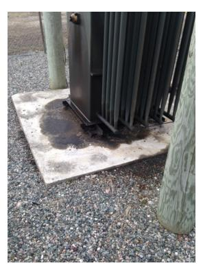
Figure 12 – Transformer leakage at Substation #1, first example
