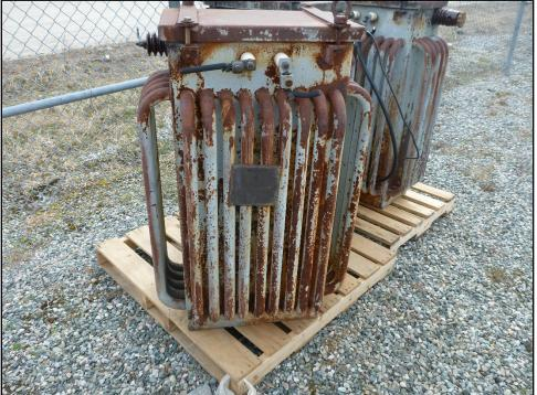
Photo 6: Three transformers from another location temporarily stored awaiting oil testing.
