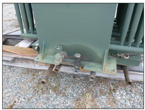
Photo 5: T1 located off the concrete pad awaiting repair. Some oily staining on side by valves.
