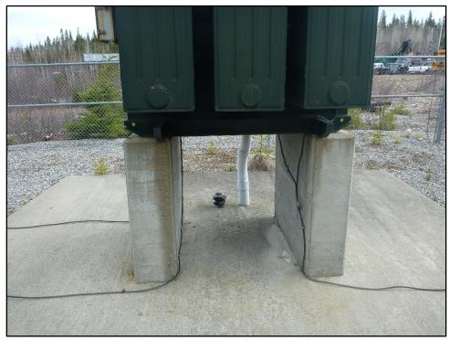
Photo 3: Photo showing the lower part of the transformer and the concrete foundation and pad.
