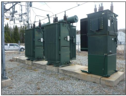
Photo 3: Photo showing the three transformers (T2, T3 and T4) on the concrete pad with no significant oil staining on concrete or gravel.
