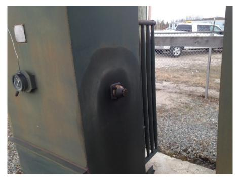
Figure 13 – Transformer leakage at Substation #1, second example
