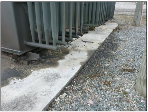
Photo 7: Oil staining on gravel surface on the north side of the concrete pad.
