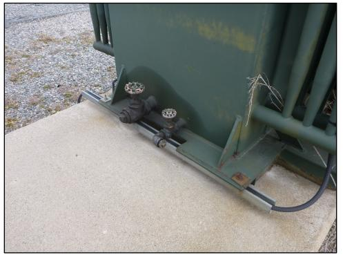
Photo 4: T3 oil staining on side of transformer by valves.
