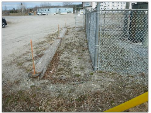
Photo 10: Retaining wall installed approximately 2 years ago to avoid pooling of rainwater run off.
