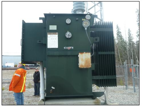
Photo 4: West side of the transformer. Wet staining around the valve.
