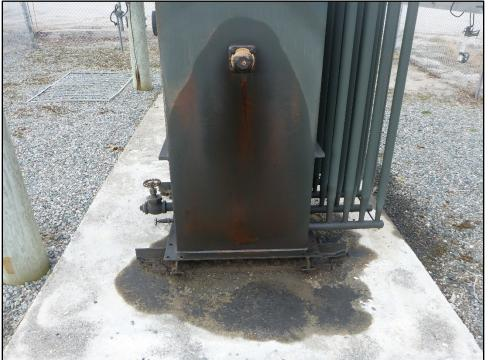
Photo 6: Leak on East side of transformer T3.
