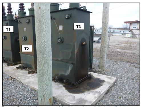
Photo 5: East side of concrete pad. Leaking gasket on "tab changer".
