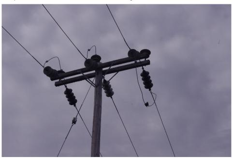
Figure 16 – Broken insulator at Substation #3
