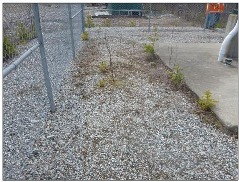
Photo 5: North side of concrete pad. Dark discolouration of the concrete does not appear oily.
