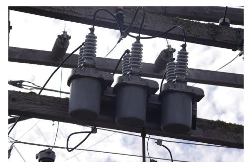
Figure 14 – Single-phase, oil-filled switch units
