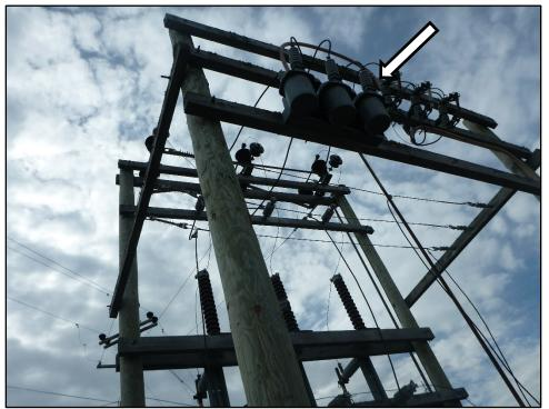
Photo 8: Three oil-filled breakers on the North side.
