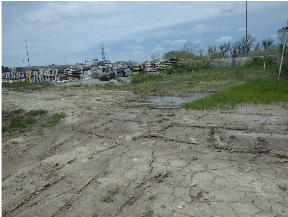
Photo 24 – Restoration required at the wetland near Beaver Creek Tributary 1 (May 2017)
