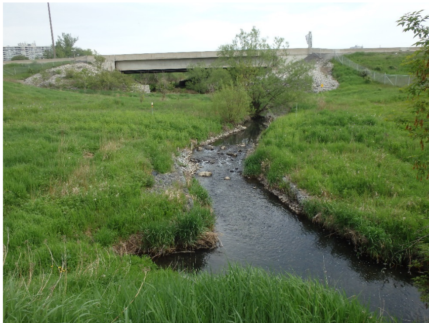
Photo 18 – German Mills Creek watercourse crossing (May 2017)
