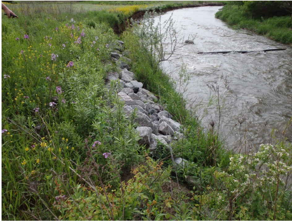
Photo 13 – Stabilization of bank at Etobicoke Creek (May 2017)
