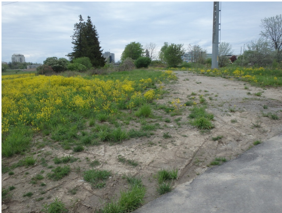
Photo 10 – Bare patches requiring some additional seeding to prevent erosion on the east side of Little German Mills Creek, Site #1B (May 2017)
