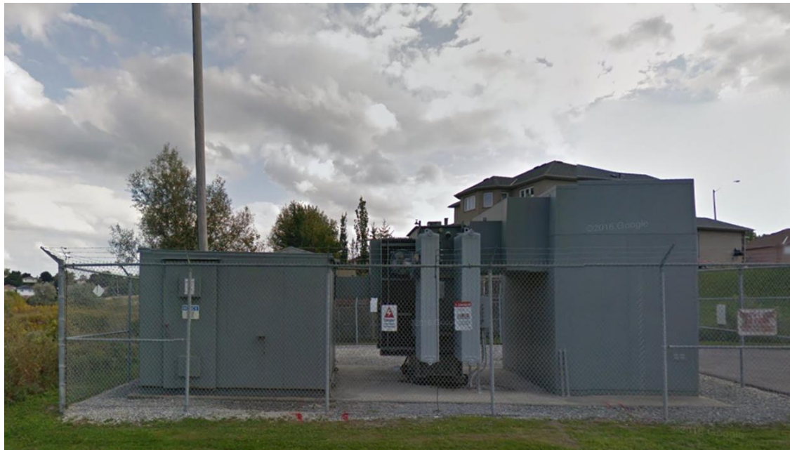
Figure 3 – Configuration of Outdoor Switchgear at MS323
