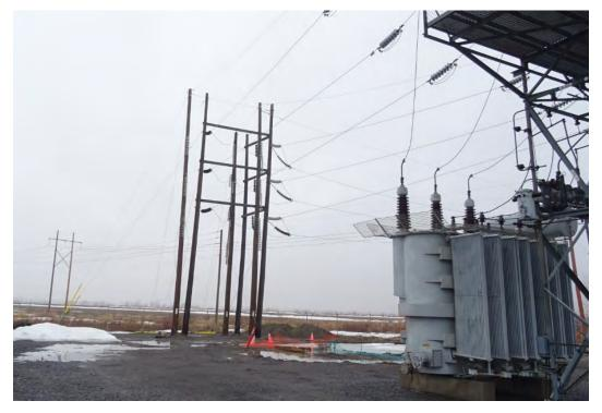
Figure 12: New 110kV Poles
