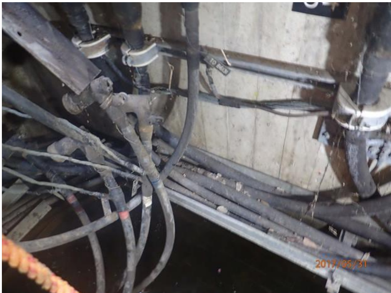
Figure 13 - Cables Laying Side-by-Side in Cable Tray
