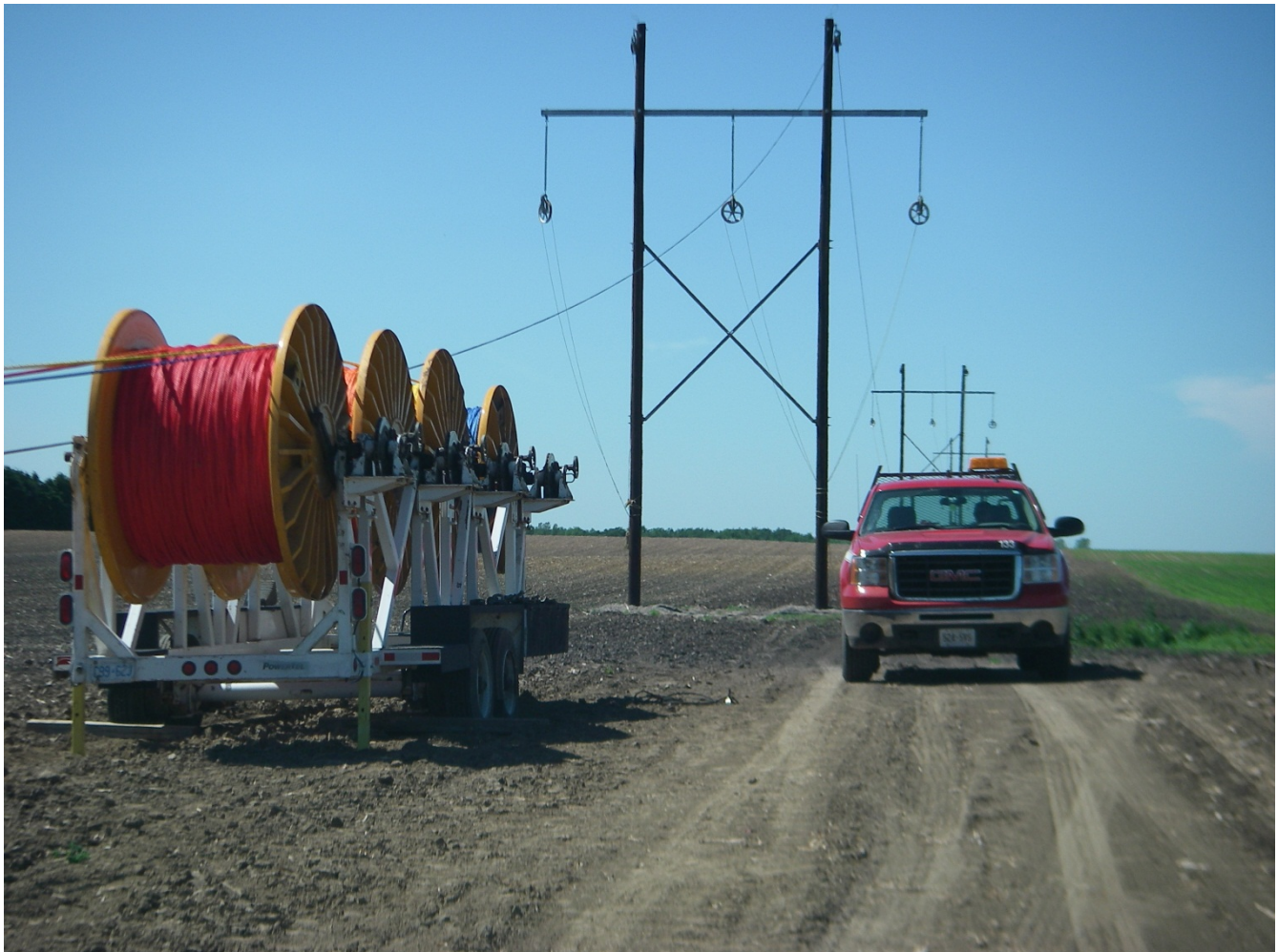
Figure 3.0-42: Illustration of Typical Conductor Installation
