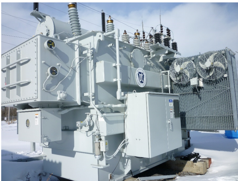
Figure 2: 110kV/12.48kV 15/20/25 MVA oil-filled transformer
