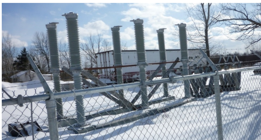
Figure 1: 115kV 3-pole circuit switcher
