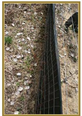
Plate 2. Example of a heavy-duty geotextile fencing used to exclude snake species (photo credit: Jeremy Rouse).
