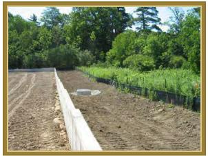
Plate 6. Stand-alone continuous concrete wall used to exclude salamander species installed as pre-cast forms (photo credit: Steven Roorda).
