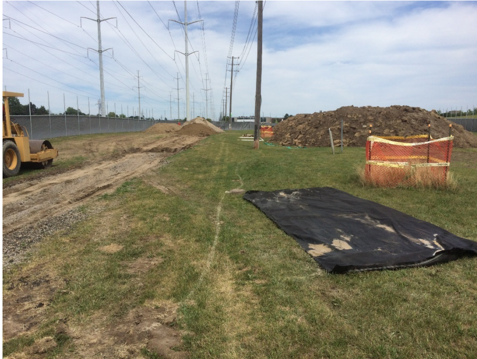
Photo 1 Location of dewatering filter bag (August 2016)
