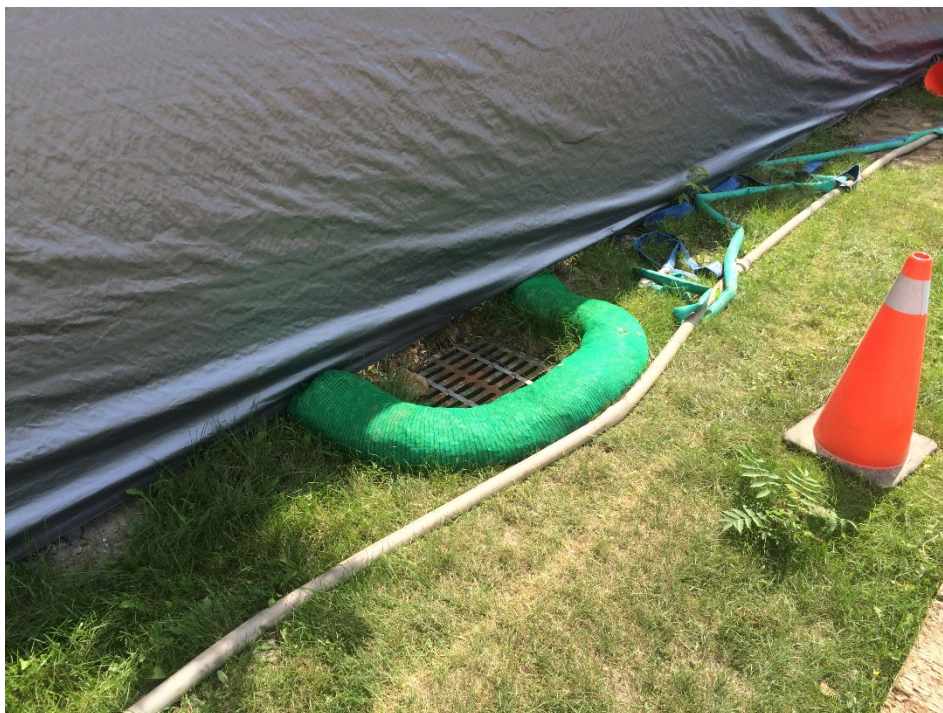
Photo 8 SiltSoxx™ surrounding storm sewer near excavation (August 2016)
