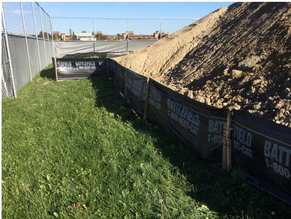
Photo 6 Sediment fencing surrounding spoil pile (October 2016).
