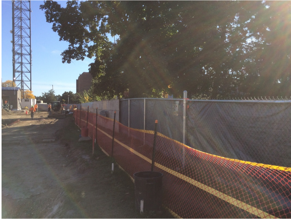
Photo 5 Tree protection zone in place (October 2016).
