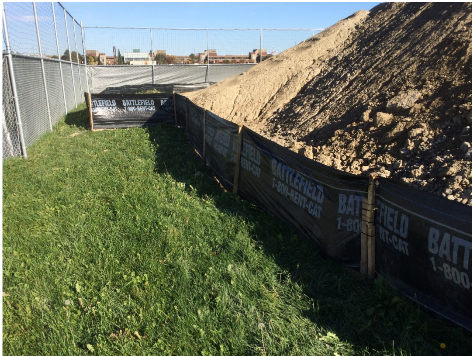
Photo 6 Sediment fencing surrounding spoil pile (October 2016).
