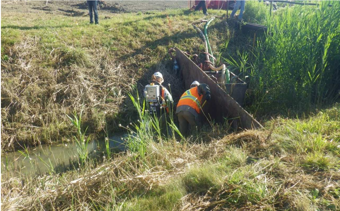
Fish rescue prior dewatering construction area as part of the typical watercourse crossing procedure.
