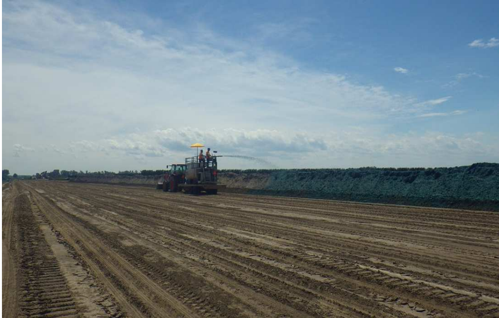
Hydro seeding of topsoil piles was completed at select location, based on topsoil type, to reduce erosion and weed growth.
