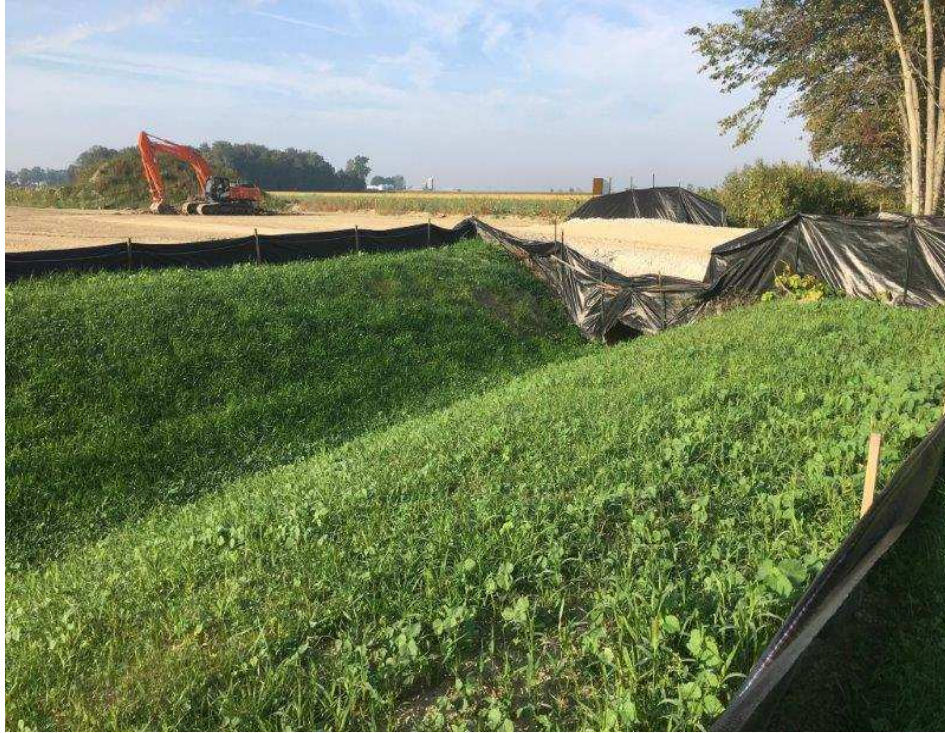
Restored Watercourse crossing following seeding establishment.
