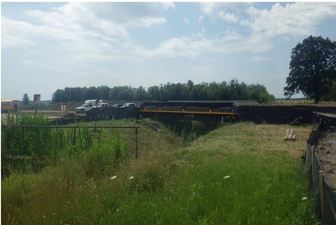
Typical temporary bridge crossing used for the Panhandle Reinforcement Pipeline Project.
