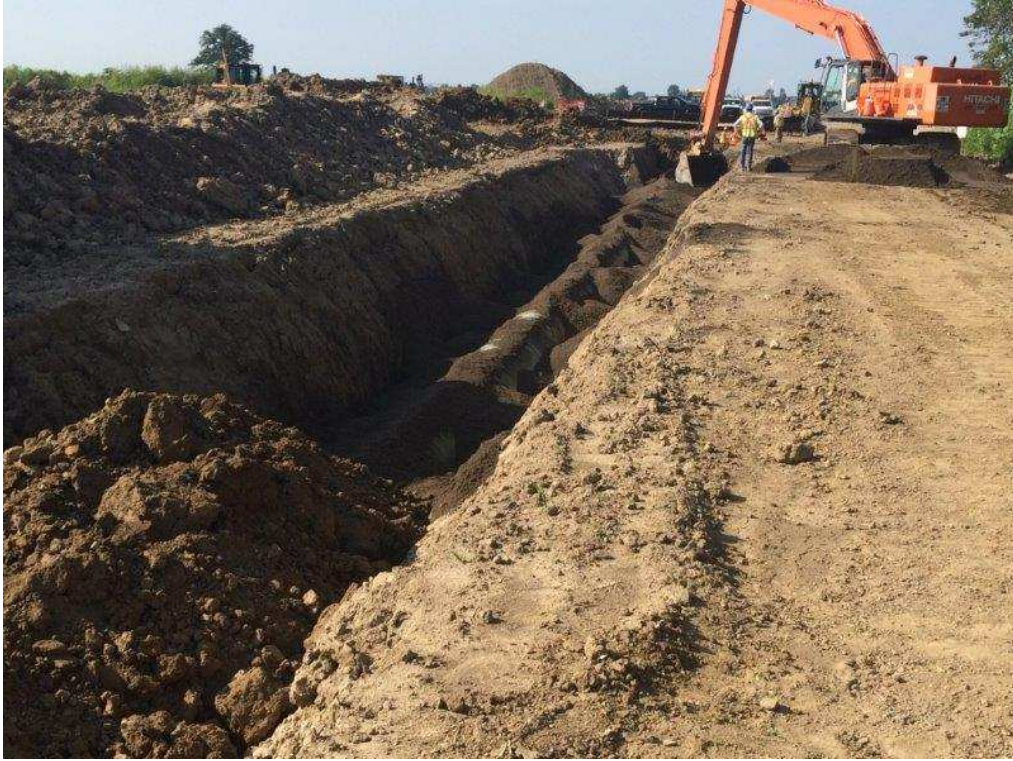
Pipe backfilling.
