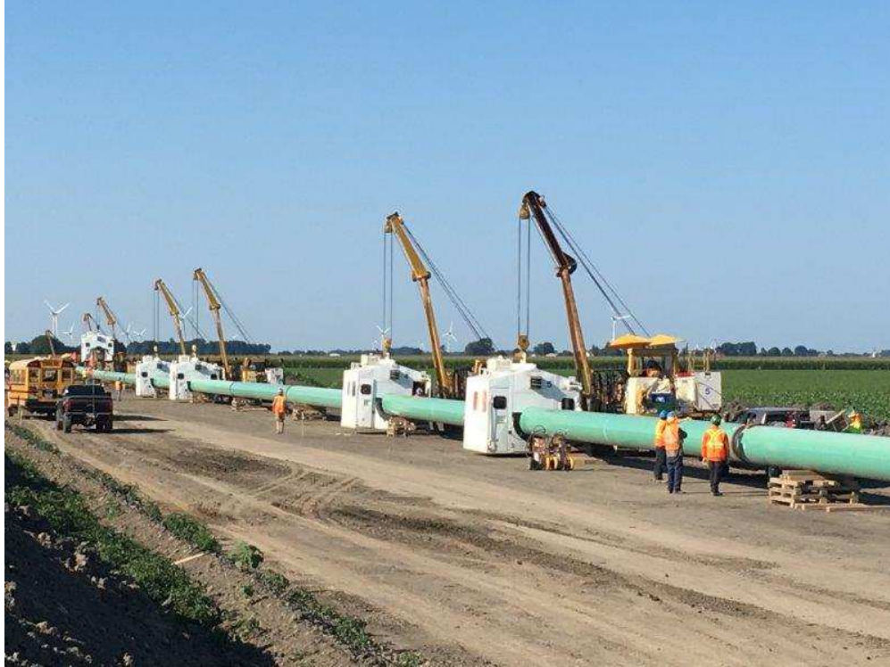
Automatic welding the pipeline joints together.
