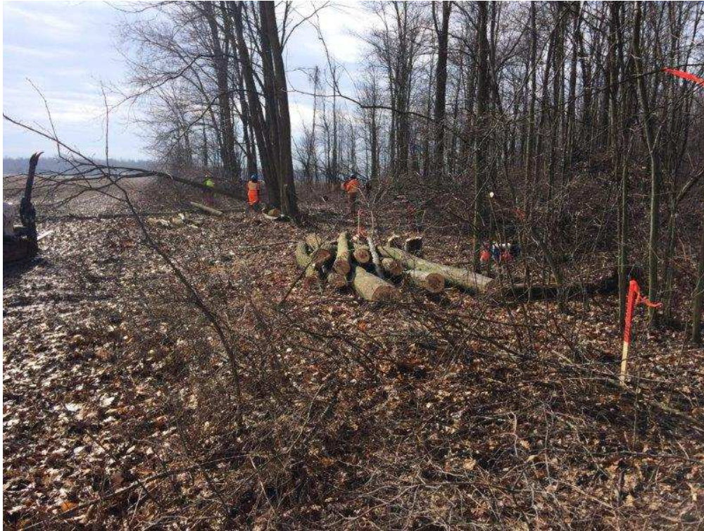
Tree clearing prior to the breeding bird window to prepare the construction easements
