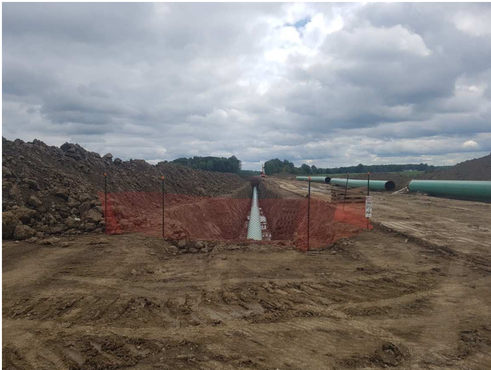
Pipeline lowered in ready for backfill, beside work area utilizing rig mats.
