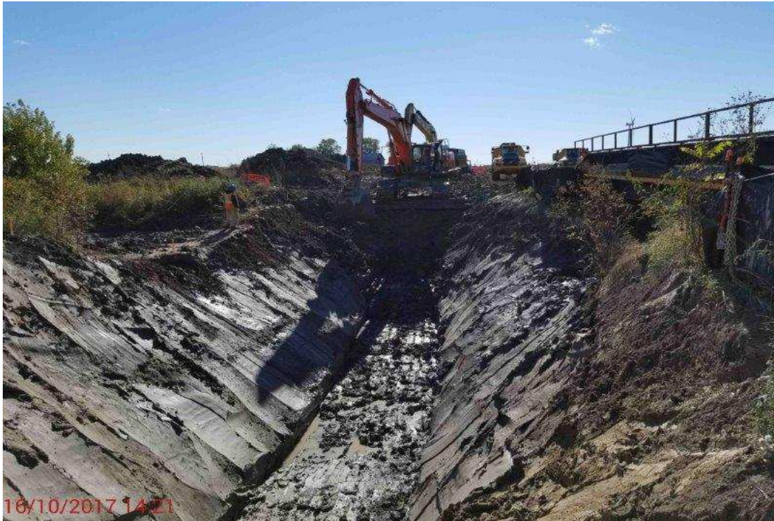
Trenching through an isolated watercourse crossing.
