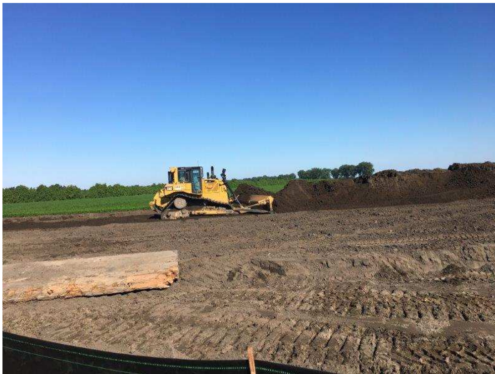
Topsoil stripping to prepare and protect the land for the construction of the pipeline.
