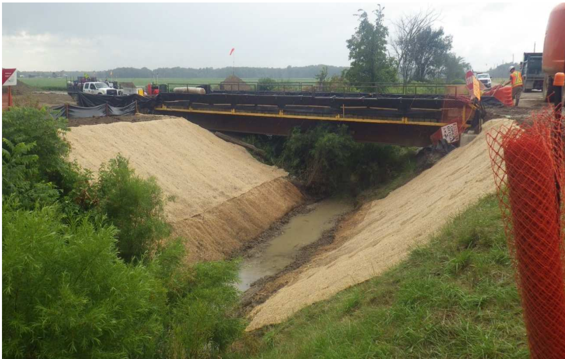
Restored watercourse crossing following pipeline installation.
