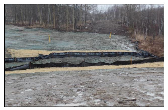
Once the pipeline is installed across a watercourse, silt fencing and erosion control matting is installed to control the migration of sediment.
