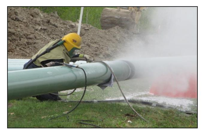
Following the stringing and welding of the pipeline, the joints are sand blasted to remove any impurities and rust. For safety, the worker must wear protective clothing and a helmet with a separate air supply.
