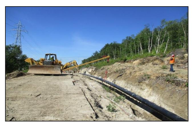
Once the section of pipeline is protected, the pipeline is lowered into the trench.
