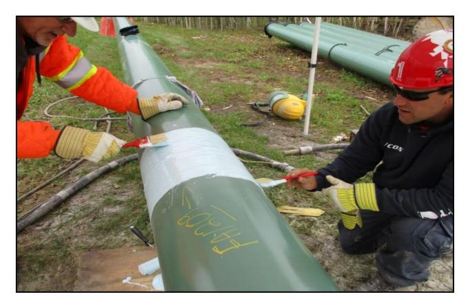
Following the sand blasting, an epoxy coating is applied to a specified thickness that will protect the joint.
