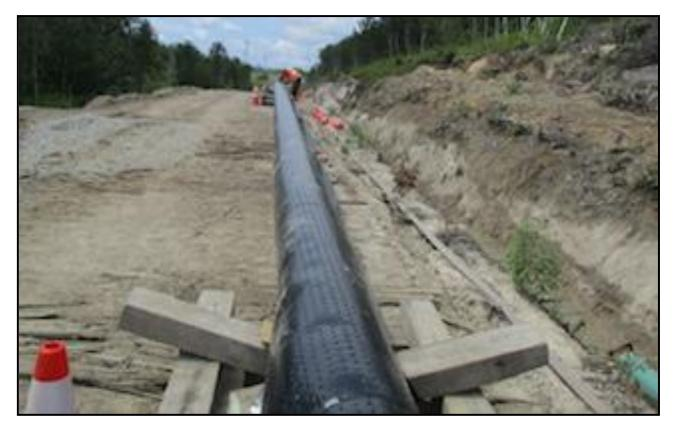
In areas where rock may have been removed to form the trench, a protective cover known as "rock shield" is wrapped around the pipe. prior to installation to protect it during backfilling,
