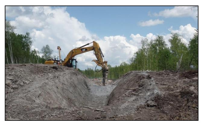
In areas of less dense or fractured rock a hoe ram attached to an excavator was used. This equipment is similar to a large jack hammer.
