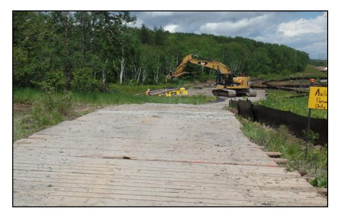
Large wooden mats were used to access remote areas preventing disturbance and rutting to the native soil leaving roots systems intact allowing for fast re-vegetation.
