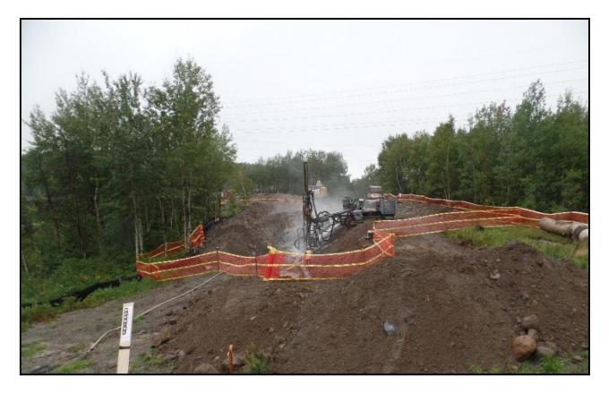
During construction some areas contained rock outcrops needed to be removed to allow for the trench. Two methods of removal where employed. In areas of dense rock, holes were drilled in the rock and blasting performed.
