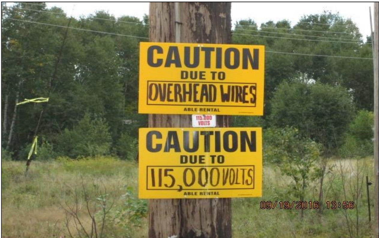
Due to the proximity of the Ontario Hydro Station, caution signs were installed along the pipeline easement
