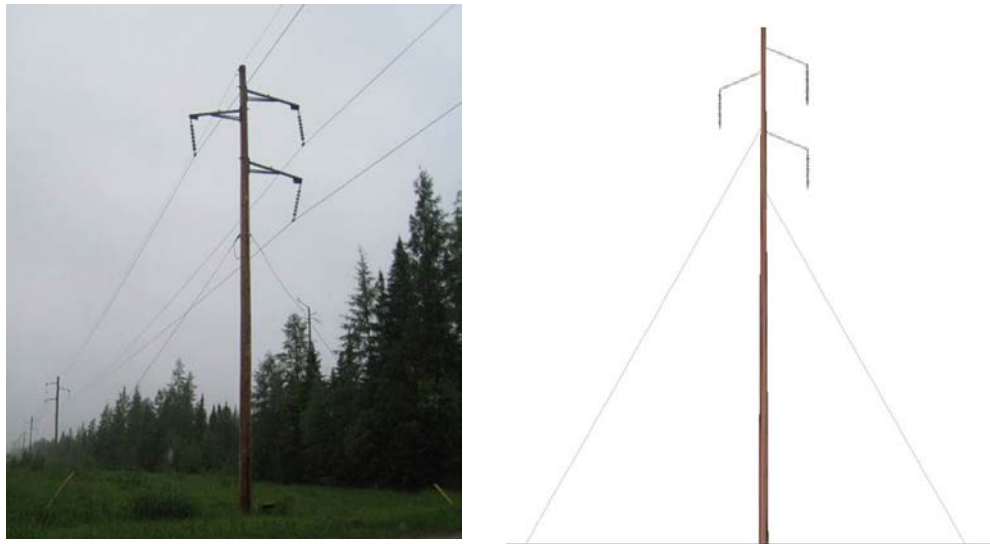
Figure 1: Picture of a single-pole suspension structure along the H9K circuit with steel harp arms adjacent to a virtual rendition of the same structure.
