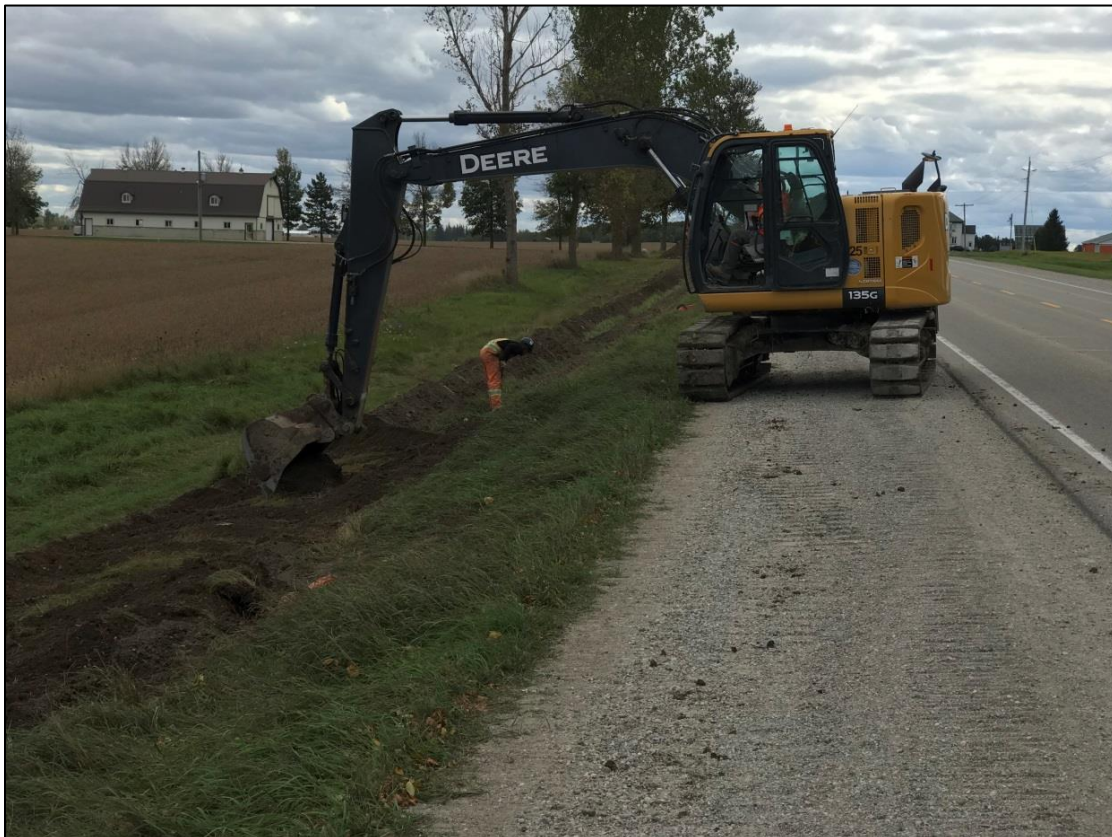
2. Backfilling the trench. Once the pipeline is lowered in, the soil is placed back in the trench if it is suitable.
