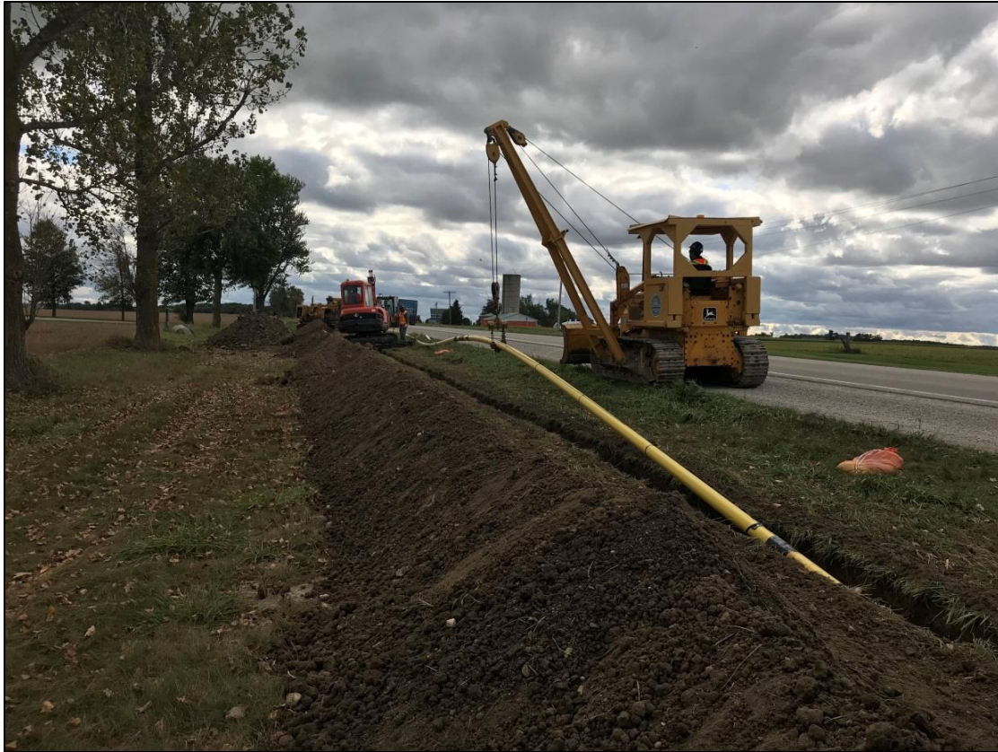
1. Lowering in the pipeline in a trenched section of the pipeline route.
