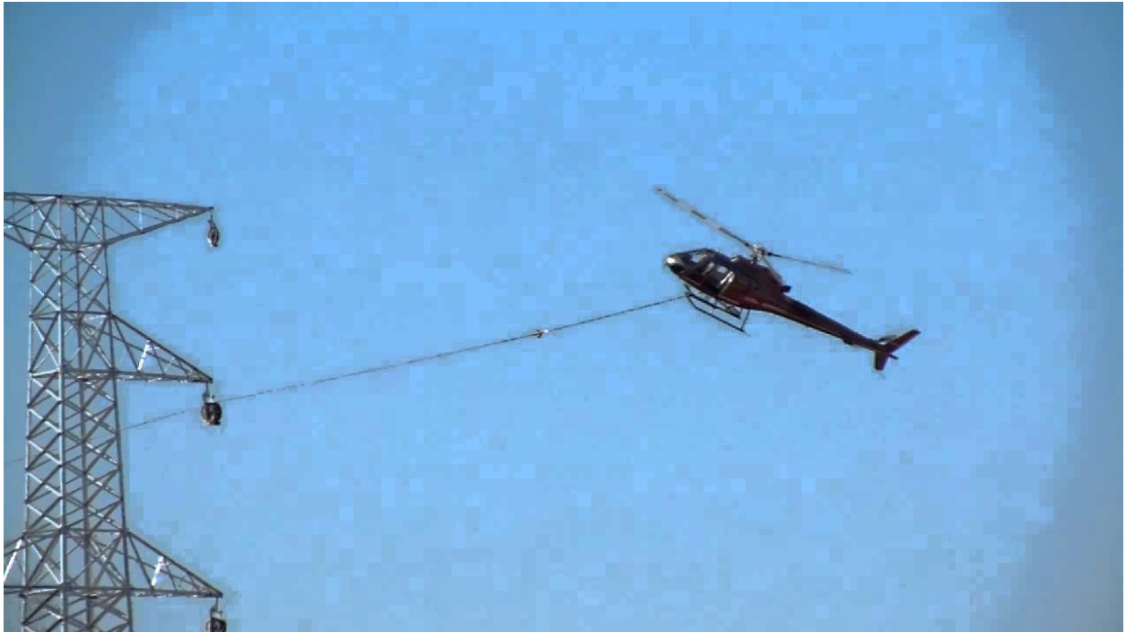
Figure 2-4 Helicopter Installation of Pilot Wire for Stringing Operations
