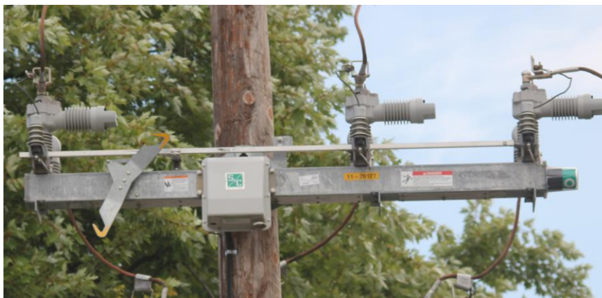
Figure 5: SCADA-Mate Switch
