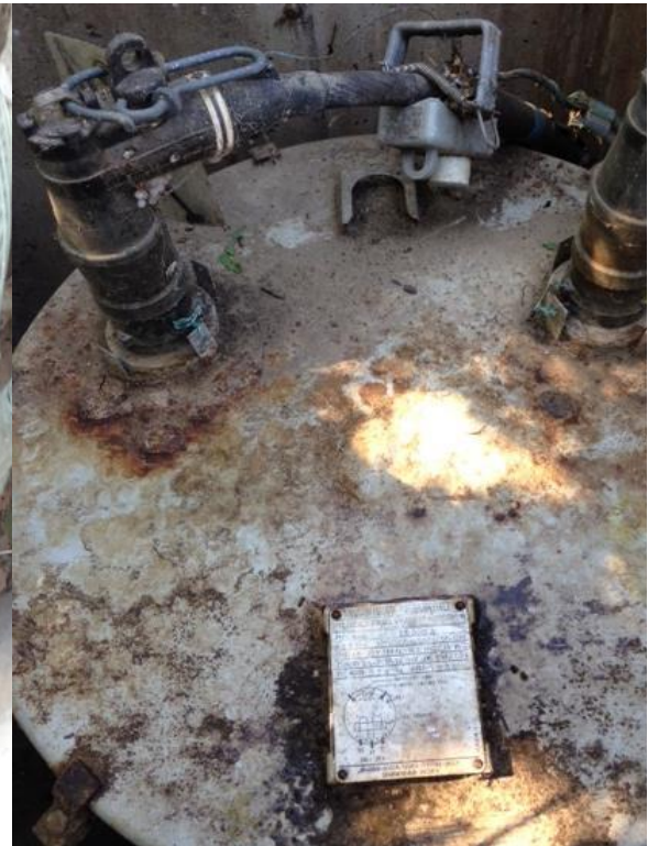
Figure 7: Corrosion on Top of a Transformer
