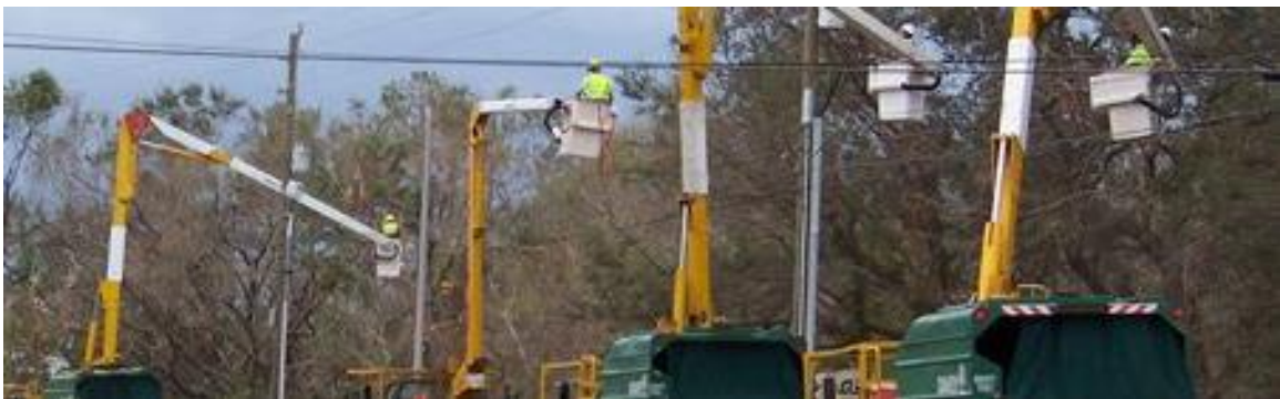
Figure 12: Tree Trimming of an Overhead Feeder
