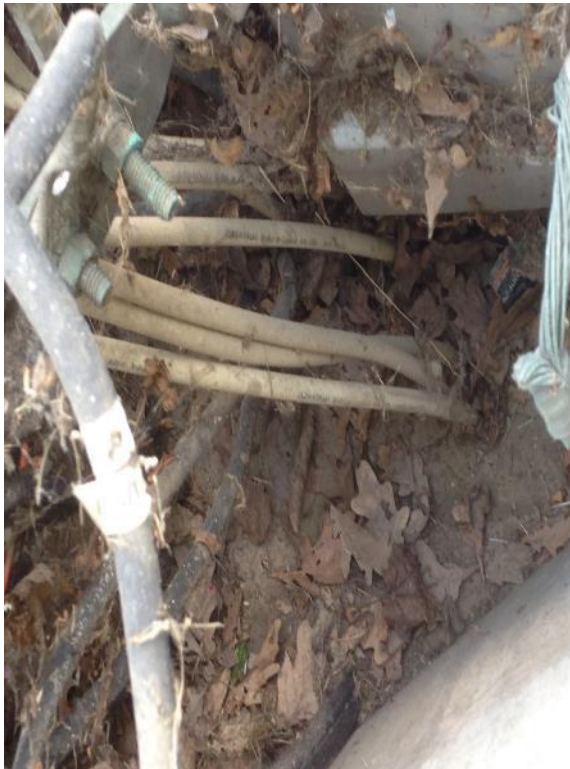
Figure 6: Vault Full of Dirt and Debris
