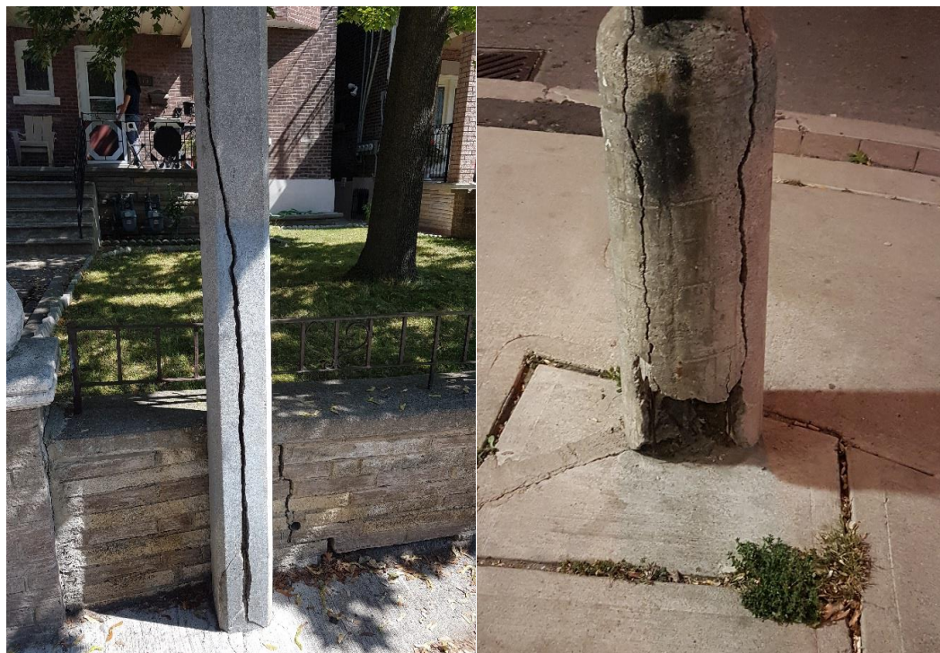
14 Figure 4: (Left) Longitudinal Crack on Pole, (Right) Cracked Concrete Base
