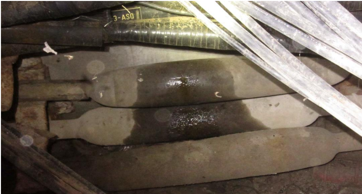
Figure 18: Oil Leakage from Cable Lead Splice
