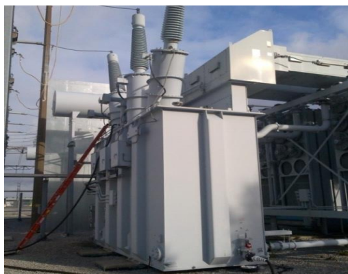
Figure 20: Power Transformer at Cavanagh TS
