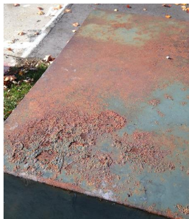
Figure 15: Padmounted Transformer with Surface Corrosion
