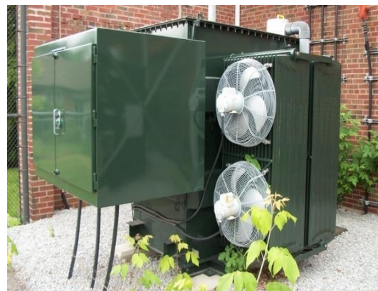
Figure 21: Power Transformer at Neilson Dr. MS
