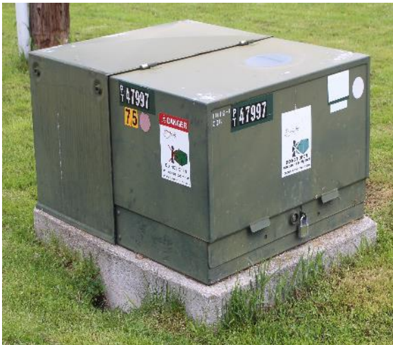
Figure 11: Padmounted Transformer
