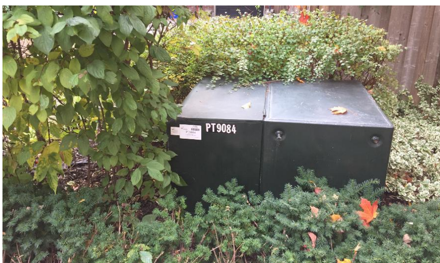
Figure 17: Padmounted Transformer Requiring Vegetation Removal
