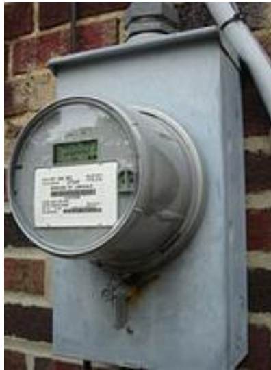
Figure 14: Smart Meter installation at Customer Location.
