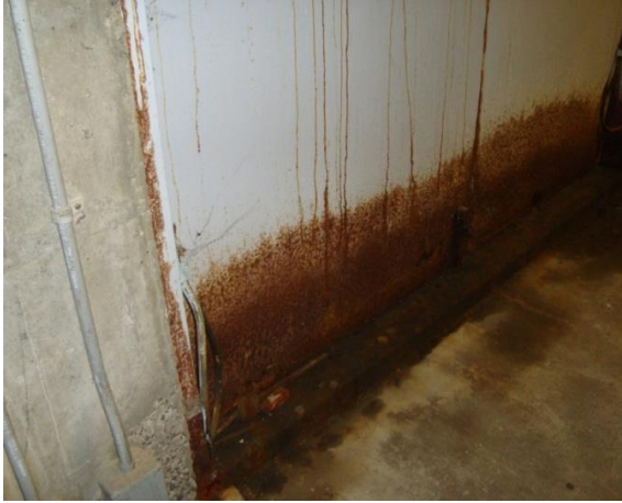
Figure 15: Rusty Switchgear Enclosure
