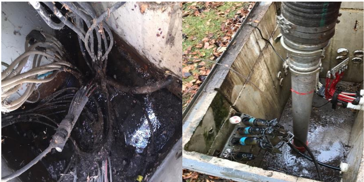
Figure 8: Oil Leaking from a Transformer Base Inside a vault
