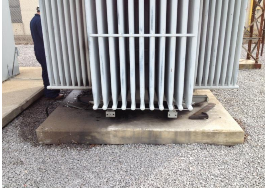
4 Figure 11: Oil Leak on a Station Transformer
