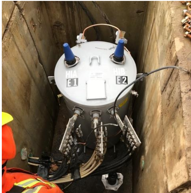
Figure 2: Submersible Vault
