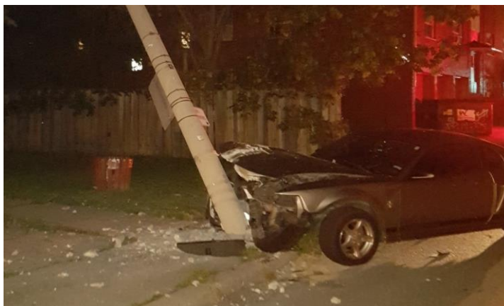
Figure 8: Distribution Poles Damaged by Vehicle Impacts
