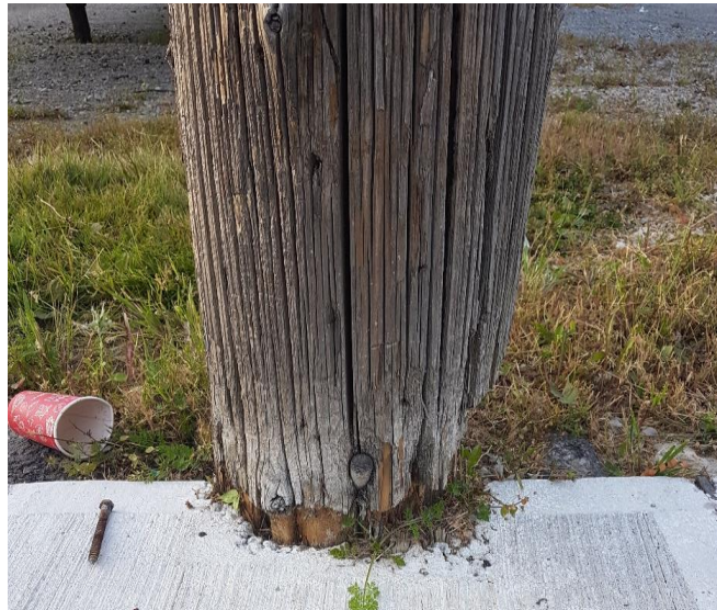
Figure 2: Rot at Base of a Pole
