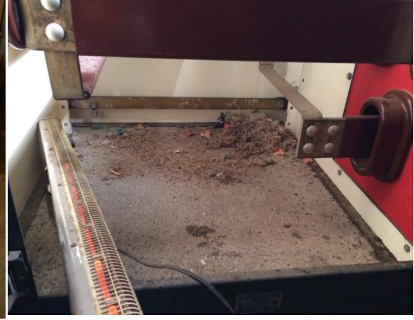
Figure 16: Pests Inside Outdoor Switchgear
