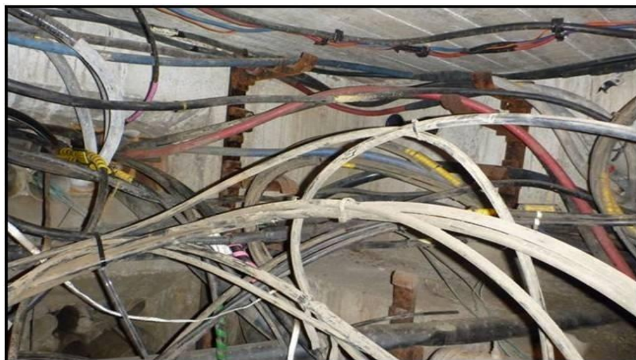
Figure 8: Underground Cable Chamber in Toronto Hydro's System.
