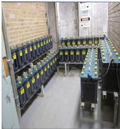
Figure 9: Station Battery System at George and Duke MS
