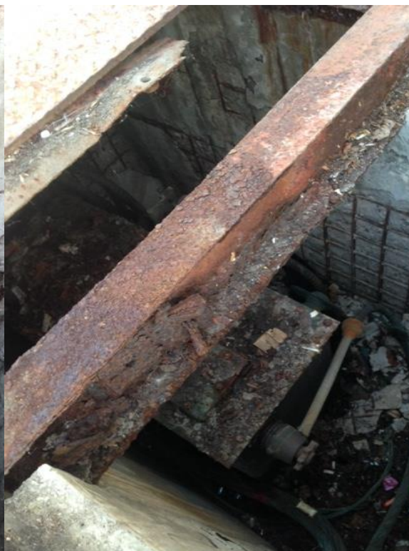
Figure 4: Corroded I-Beams
