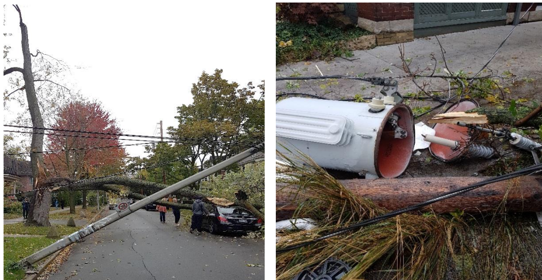
4 Figure 4: Fallen Tree on Oower Lines from High Wind Event on October 15th, 2017
