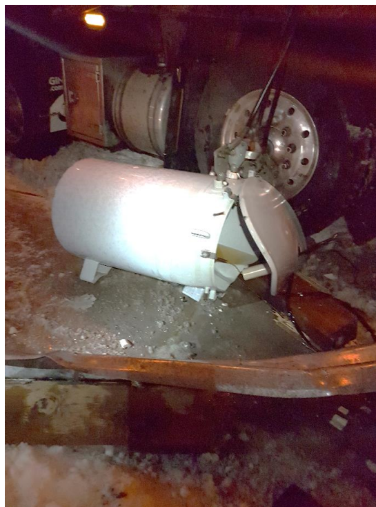
Figure 9: Distribution Transformer Leaking Oil After Vehicle Impact with Pole
