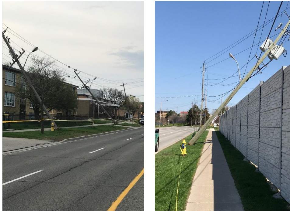
Figure 6: Examples of Wind Damage Recent 2018 Storm
