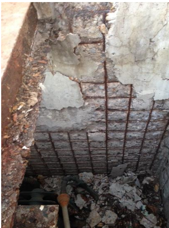
Figure 3: Crumbling Vault Roof with Exposed Rebar
