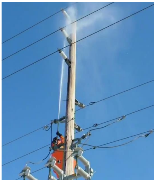
16 Figure 7: Porcelain Insulator Washed Using a High Pressure Water Jet
