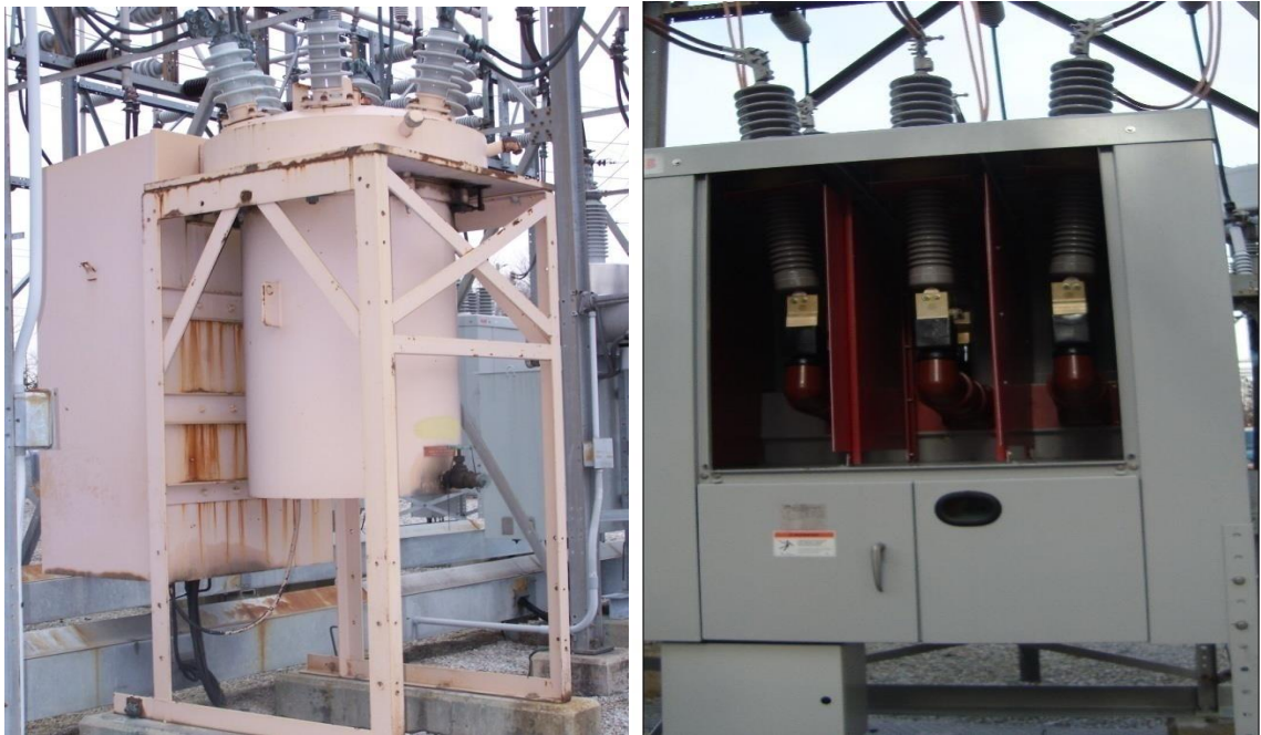
Figure 14: (Left) KSO Oil Circuit Breaker, (Right) Vacuum Circuit Breaker
