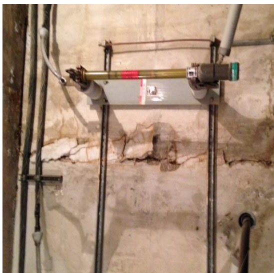
Figure 4: Cracked Walls
