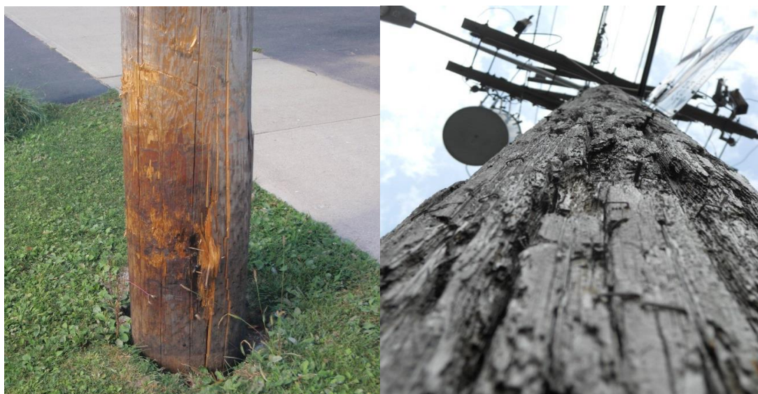
Figure 3: (Left) Cracked Wood Pole, (Right) Surface Rot on Pole
