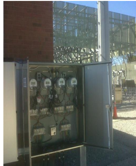
Figure 15: Wholesale Meter Installation at Transformer Station.
