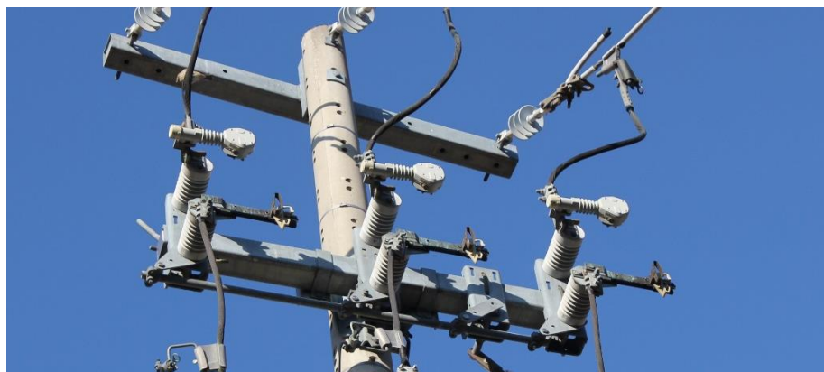
Figure 6: Manual Gang-Operated Switch
