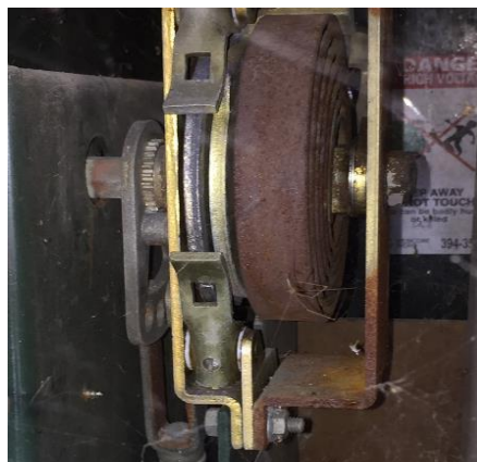
Figure 16: Padmounted Switch with Rusted Coil Spring
