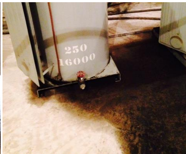
Figure 3: Transformer Leaking Oil
