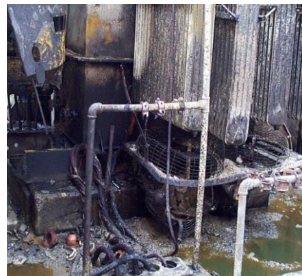
Figure 25: Leaking Fluids from Failed Transformer
