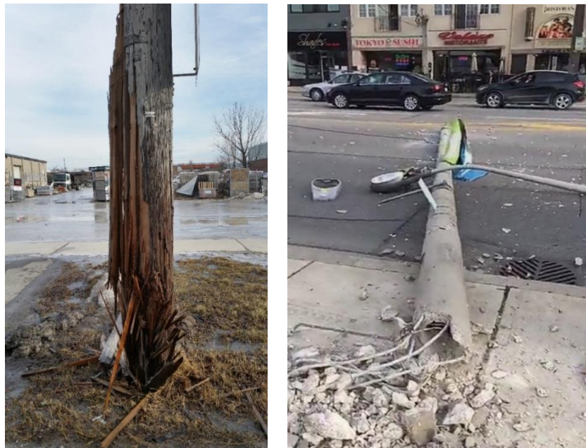
8 Figure 7: Distribution Poles Damaged by Vehicle Impacts
