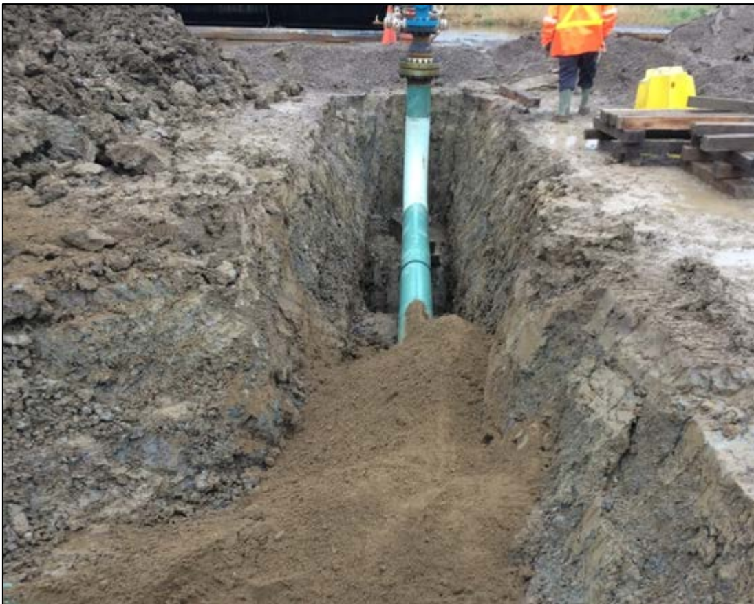
6. Backfilling the trench with sand prior to backfilling with original soil.
