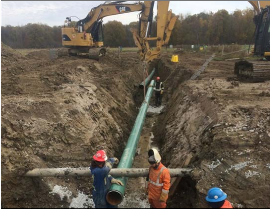
5. Lowering-in a section of pipe to connect a new well to the gathering system.
