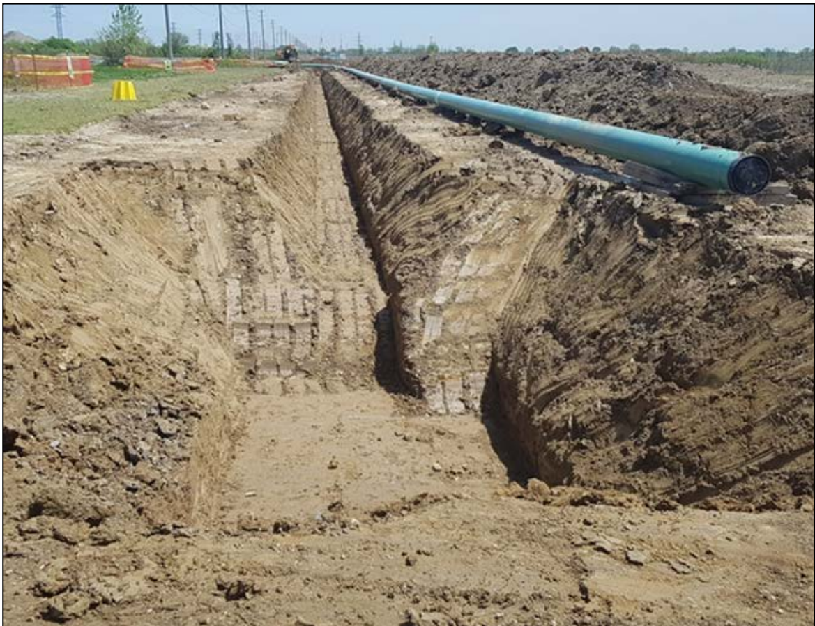
4. The pipe is strung next to the trench prior to lowering-in.
