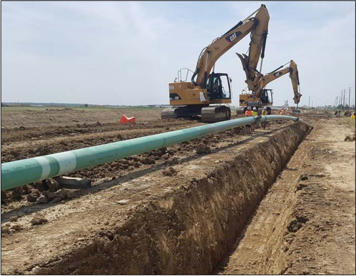
5. Lowering-in of the welded pipe in progress.
