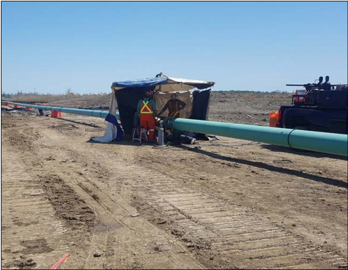
3. Pipe sections are strung out on supports and welded together.
