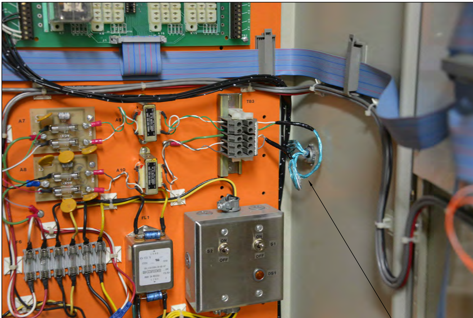
COPPER COMMUNICATION LINES WITHOUT ELECTRICAL ISOLATION
