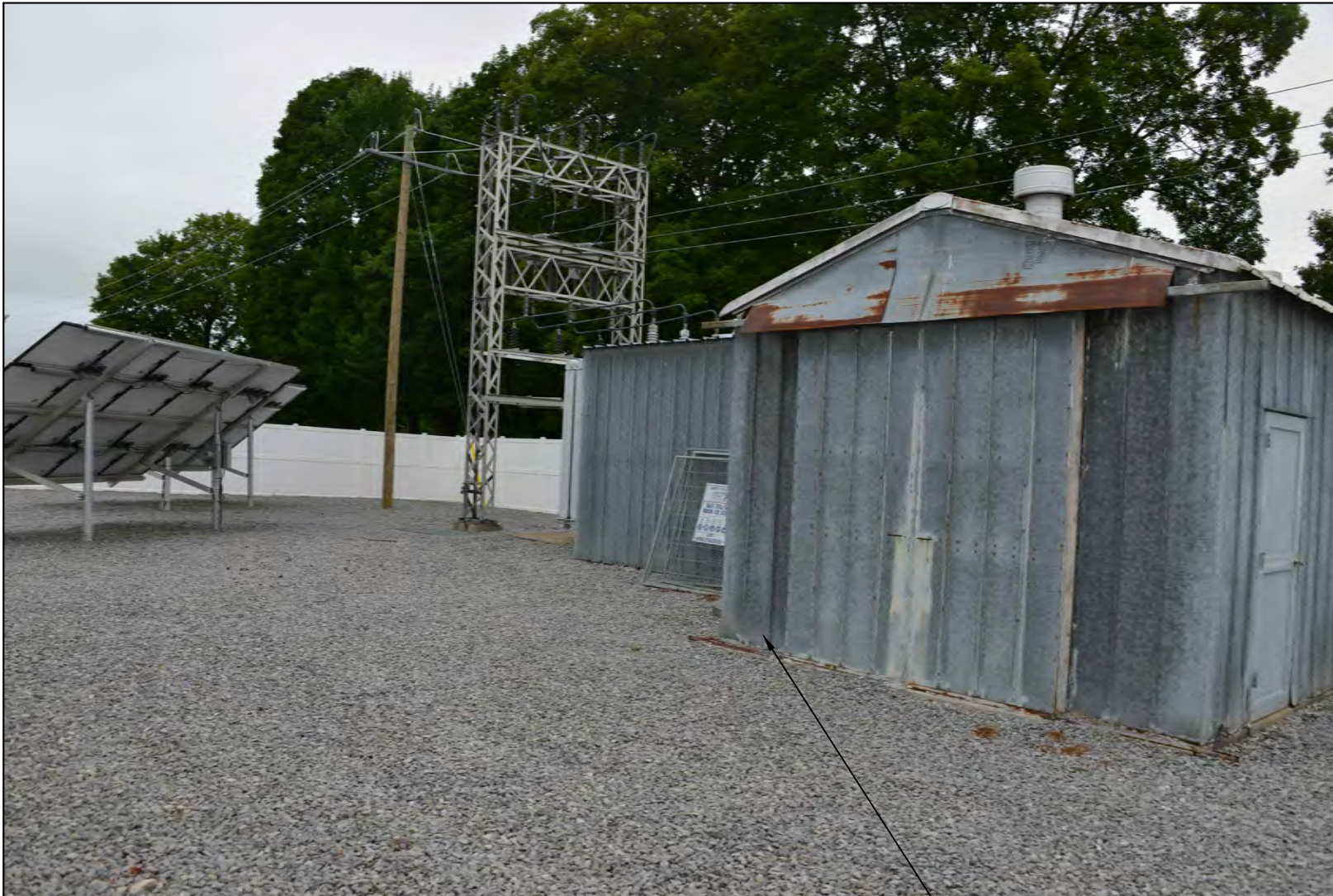
IMPROPER GROUNDING AND BONDING ON METAL CLAD SWITCHGEAR BUILDINGS
