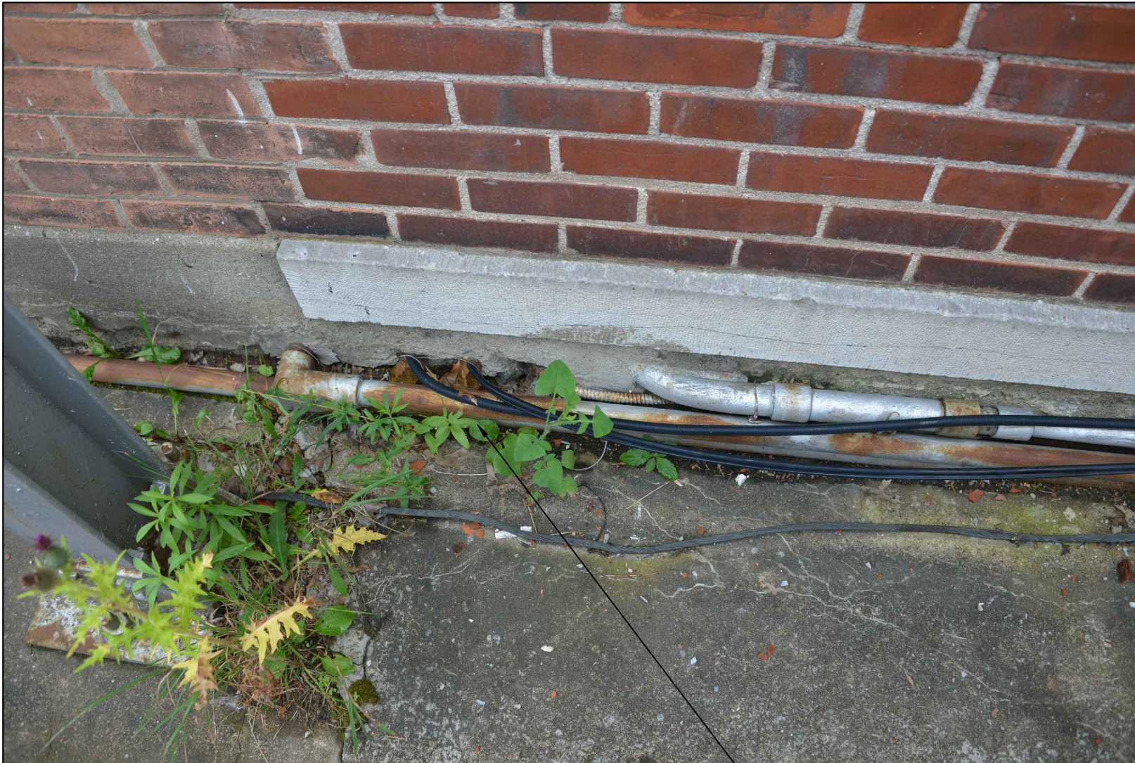
IMPROPER INSTALLATION OF CONTROL CABLES – NOT TO CODE
