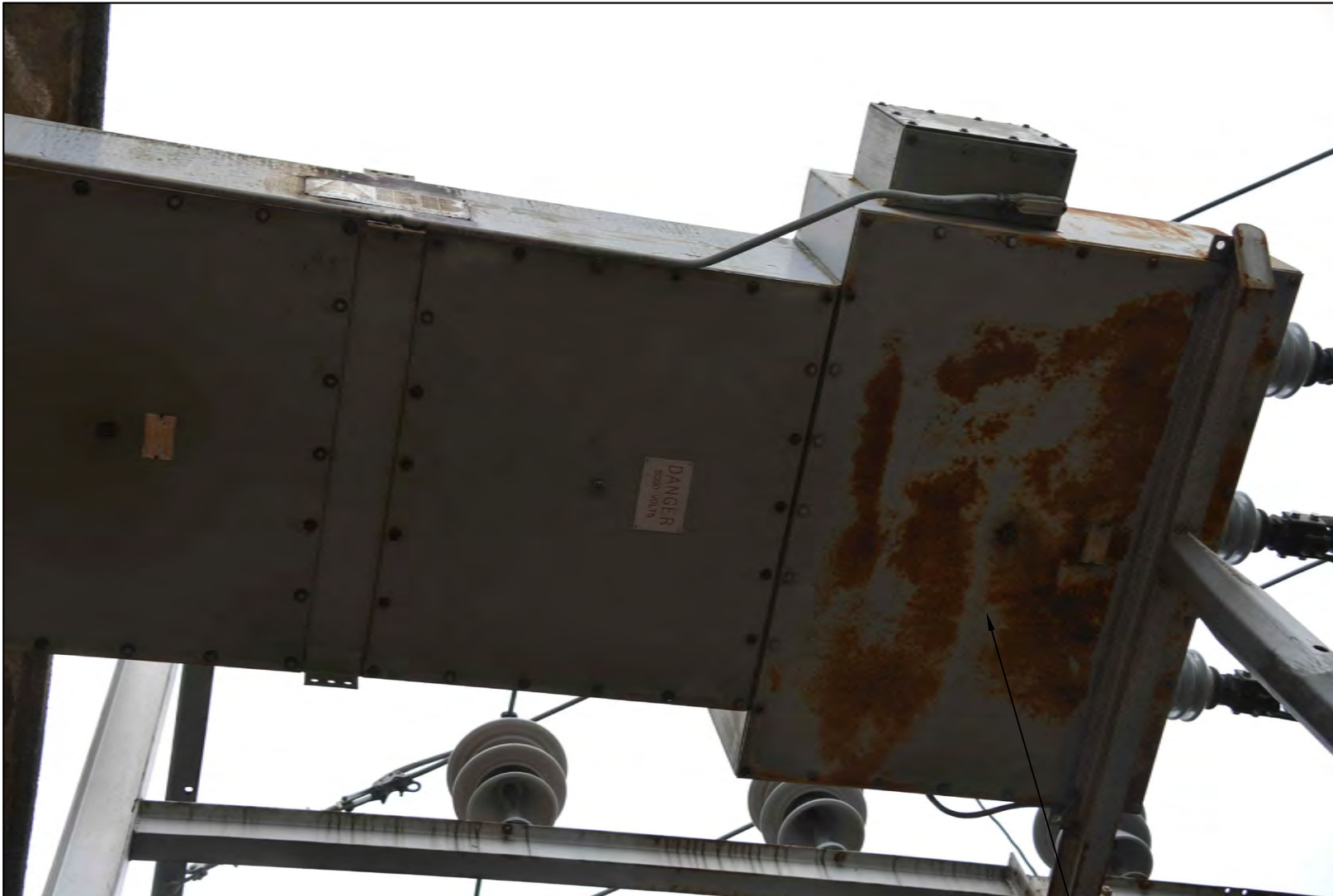
PAINT CONDITION ON BUS DUCT
