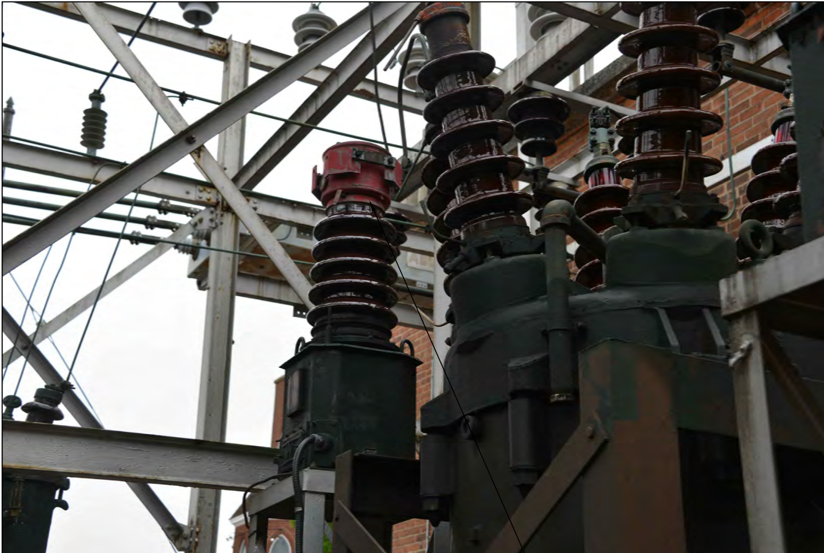
PORCELAIN INSTRUMENT TRANSFORMERS – VERY LOW CLEARANCES FOR WORKERS
