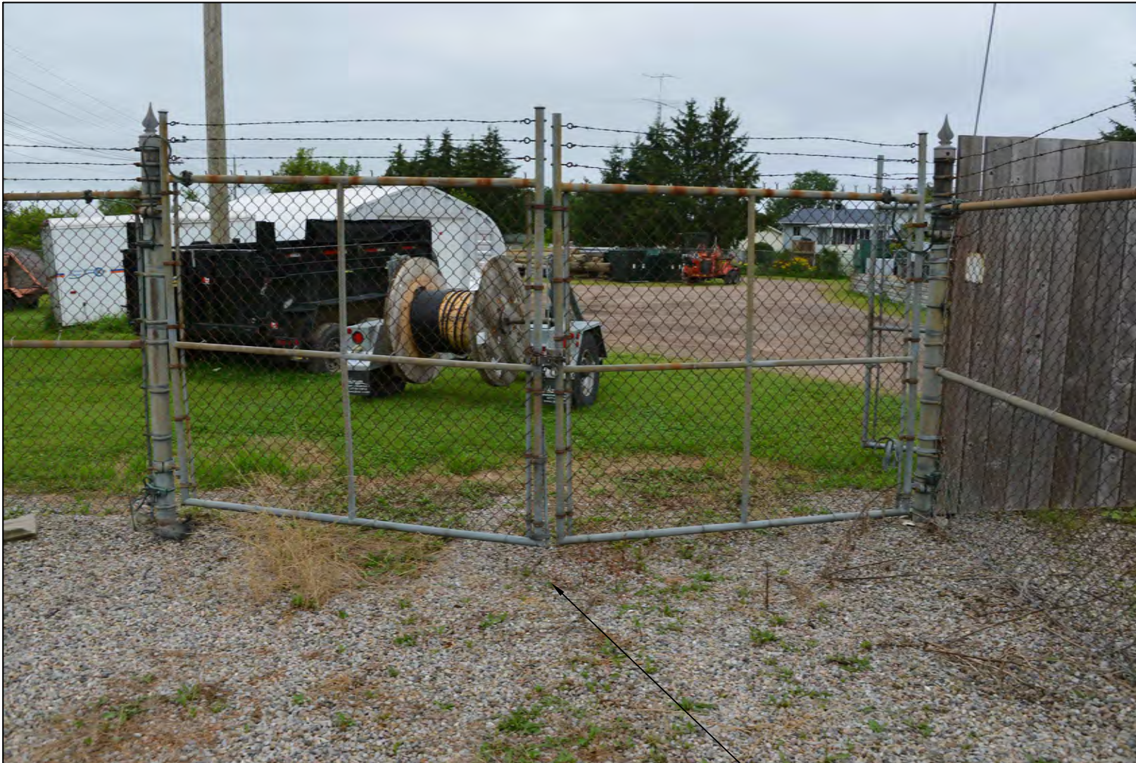
FENCE GATE SWINGS OUTSIDE OF THE STATION GROUND GRID
