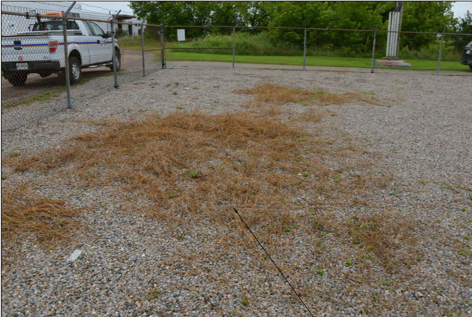
INADEQUATE CRUSHED STONE WITH VEGETATION GROWING THROUGH IT
