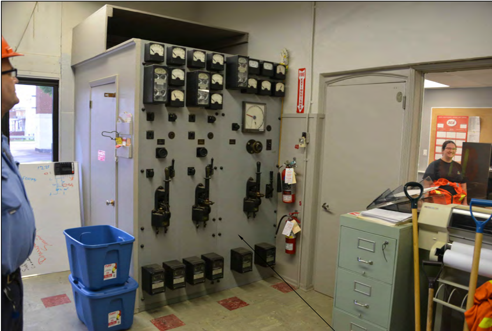
MINI OCB'S COMBUSTIBLE IN OFFICE ENVIRONMENT
