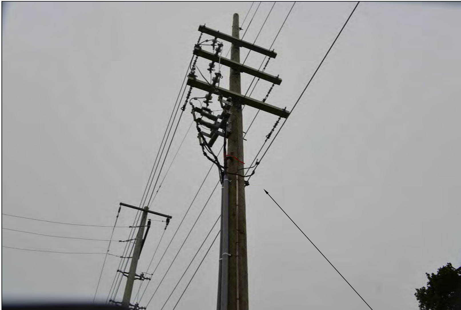
STATION L.V NEUTRAL CONNECTION IS BARE 3/0 WIRE
