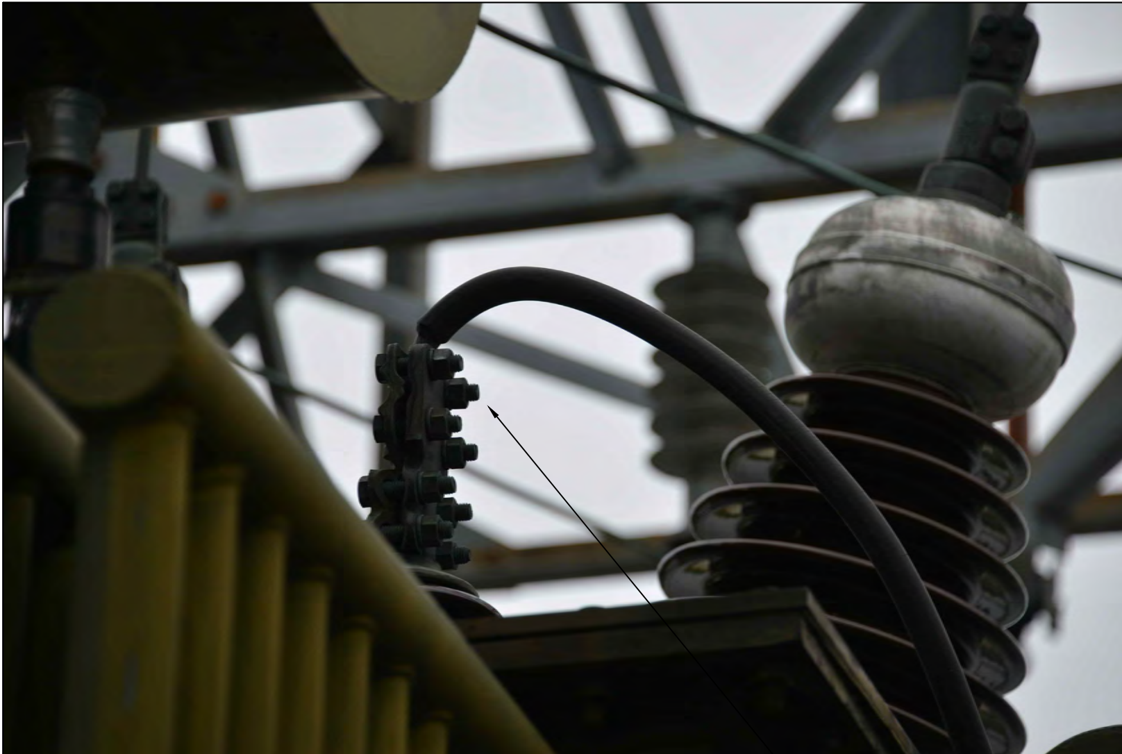
TRANSFORMER LV NEUTRAL NOT MECHANICALLY PROTECTED
