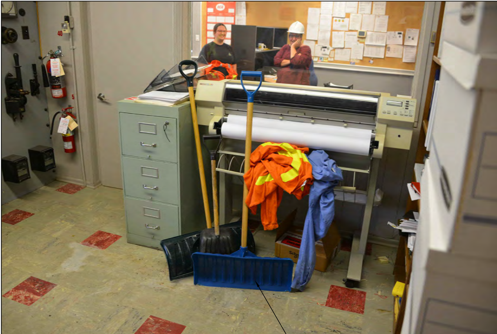
OFFICE EQUIPMENT AND STORAGE IN THE SUBSTATION ROOM – CODE VIOLATION. OFFICE ATTACHED TO SUBSTATION (GLASS).
