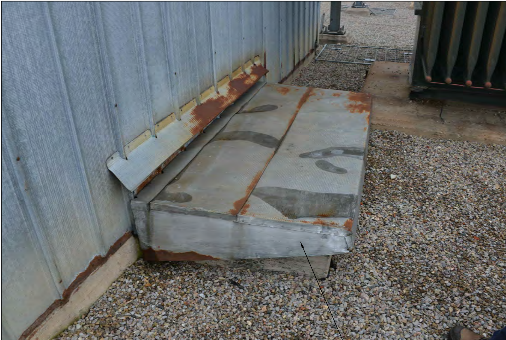
GROUNDING AND BONDING OF VAULT LID
