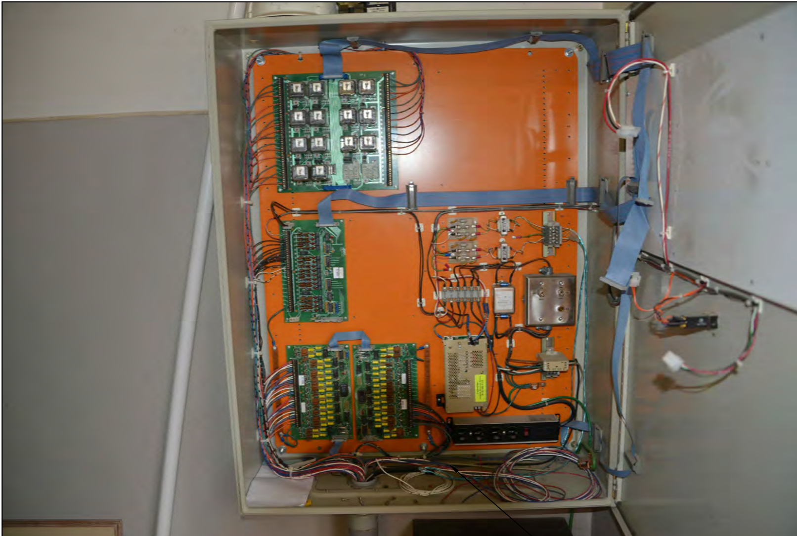
— FAILED SCADA RTU
