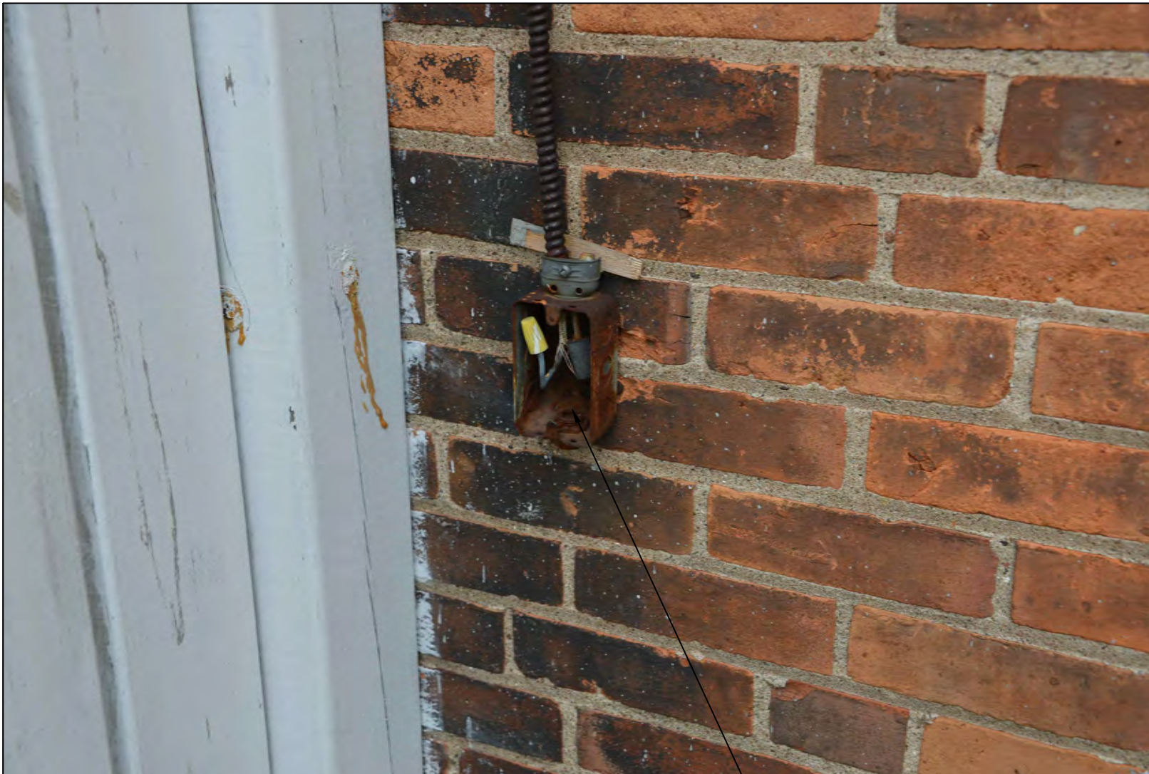
EXPOSED WIRING - CODE VIOLATION
