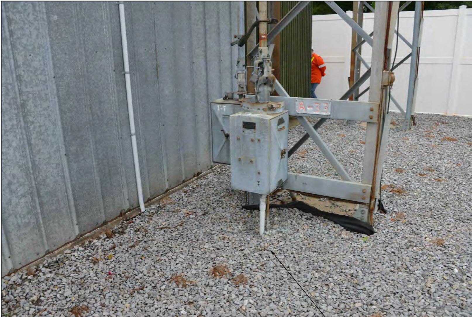
GRADIENT CONTROL MAT OR PORTABLE MAT REQUIRED FOR SWITCHING
